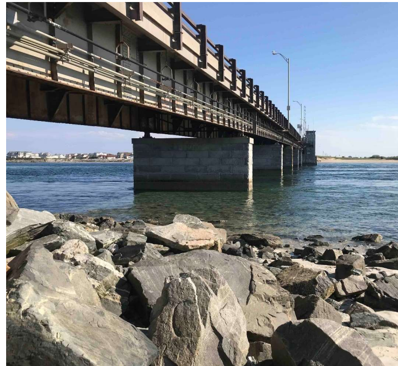
Bridge looking south
