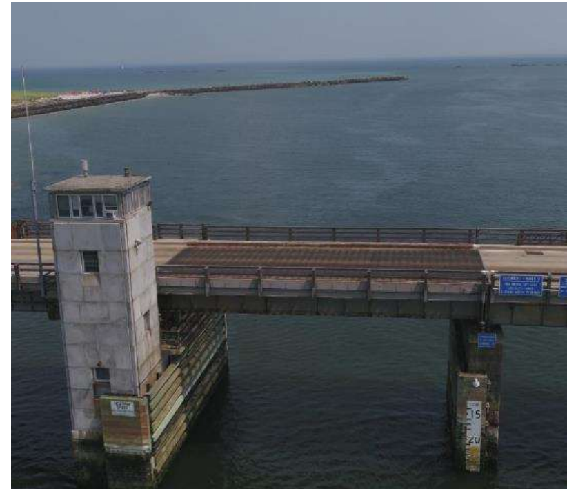
Bascule span, looking east
