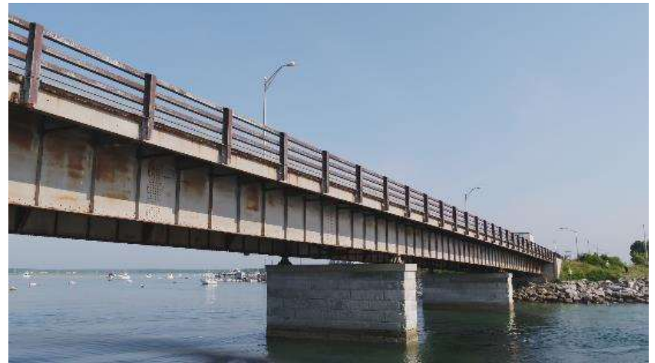
Seabrook-Hampton Bridge looking northwest
