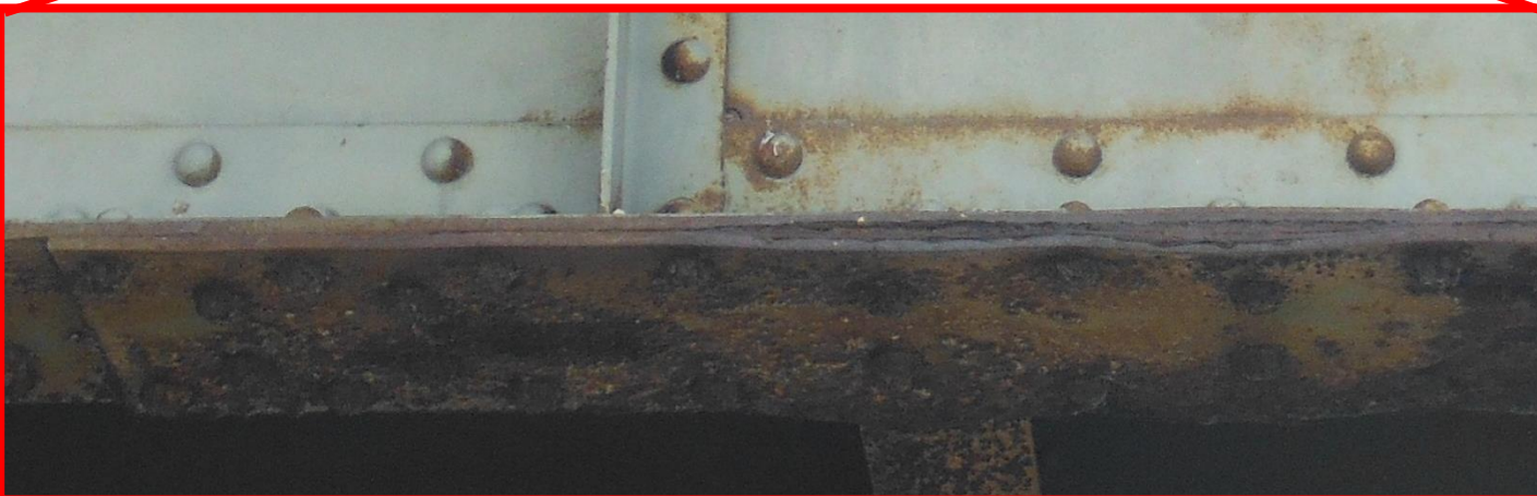
North Approach – Looking East
