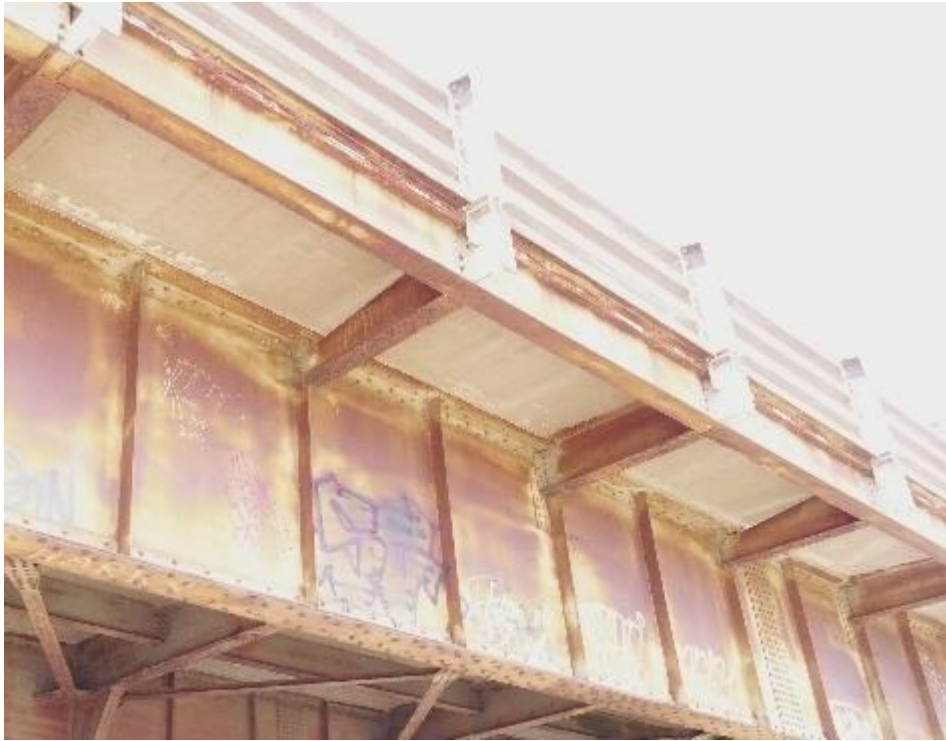
South Approach Looking West
