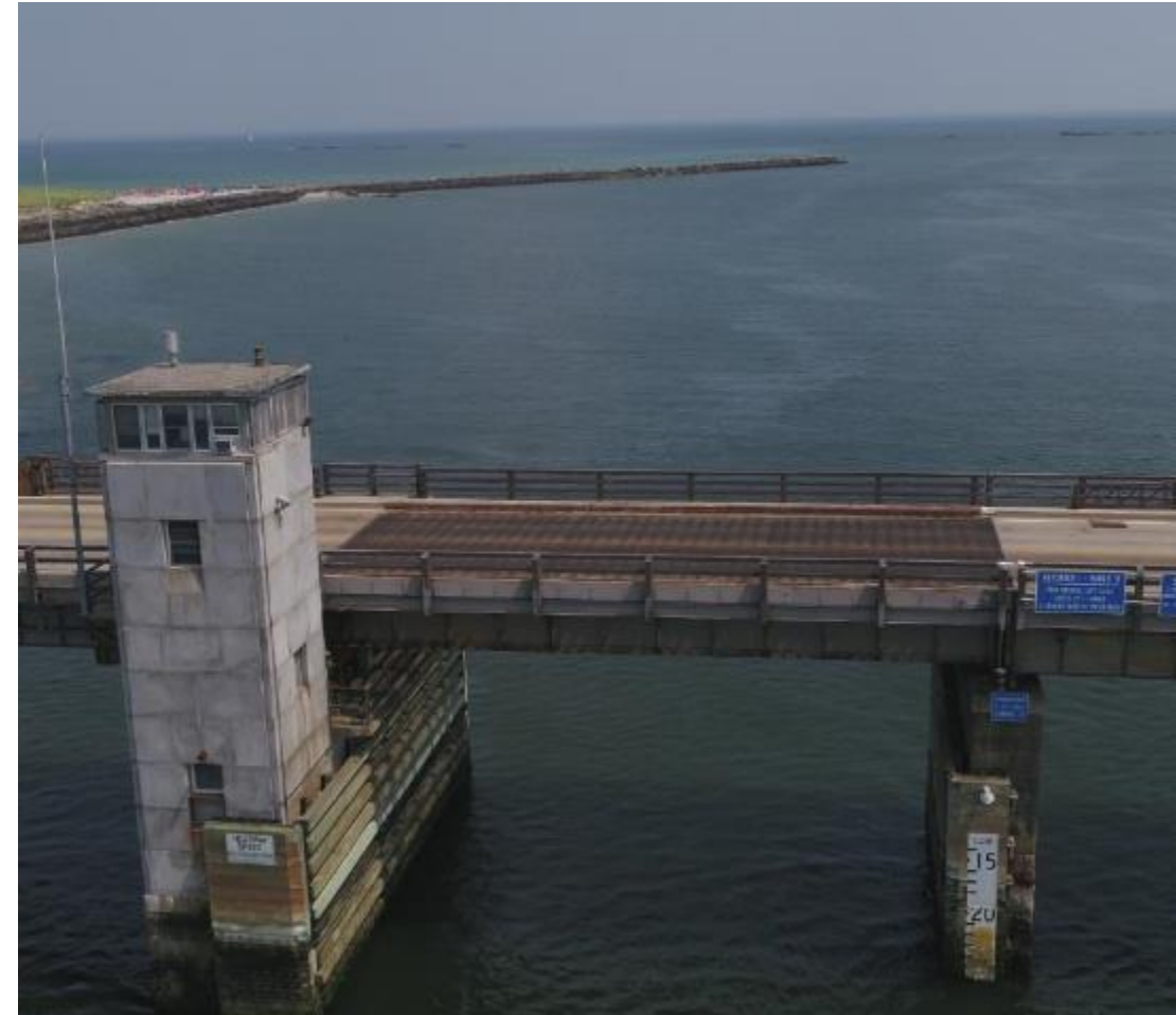
Bascule span, looking east
