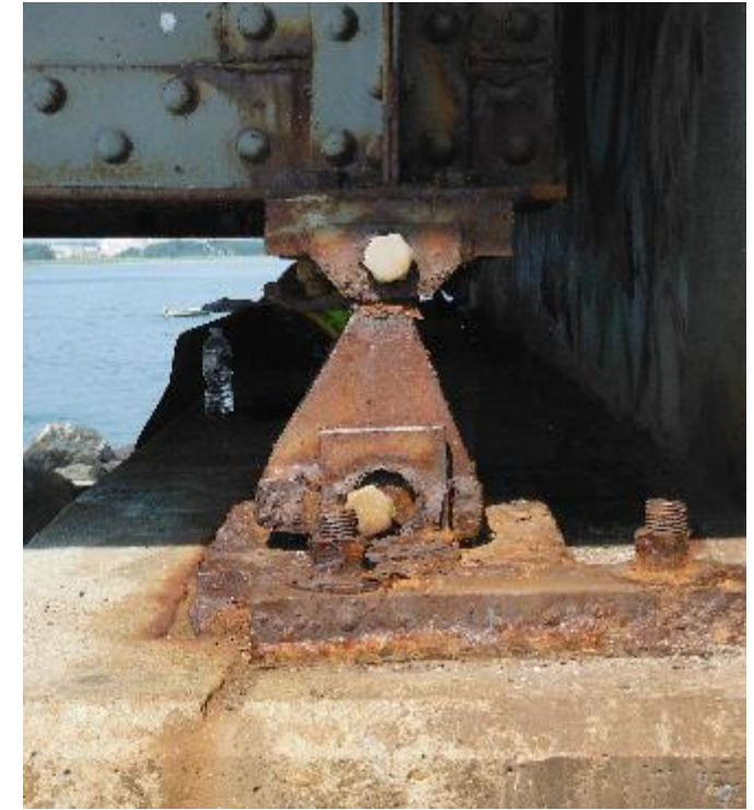
North Abutment Bearing
