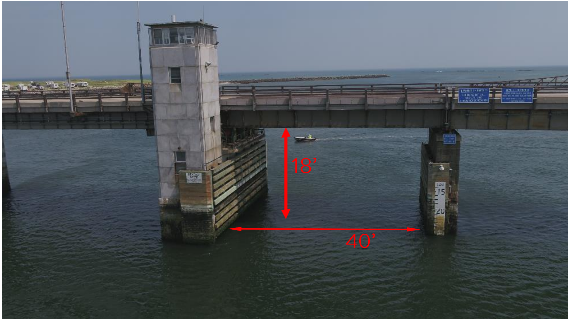
Stated Navigational Clearances per Coast Surveys at MHW
