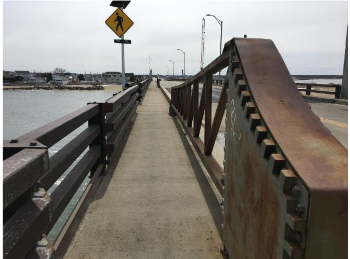
Existing sidewalk at barrier gate
