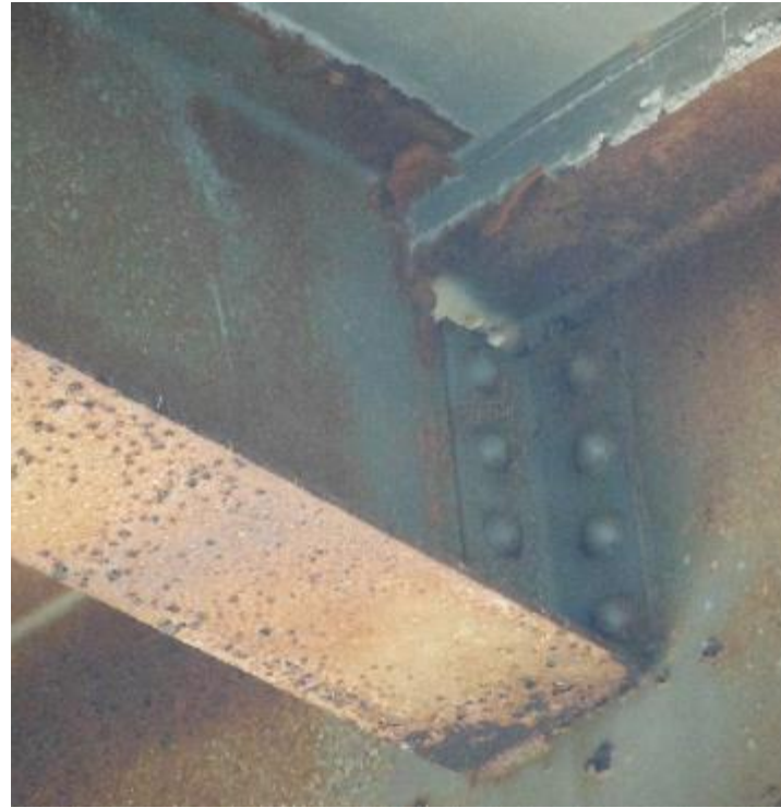
Typical Floorbeam/Girder Connection
