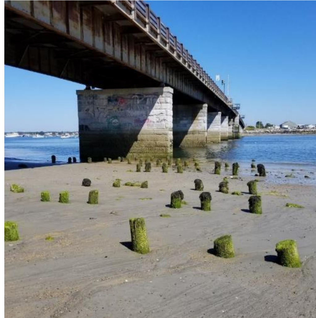
Near South abutment
