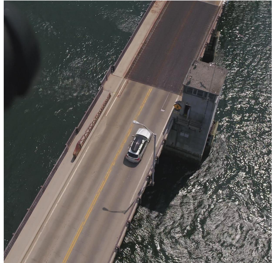
Looking downward at bascule span
