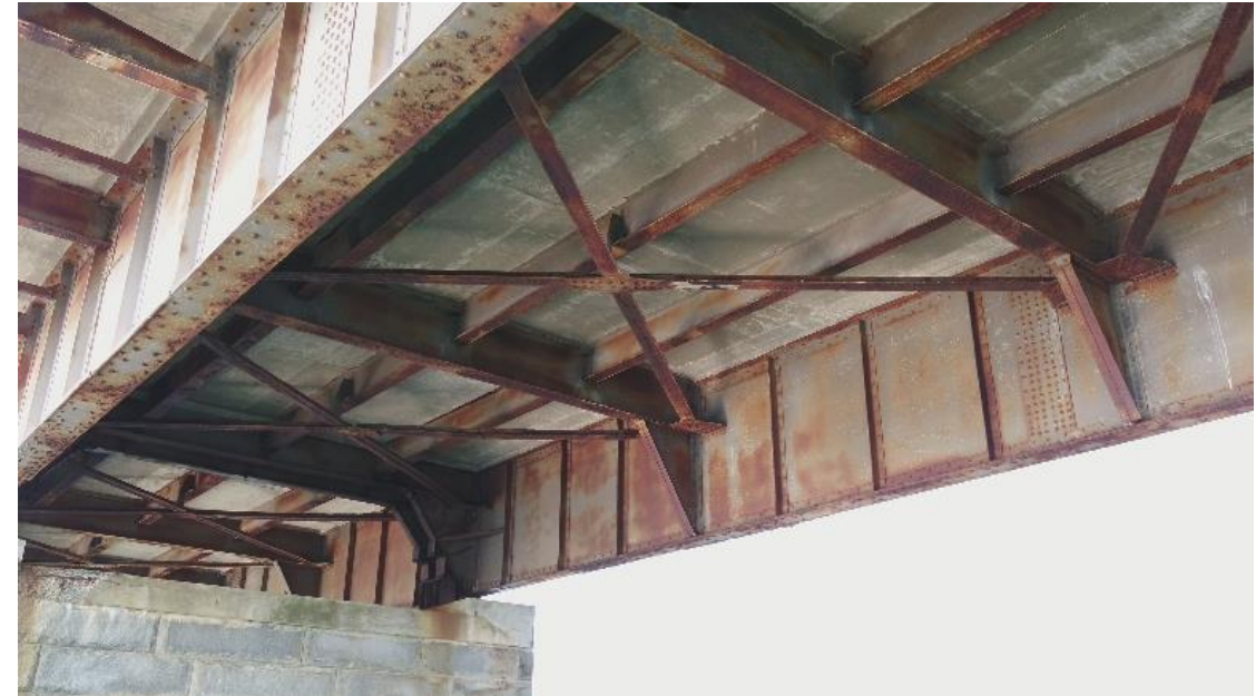
Typical Bridge Underside
