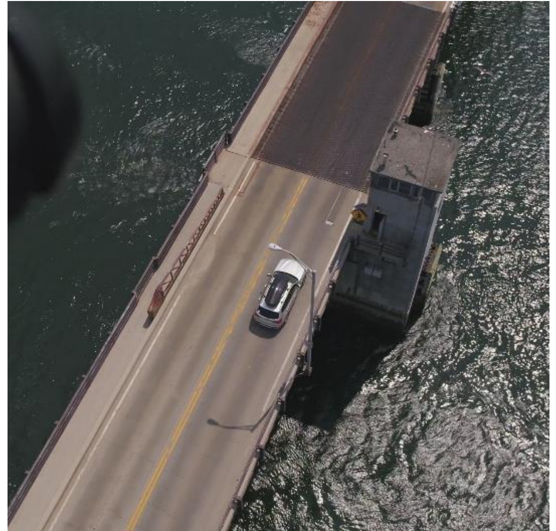
Looking down at bascule span
