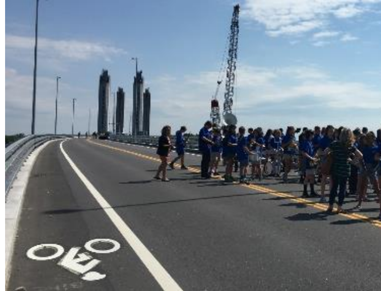
Sarah Mildred Long Bridge 4% Grade ~1,600 Linear Feet
