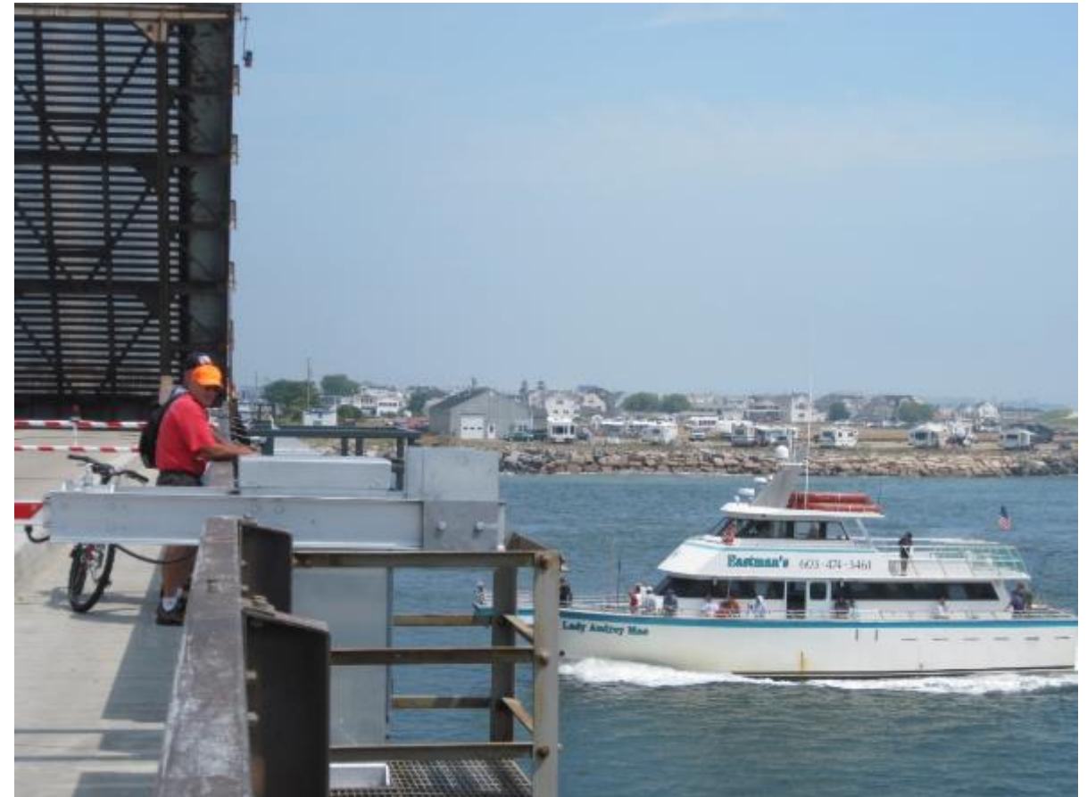
Bridge open to allow for vessel passage
