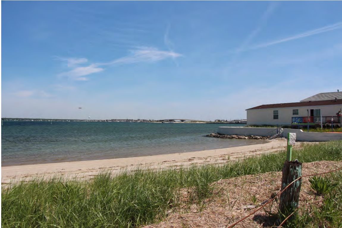
Figure 20: Simulation of the Fixed Bridge – west end of River Street looking northeast
