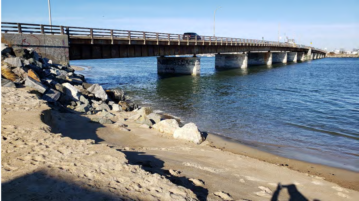
Figure 7: Existing view looking northwest from Sun Valley Beach
