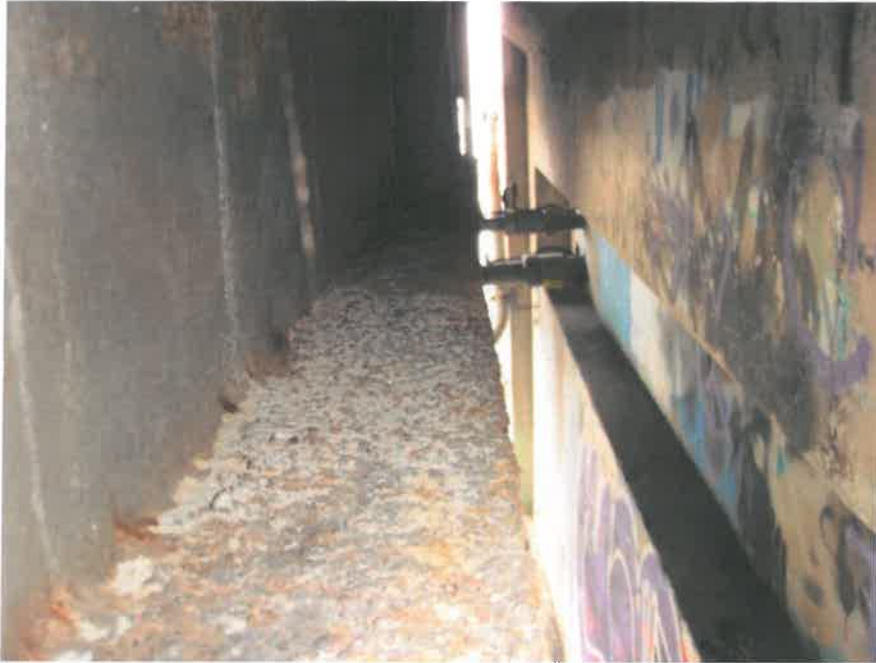
Photograph 9 – Upper Surface of Floorbeam Flange Depicted in Photograph 8
