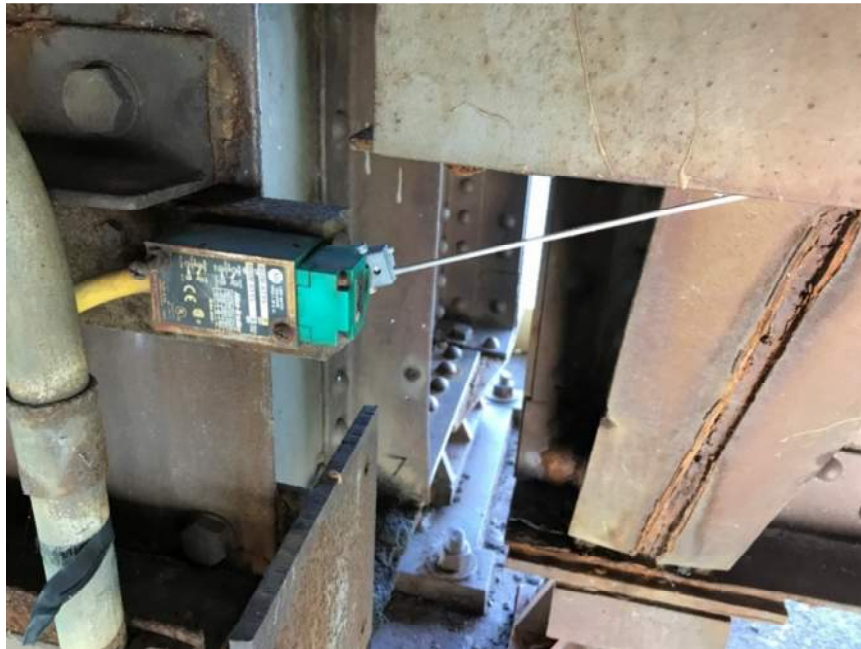
Photo E-11: Newer Span Seated Limit Switch
