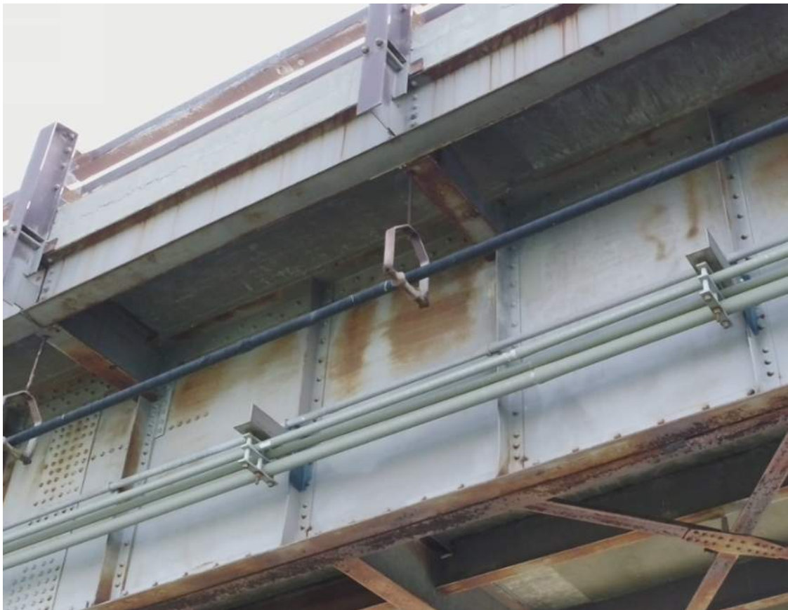
Photo S-10: General utility condition.
