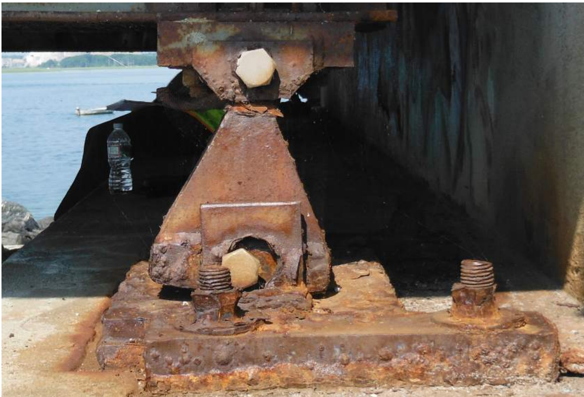
Photo S-16: Typical condition of bearings at abutments.
