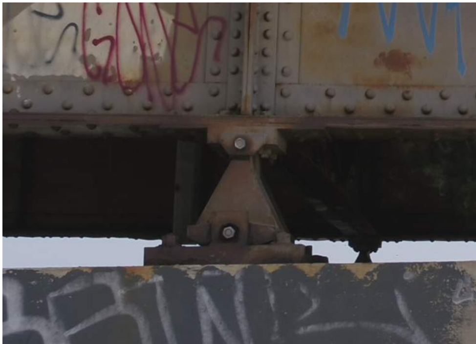
Photo S-15: Typical bearing conditions over piers without expansion joints.
