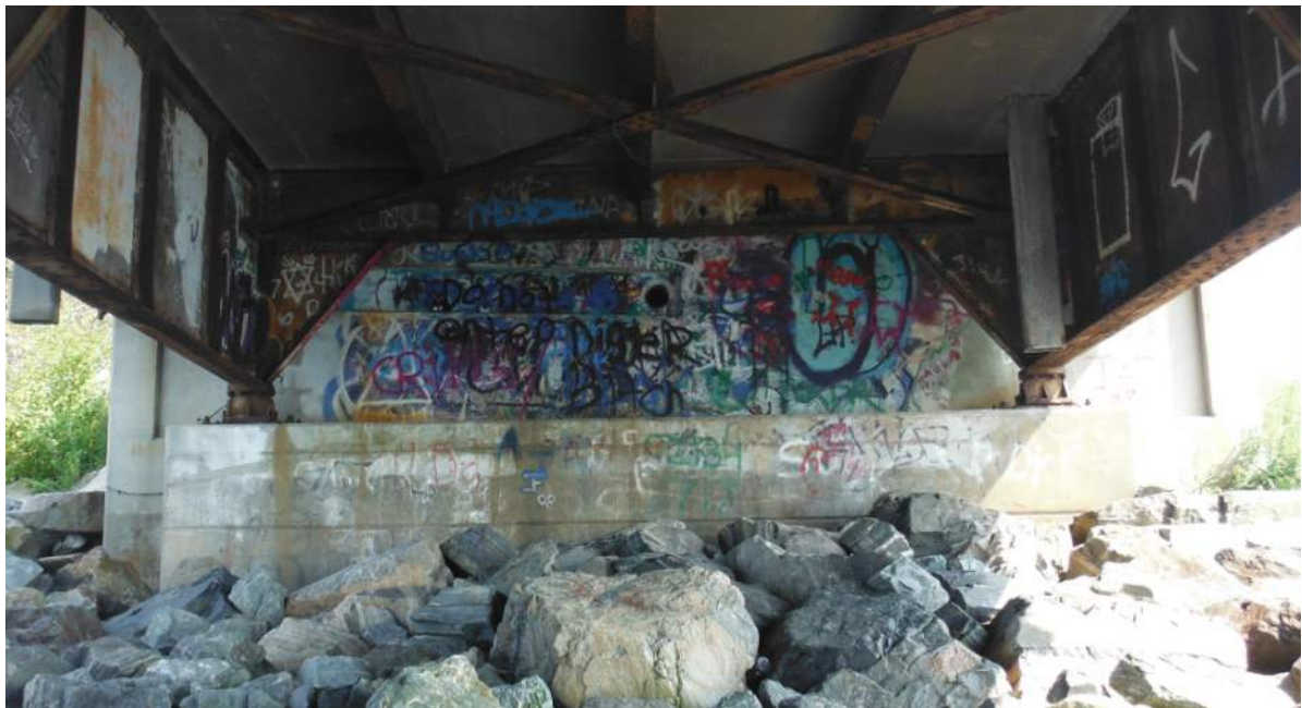
Photo S-18: North Abutment elevation.
