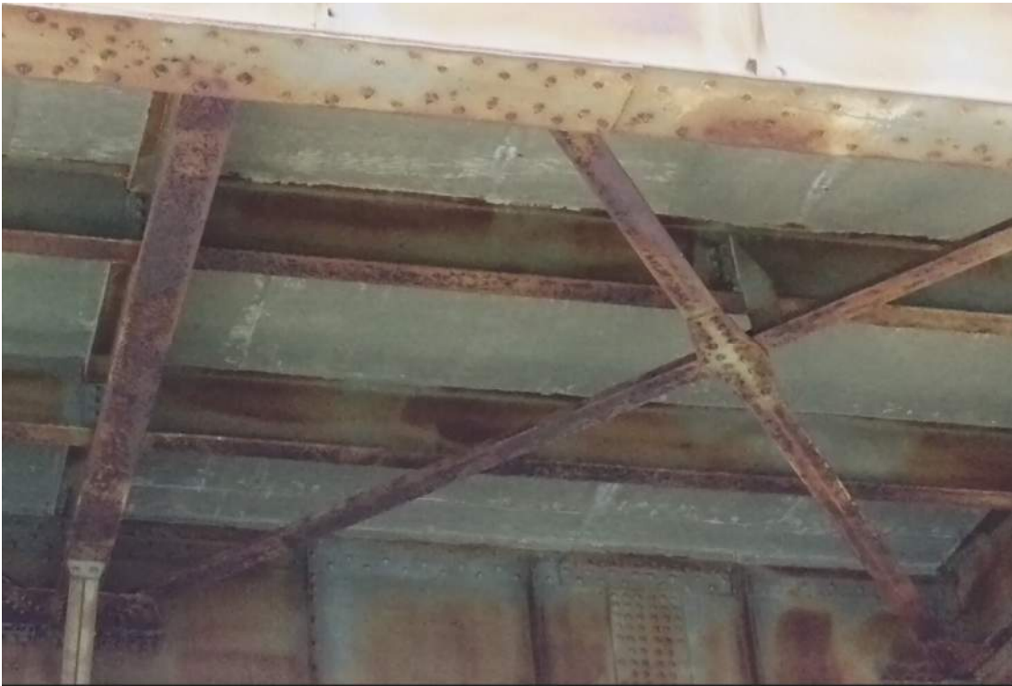
Photo S-11: Approach span stringer typical condition.
