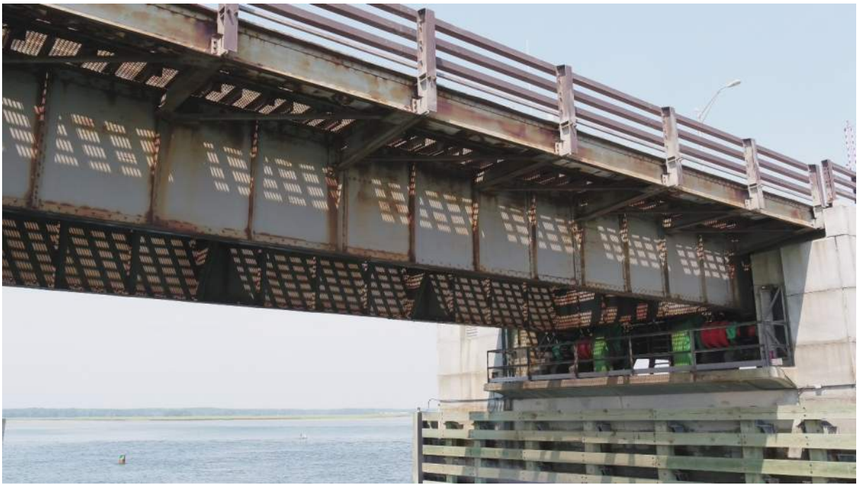
Photo S-07: Bascule span typical girder condition.
