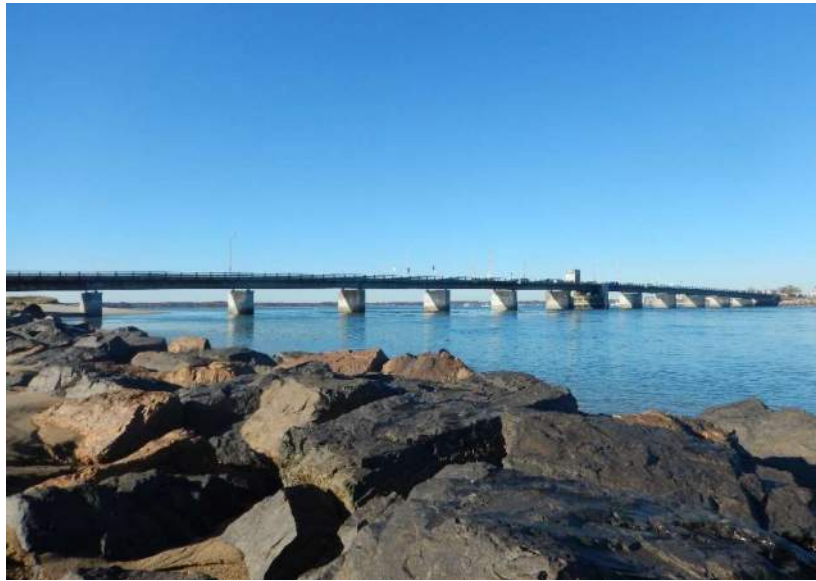
Figure 1. Existing Bridge, looking northwest from south bank.
