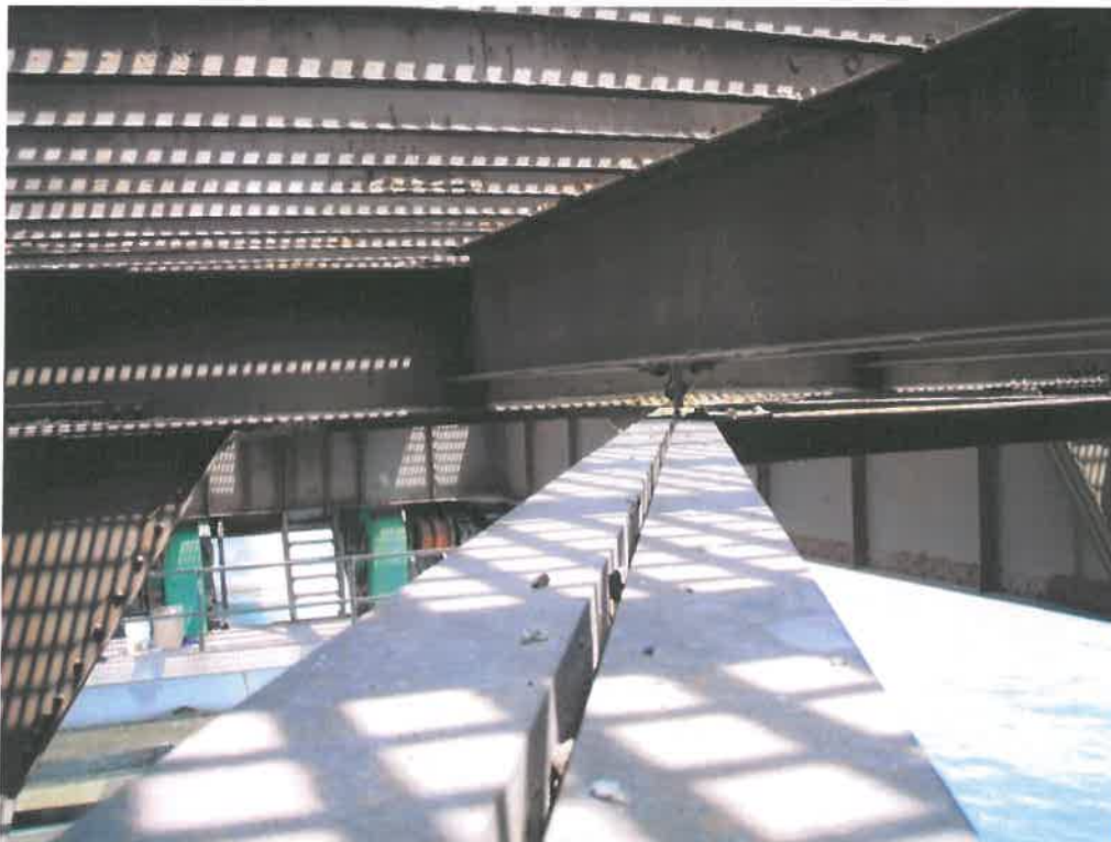
Photograph 21 – Condition of Lateral Bracing and Stringers in Lift Span
