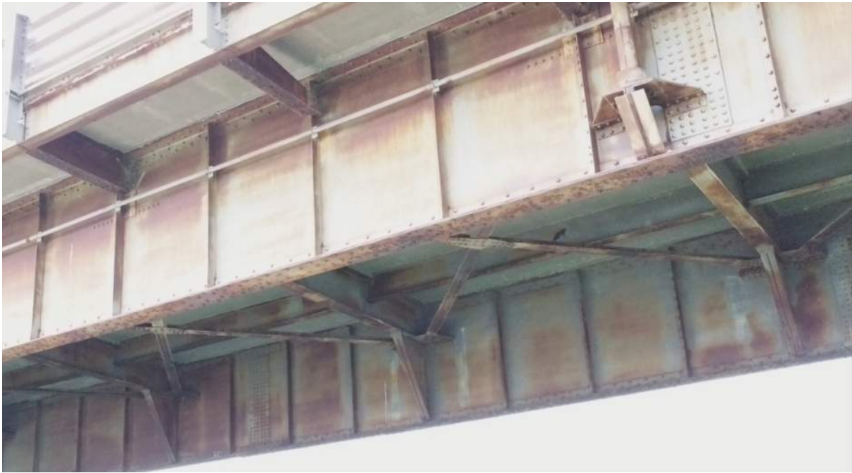
Photo S-05: Approach span typical condition.
