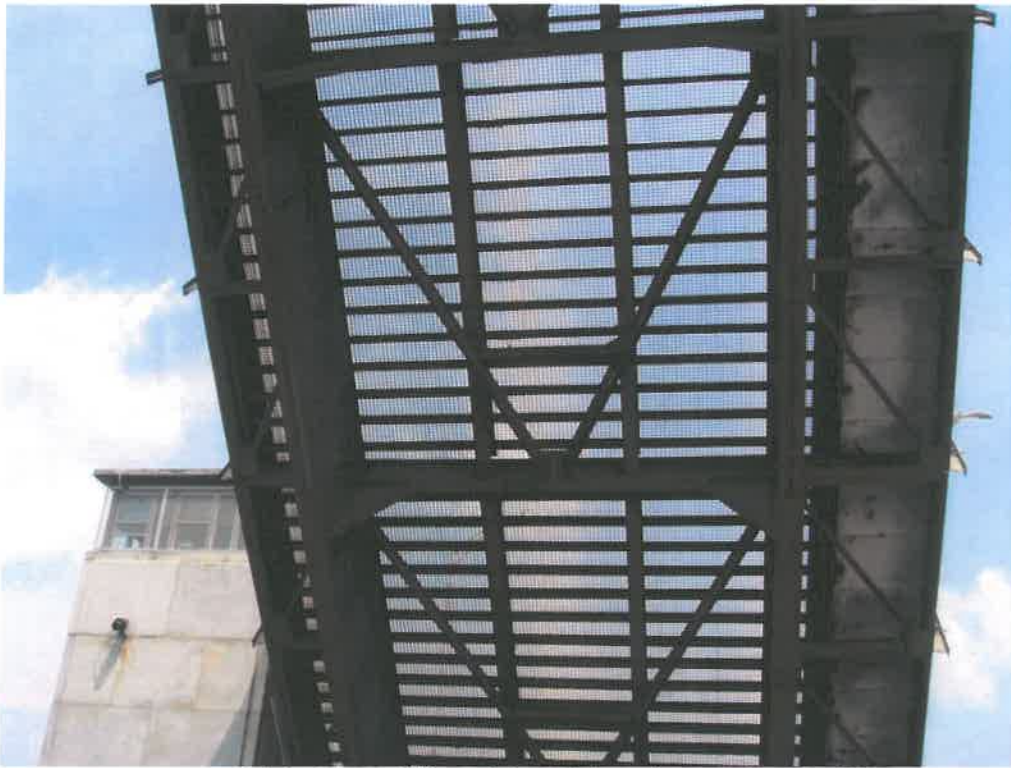
Photograph 16 – General View of the Lift Span in the Raised Position
