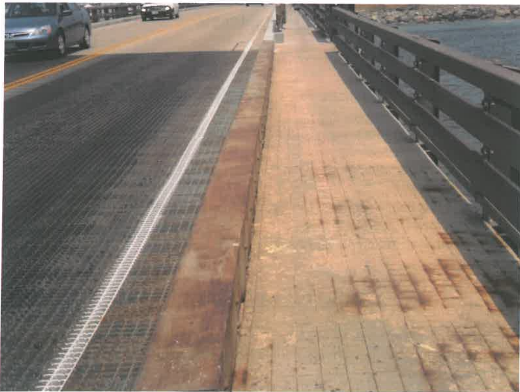
Photograph 27 -- Typical Condition of Steel Curbs in Lift Span
