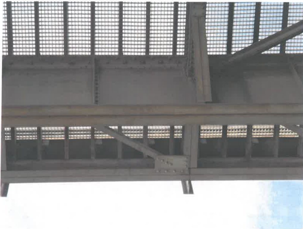
Photograph 18 – Somewhat Better Condition of Lift Span Girder and Fascia Members
