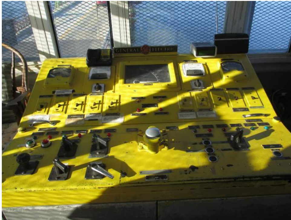
Photo E-09: Control Desk
