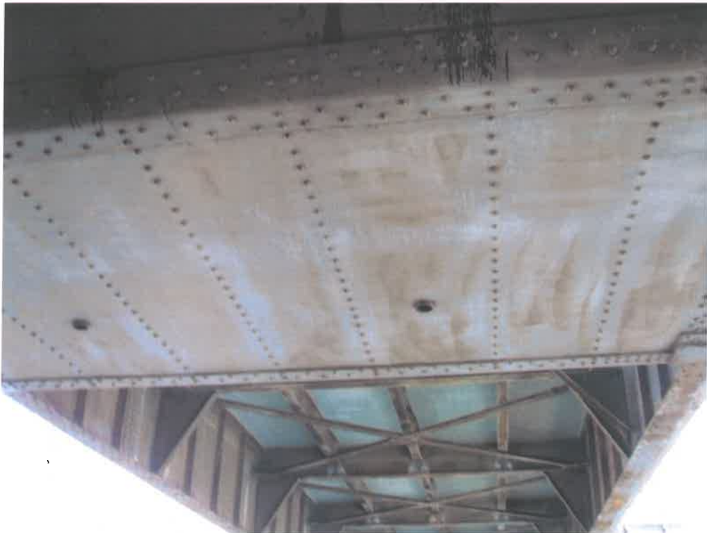
Photograph 25 – Typical Coating Condition of Counterweight
