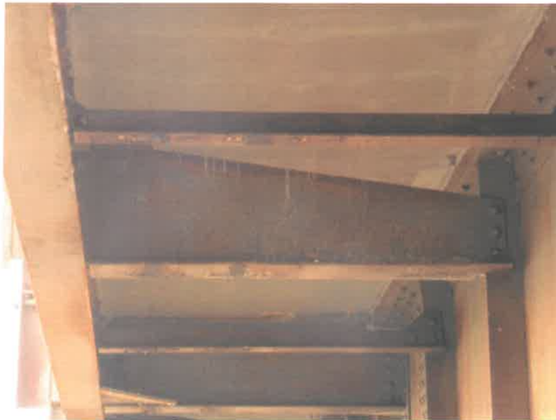
Photograph 14 -- Typical Condition of Sidewalk Support Members
