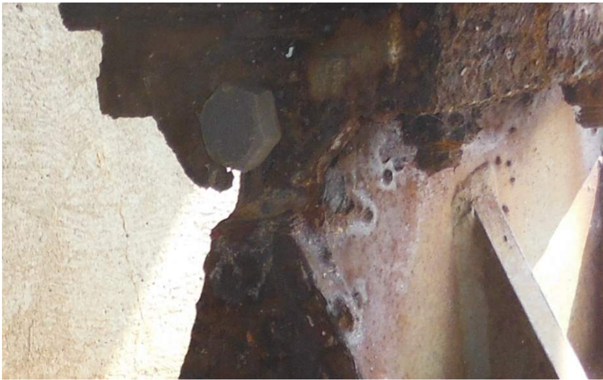
Photo S-17: Typical condition of bearings at abutments.
