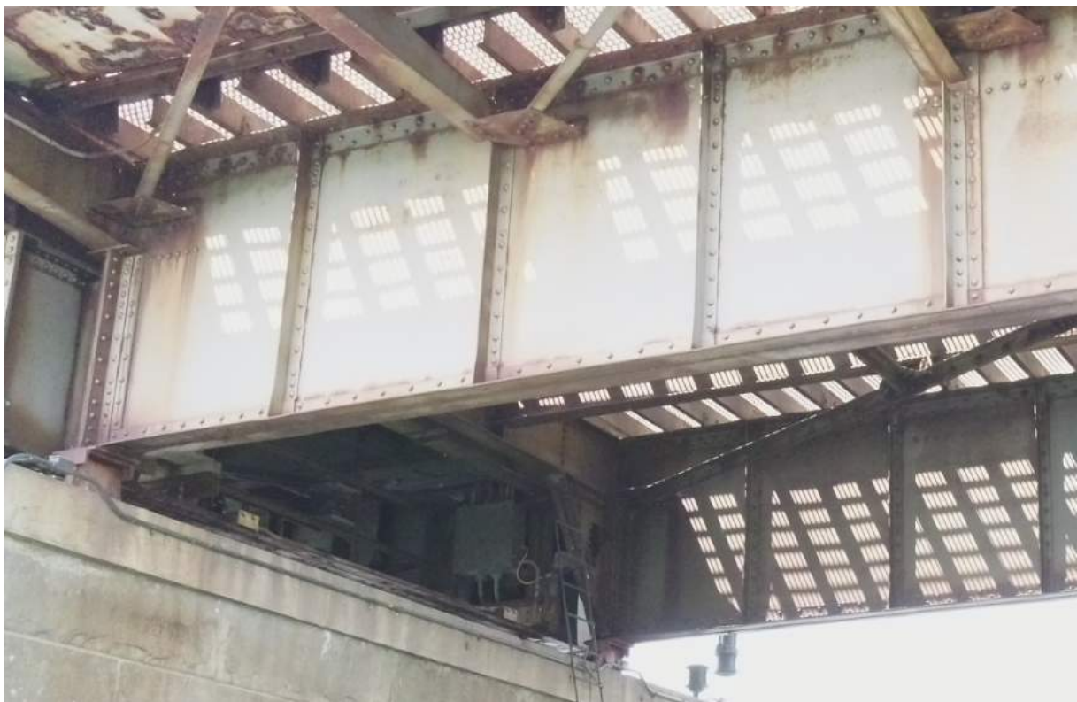
Photo S-04: Typical bascule girder condition.
