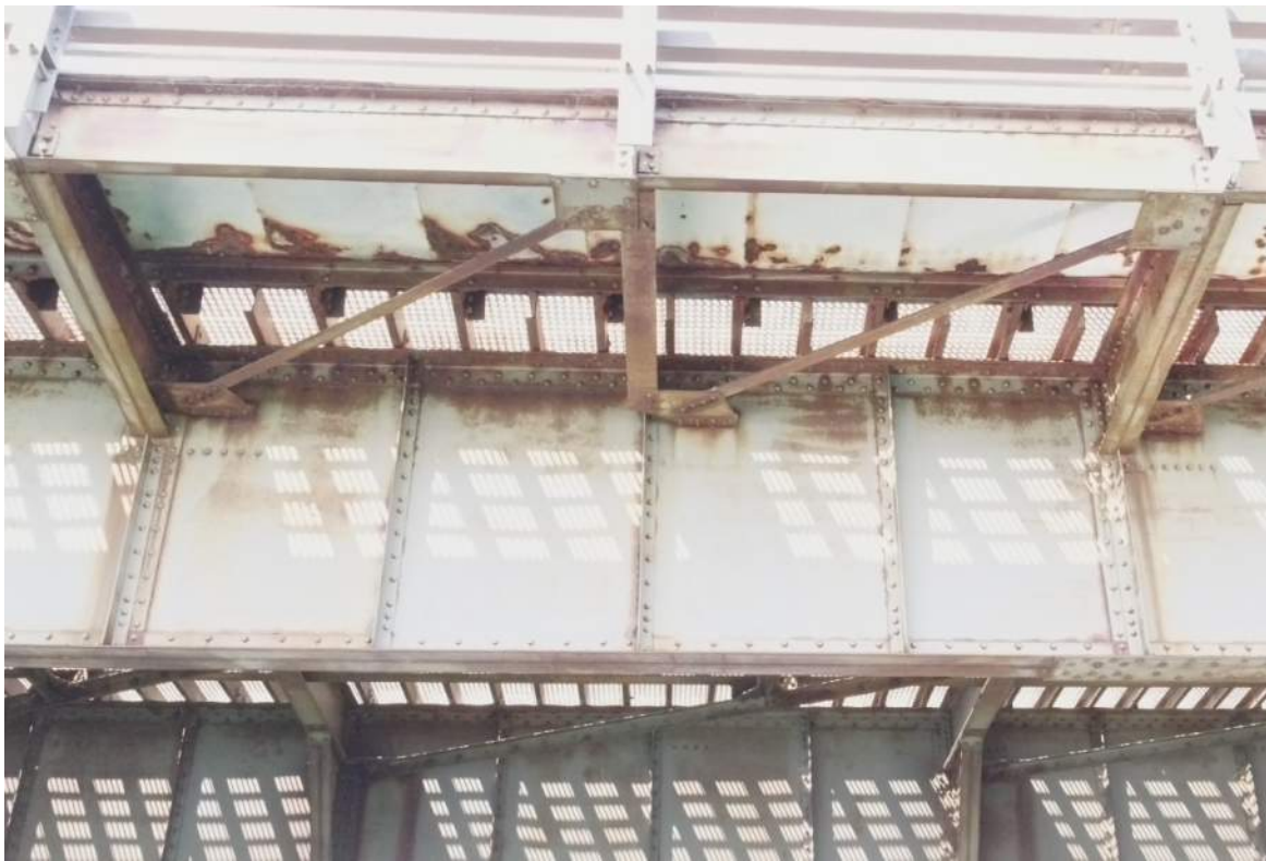
Photo S-03: Typical bascule span deck overhang condition.
