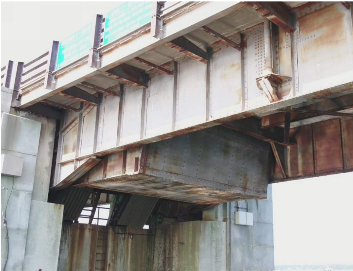
Photo S-06: Approach span at bascule span typical condition.
