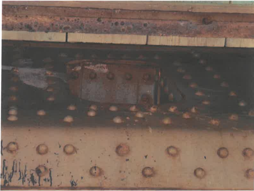
Photograph 24 – Typical Condition of Trunion Girder
