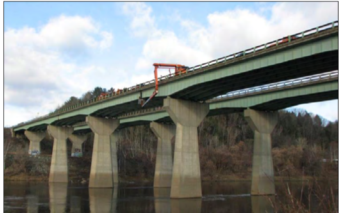
Figure BR1: Westerly Elevation View of Bridges
