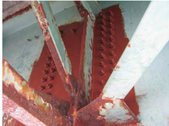
Figure BR10: Web Crack Bolted Plate Repair by NHDOT BBM (inside face)
