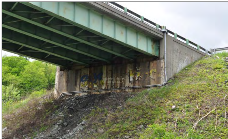
Figure BR14: North abutment on SB Bridge
