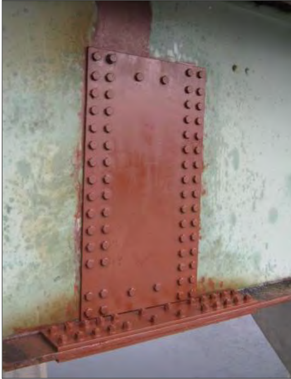
Figure BR9: Web Crack Bolted Plate Repair by NHDOT BBM (outside face)
