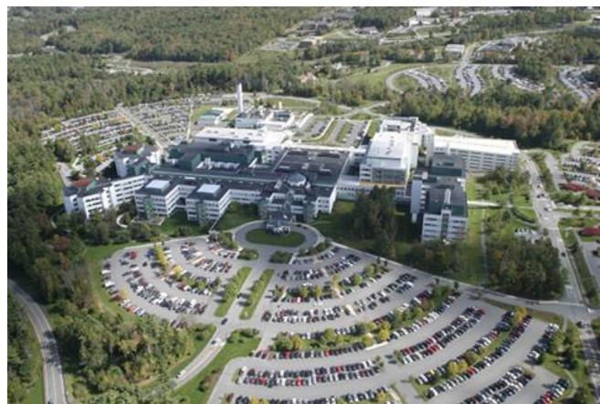
Major employers and healthcare providers such as Dartmouth-Hitchcock Medical Center rely on the I-89 Bridges Over the Connecticut River
