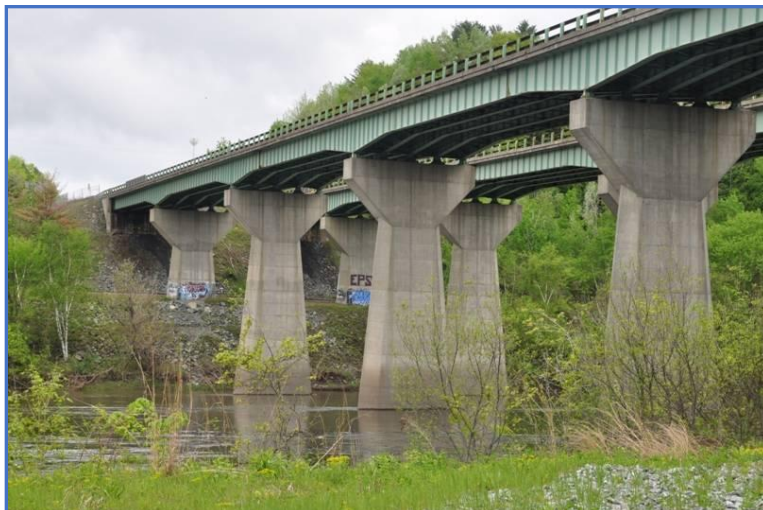
Vietnam Veterans Memorial Bridges Interstate 89 Lebanon, NH – Hartford, VT
