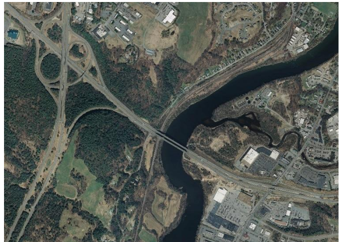
The I-89 Bridges are the key component in the transportation system of the Upper Valley
