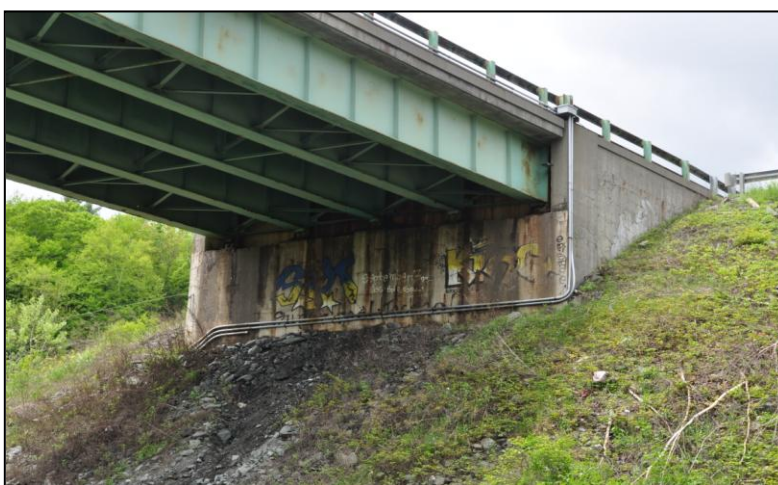
Figure BR14: North abutment on SB Bridge
