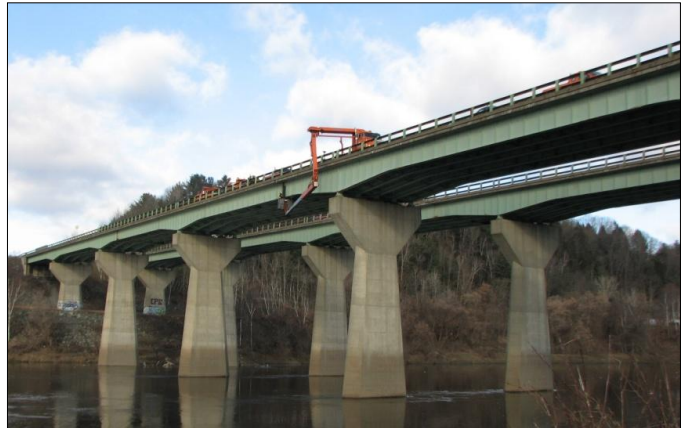
Figure BR1: Westerly Elevation View of Bridges
