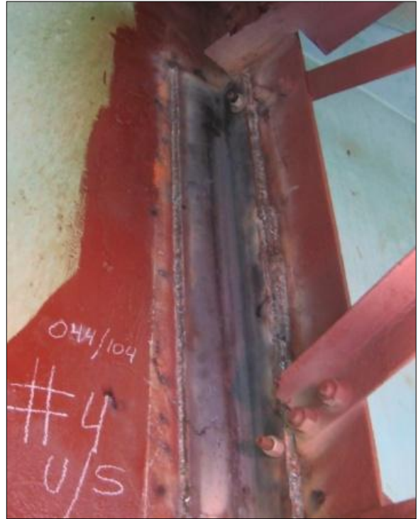
Figure BR13: Welded Angle Web Repair by NHDOT BBM
