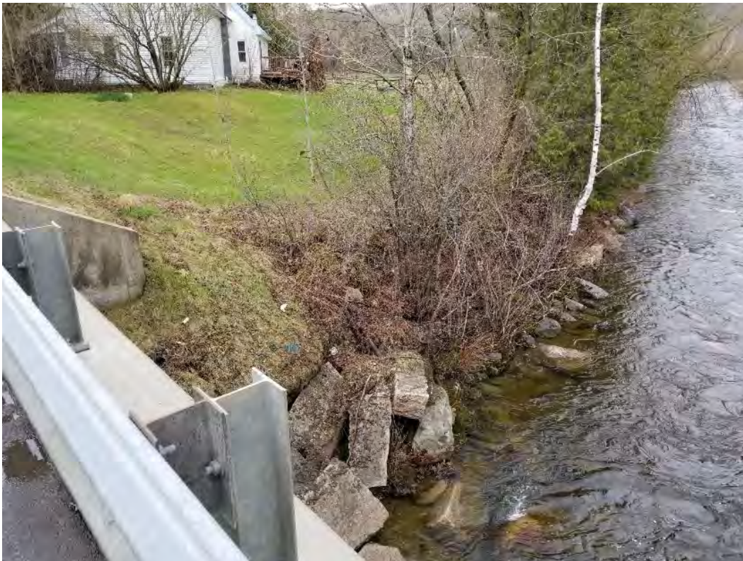
Photo 102. View of left-bank descending just below bridge from bridge
