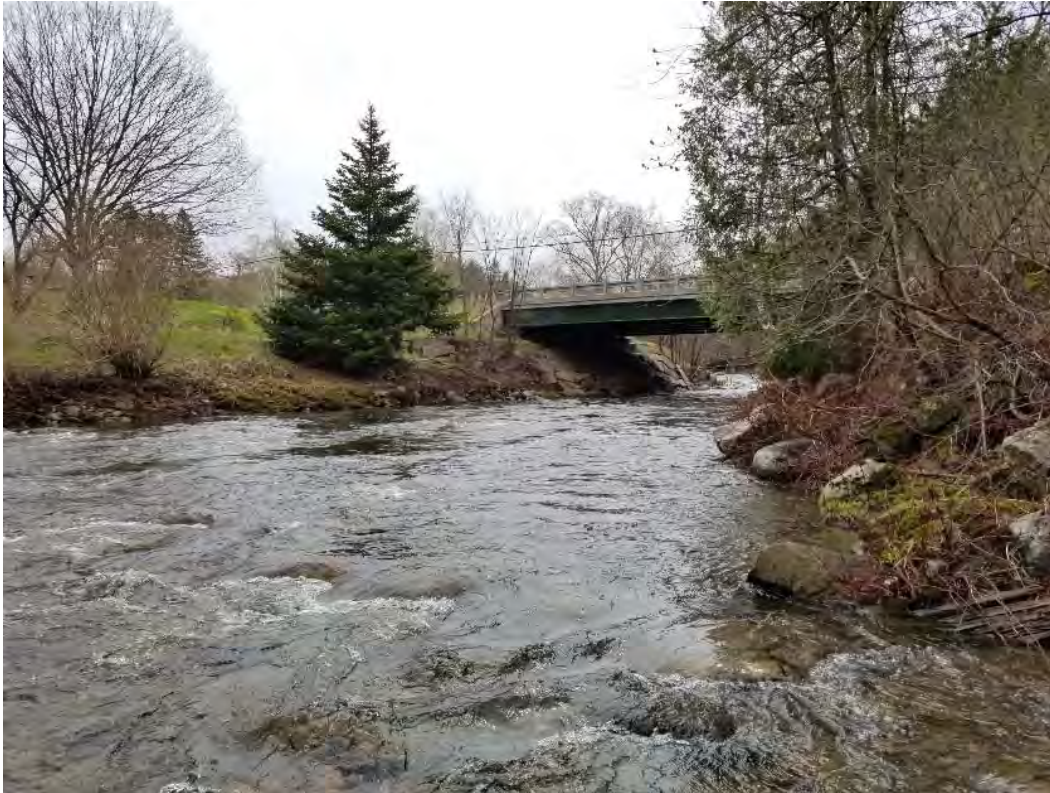
Photo 91. View upstream towards right-bank descending below bridge
