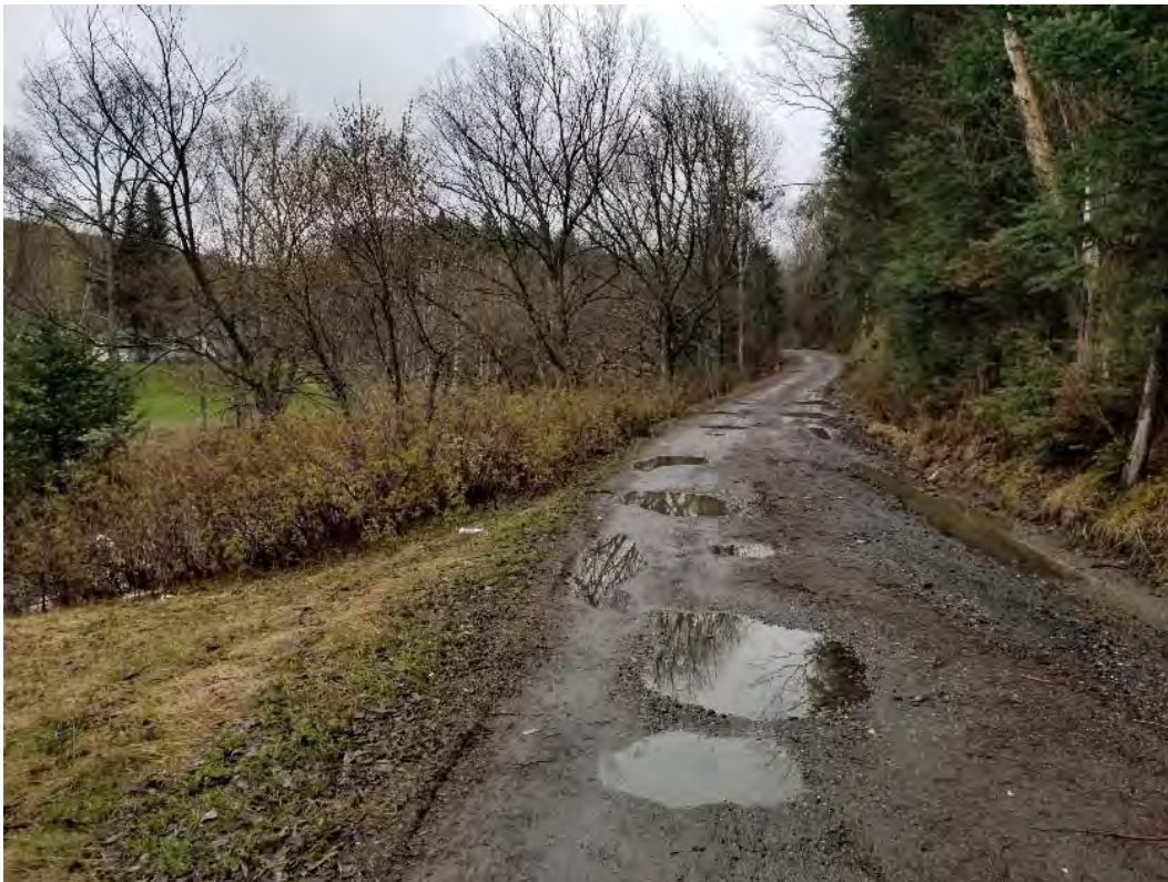
Photo 14. View of private driveway south of bridge
