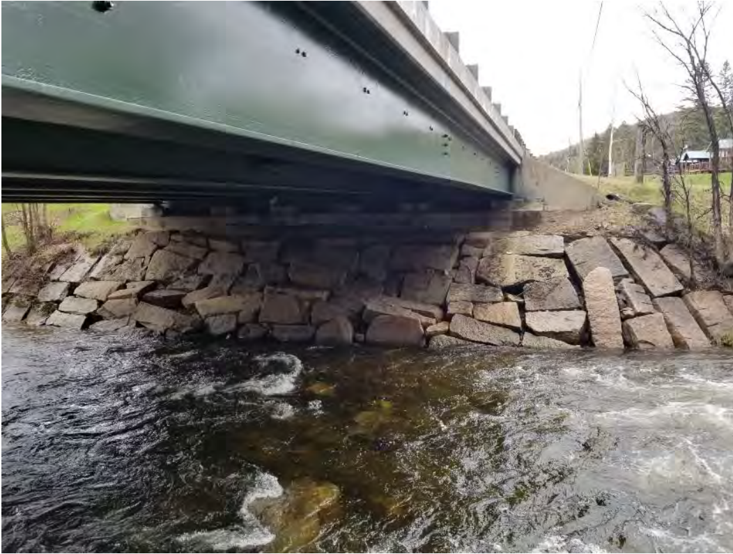
Photo 3. View of NE abutment from upstream side
