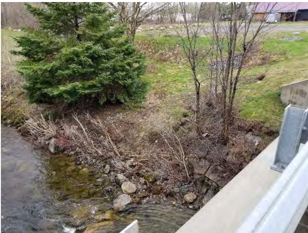
Photo 16. View of NE corner of bridge
