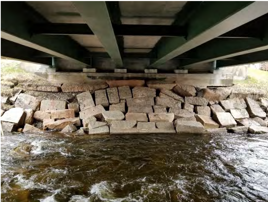
Photo 6. View of SW abutment from under bridge
