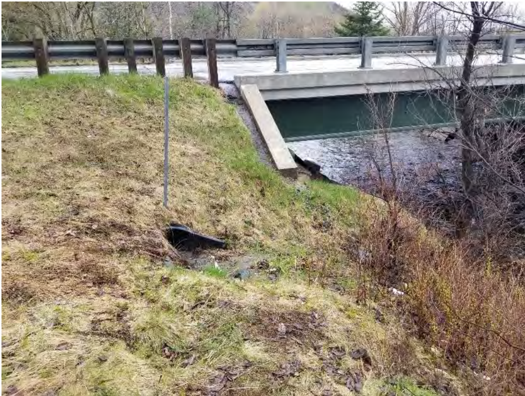
Photo 13. View of SW corner of bridge
