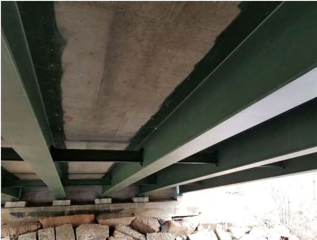
Photo 17. Underside of bridge
