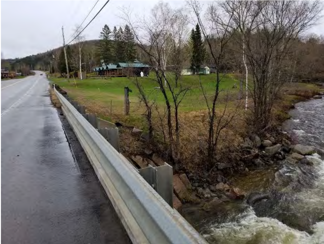
Photo 15. View of SE corner of bridge
