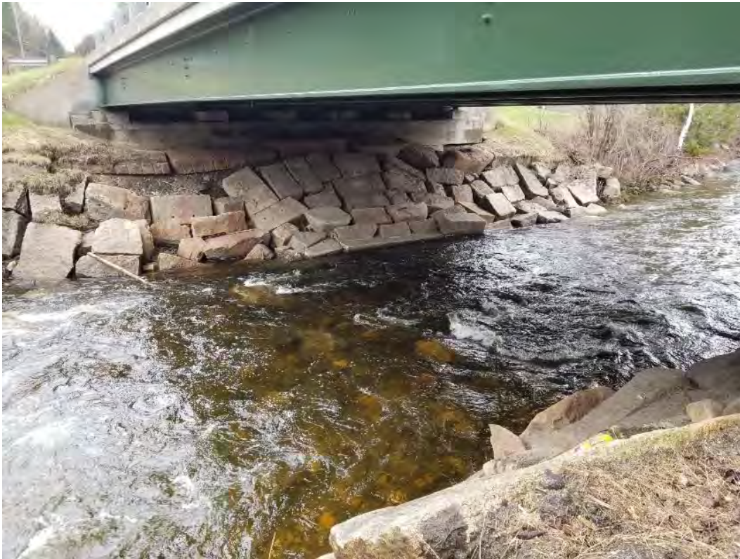
Photo 5. View of SW abutment from upstream side
