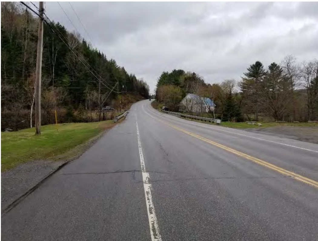
Photo 2. View SE along Route 3
