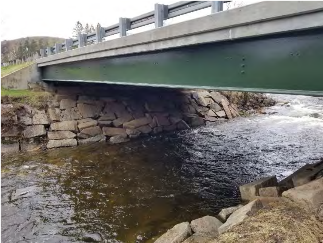
Photo 4. View of NE abutment from downstream side
