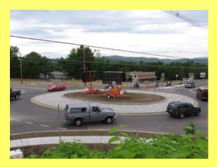
**U-Turns** – Roundabouts provide access to all approaches and also make U-Turns easy and convenient. All vehicles, including tractor trailers can make U-Turns at a roundabout.
