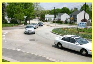
**Capacity** – Because of the free flow nature of a roundabout, the slower speeds and closer vehicles tend to travel through roundabouts, more vehicles can go through a roundabout. Studies show that a roundabout can process about 30% more traffic than other types of intersections.
