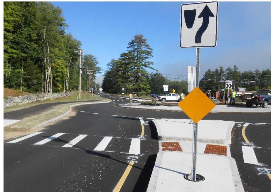
NH Route 32 South Approach
