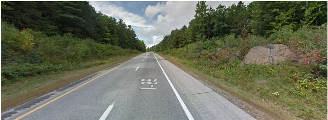
Impact Location AD (Left) and AE (Right): Looking towards north at approx. Sta. 1518 NB in Wetland # 179 for AD & # 180 for AE.
