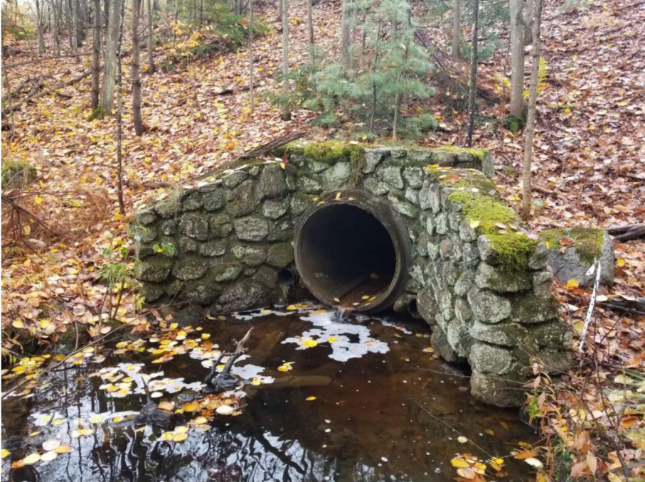
Impact Location S: Looking towards the outlet of the 36" RCP at approx. Sta. 1459 SB Median in Wetland # 138.
