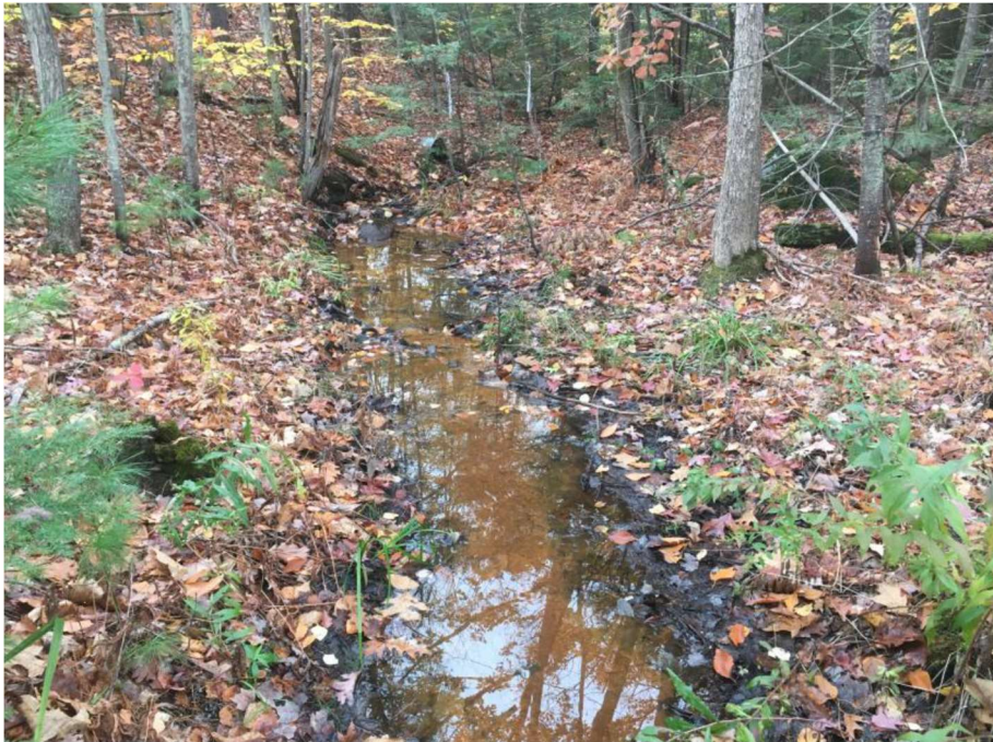
Impact Location AN: Looking towards the outlet of the 24" RCP at approx. Sta. 1542 SB Median in Wetland # 205.
