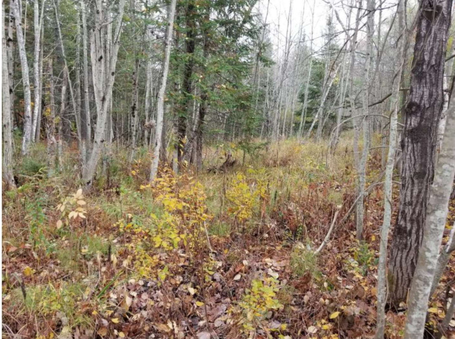
Impact Locations T, U and V: Looking away from the outlet of the 36" CMP at approx. Sta. 308 NB Off-Ramp at Exit 10 in Wetland #s 135, 138 and 140.
