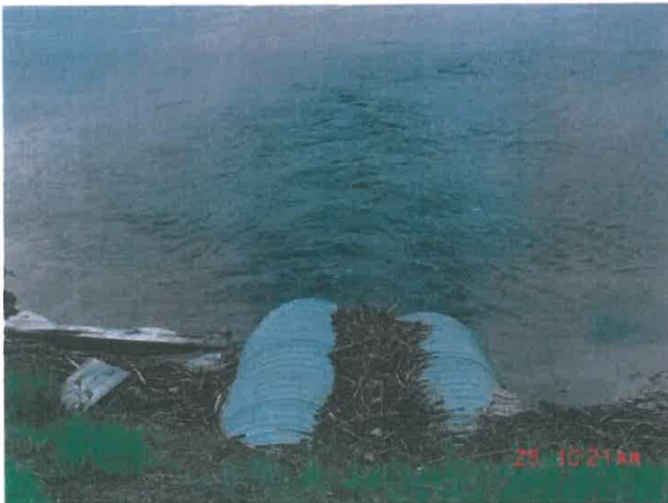
Outlet end (Looking west)
