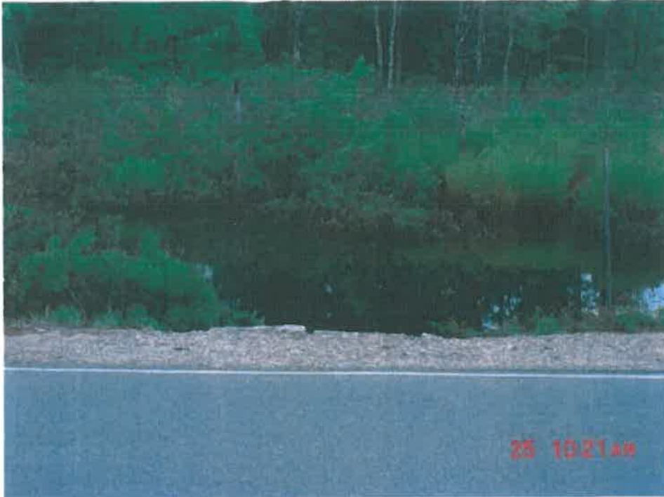
Inlet end (Looking east)
