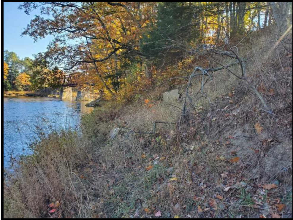
Photo 7 – Downstream of Bridge View Down West Bank Facing Downstream – 10/19/2022
