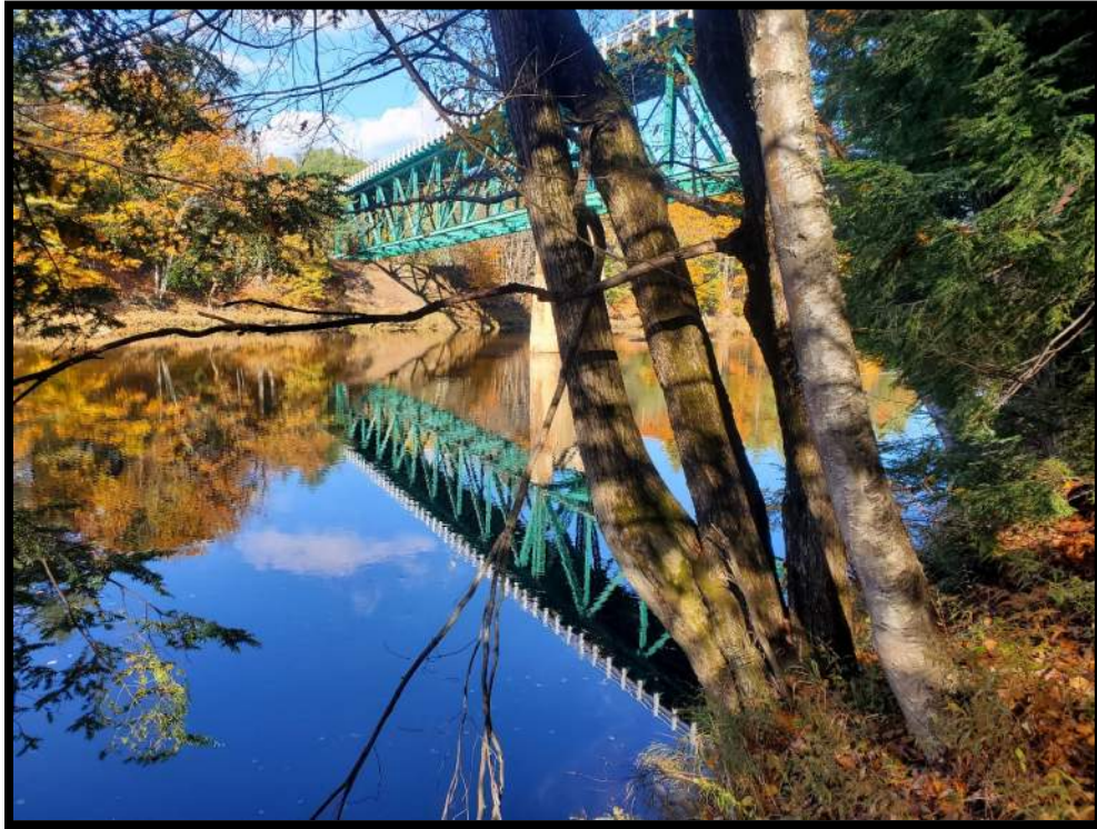
Photo 1 – Downstream of Bridge East Bank Facing Upstream – 10/19/2022
