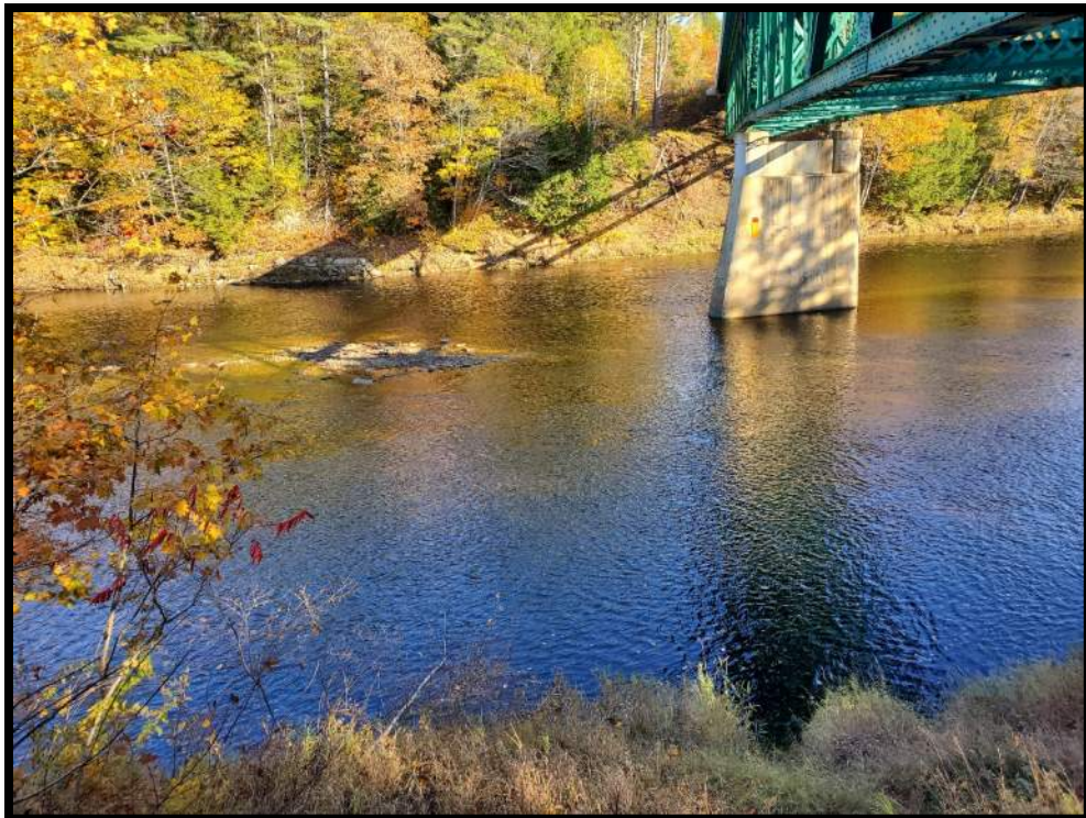
Photo 6 – Upstream of Bridge from West Bank Facing Across River – 10/19/2022
