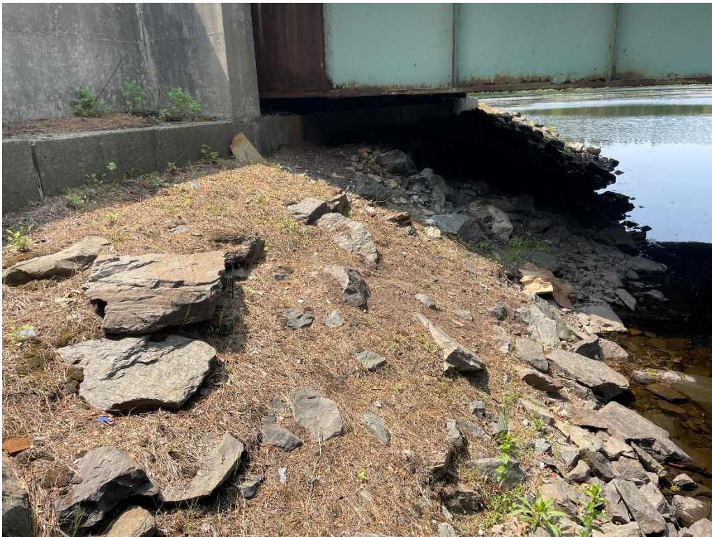
Photo 10: Pennichuck Brook Crossing Southern Abutment facing East (May 2023) IMPACT AREA: A
