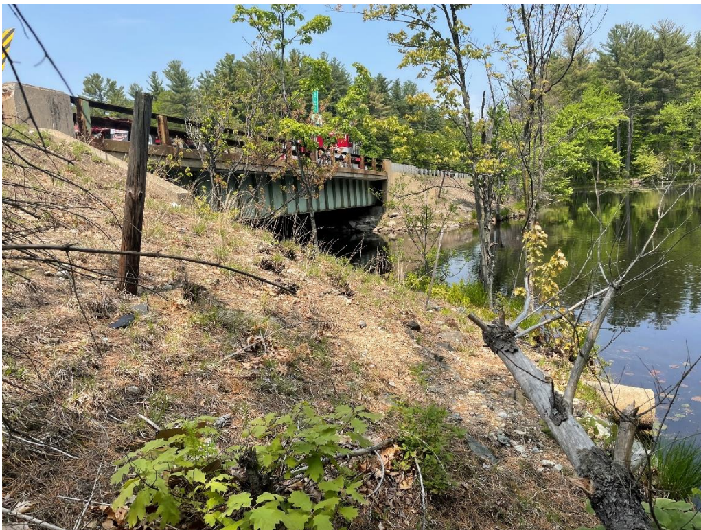
Photo 6: Pennichuck Brook Crossing SE Bridge Quadrant (May 2023) IMPACT AREA: A / B
