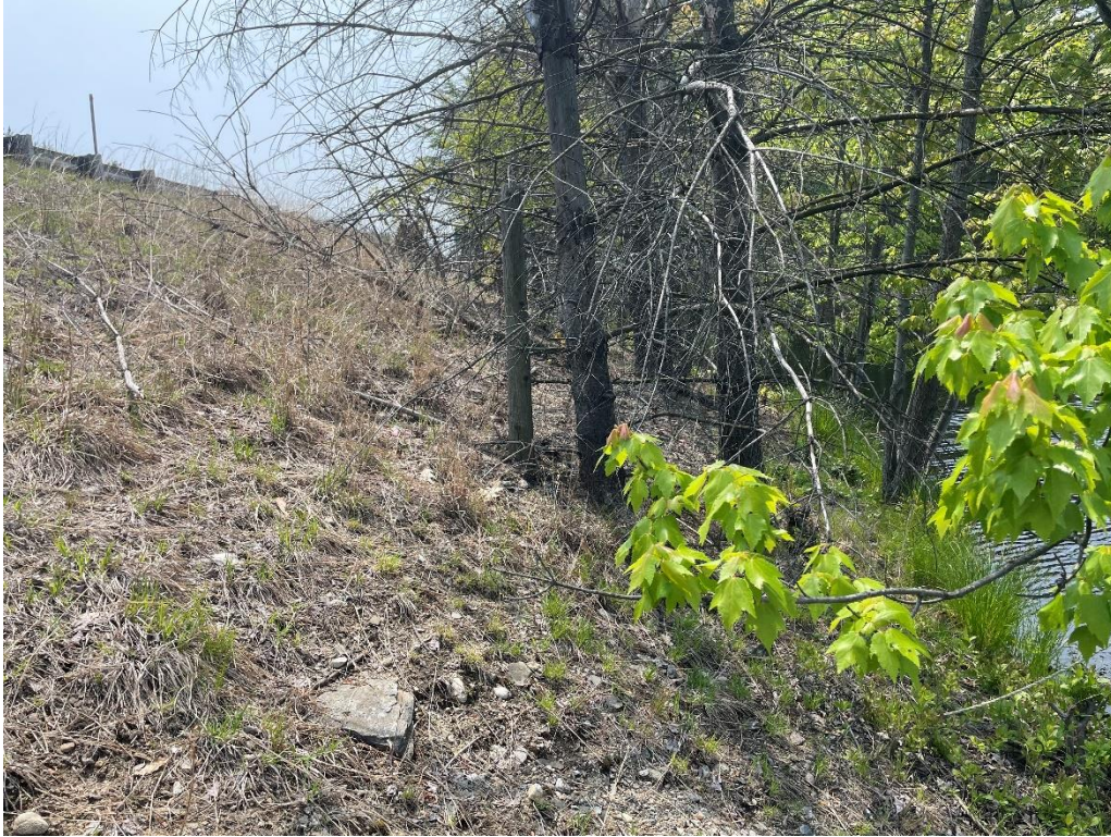
Photo 11: SW Bridge Quadrant Causeway Slope (May 2023) IMPACT AREA: A / TC
