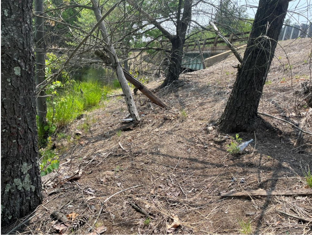
Photo 13: NE Bridge Quadrant Causeway Slope (May 2023) IMPACT AREA: D
