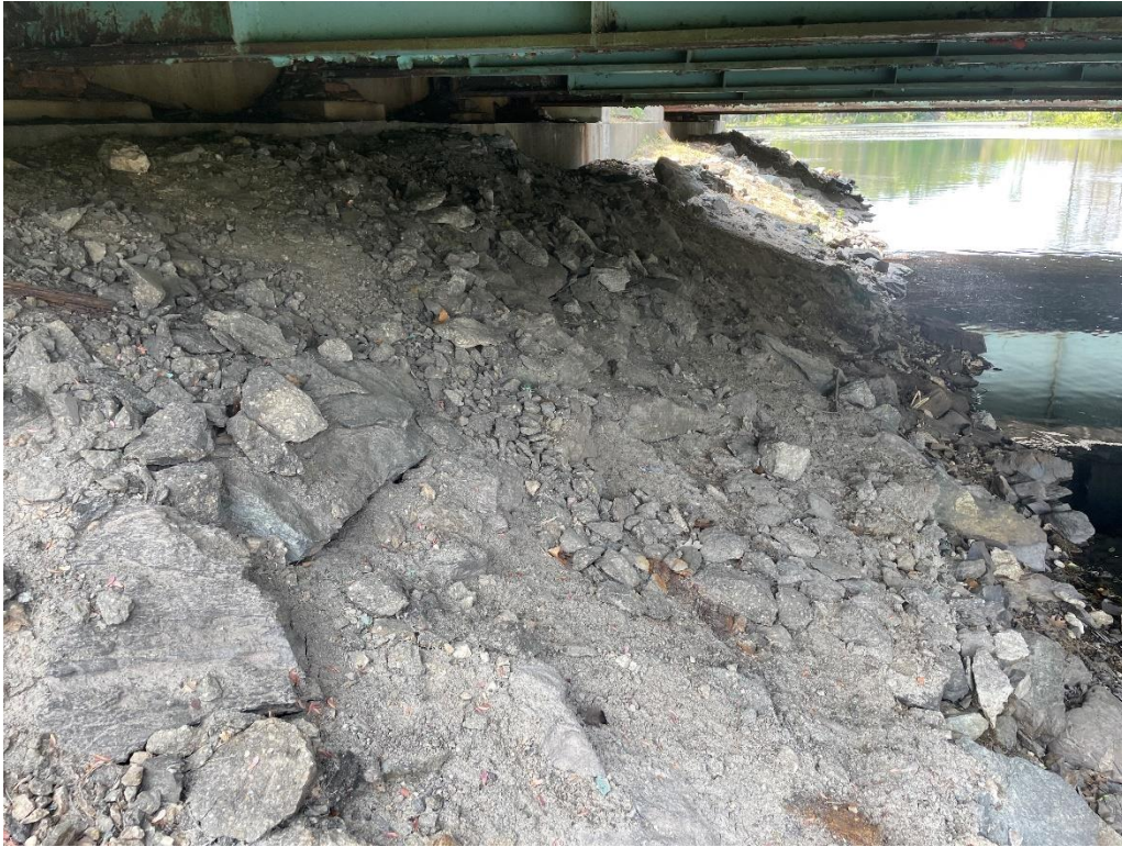
Photo 7: Pennichuck Brook Crossing Southern Abutment (May 2023) IMPACT AREA: A
