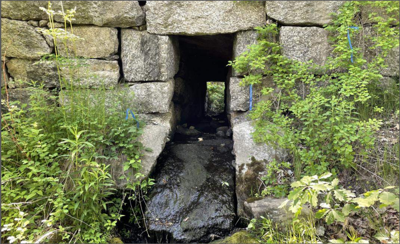
Photo 5: Looking Upstream at Crossing Outlet
