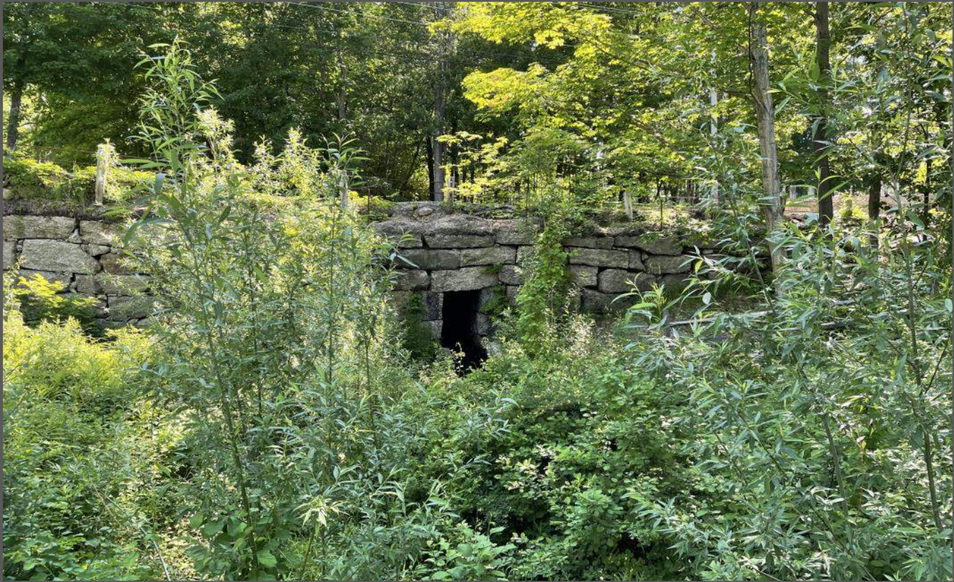
Photo 3: Looking Upstream at Crossing Outlet
