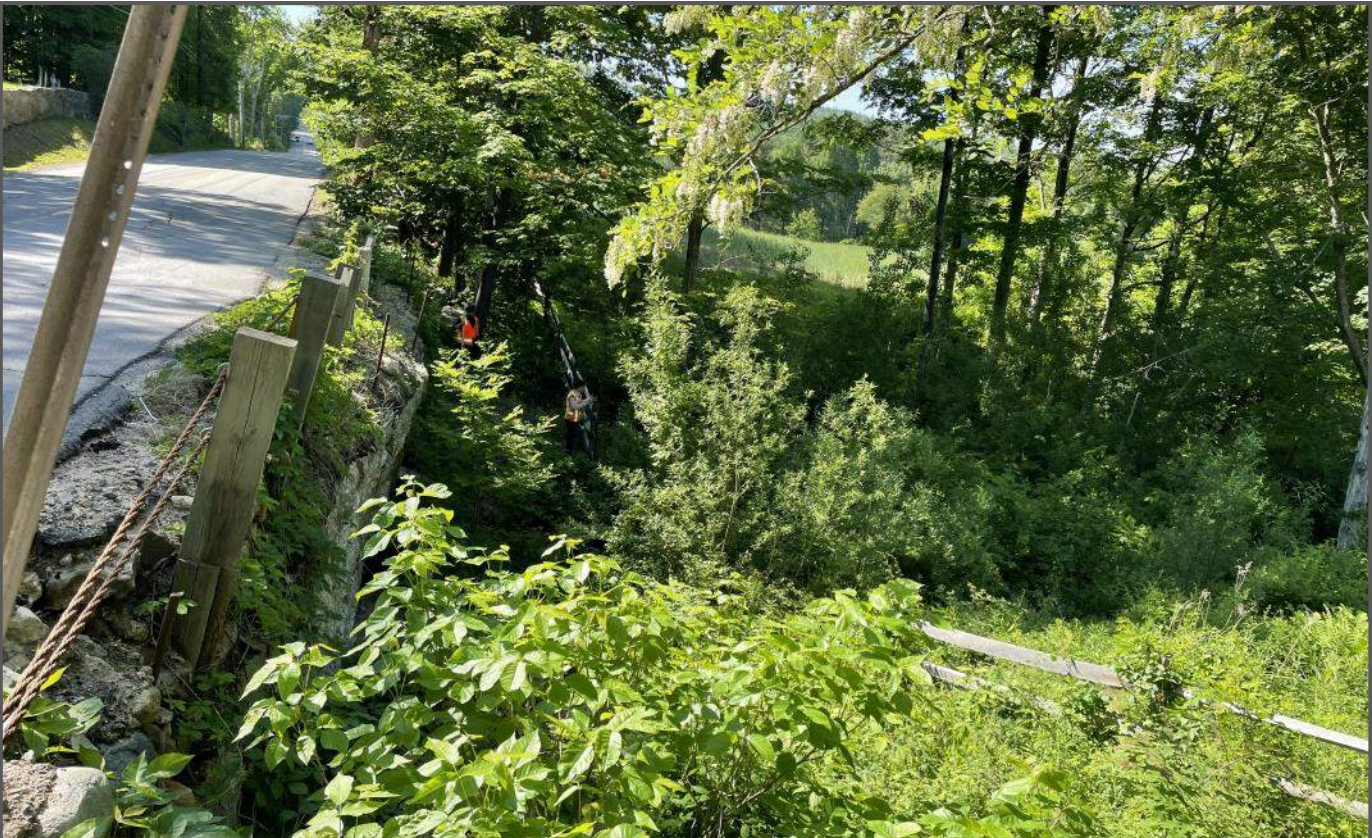
Photo 6: Looking Southeast Across Outlet
