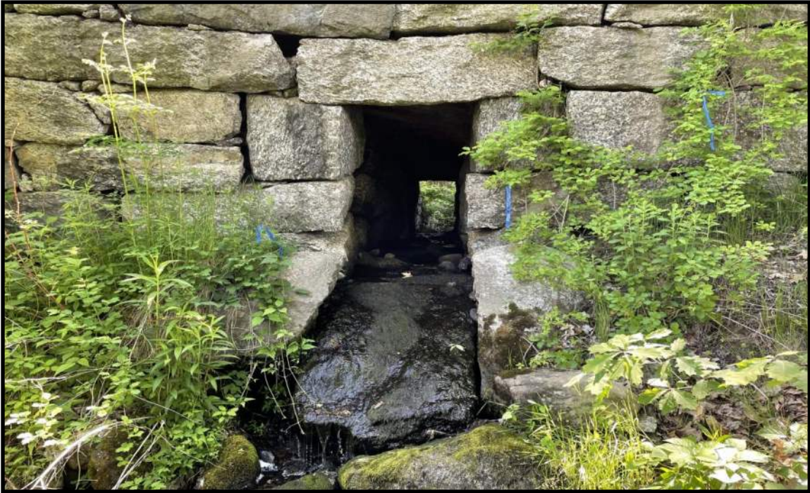
Photo 1: Outlet looking upstream
