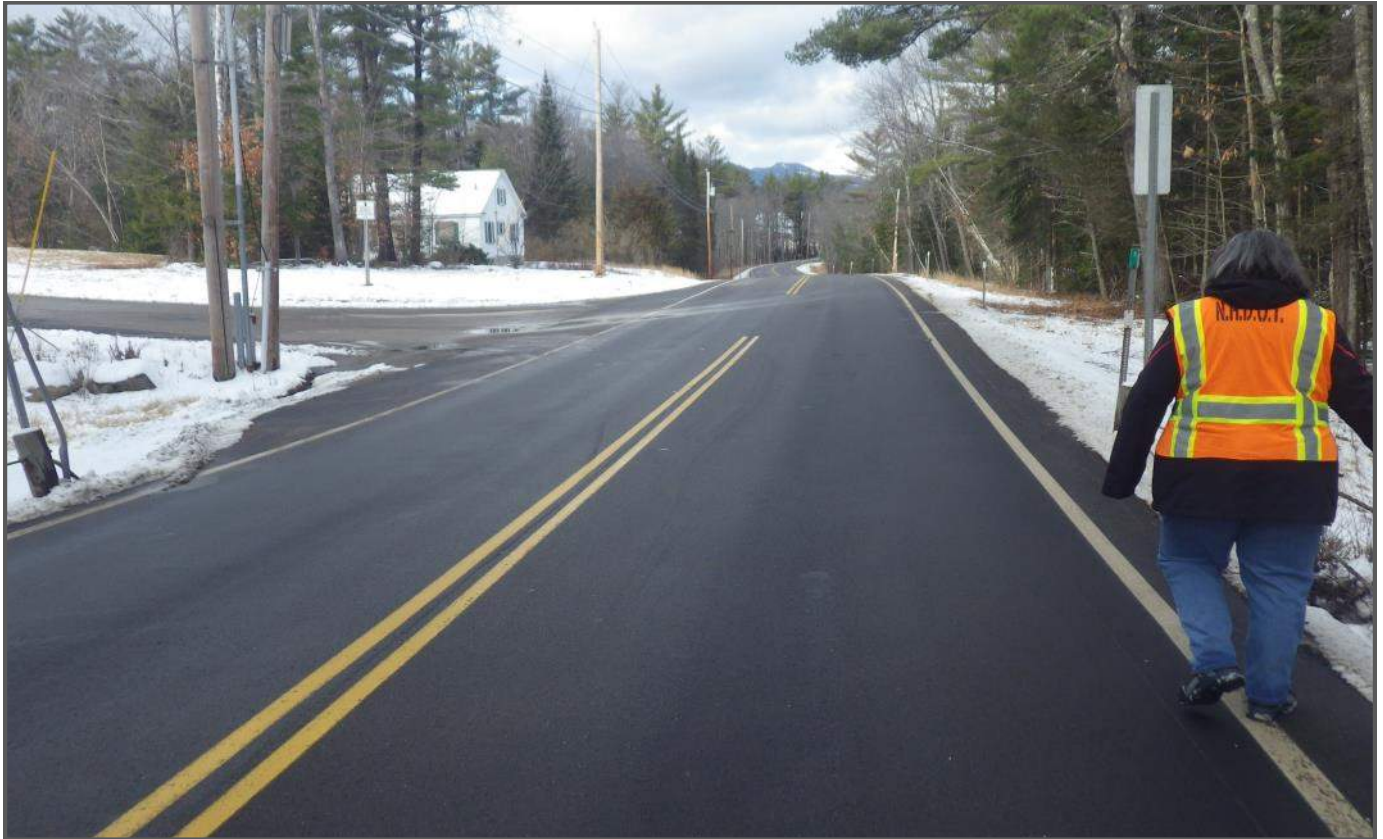
Photo 1: Looking Northwest along Route 153 from crossing (Dec 2019)
