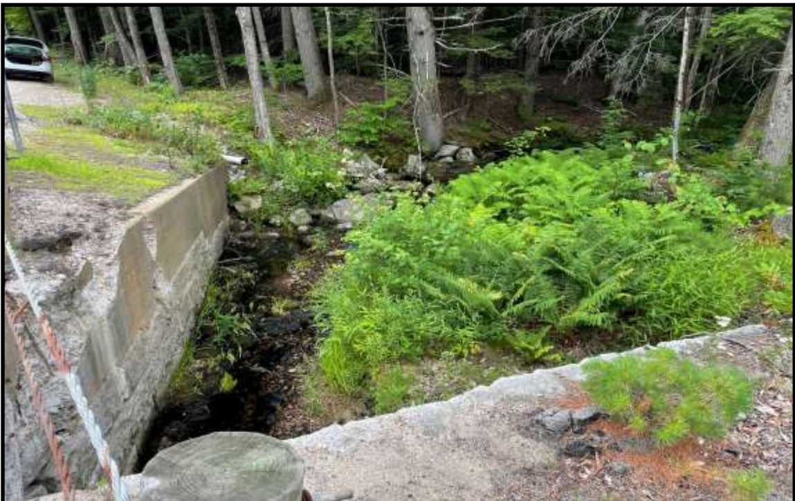
Photo 4: Inlet looking upstream
