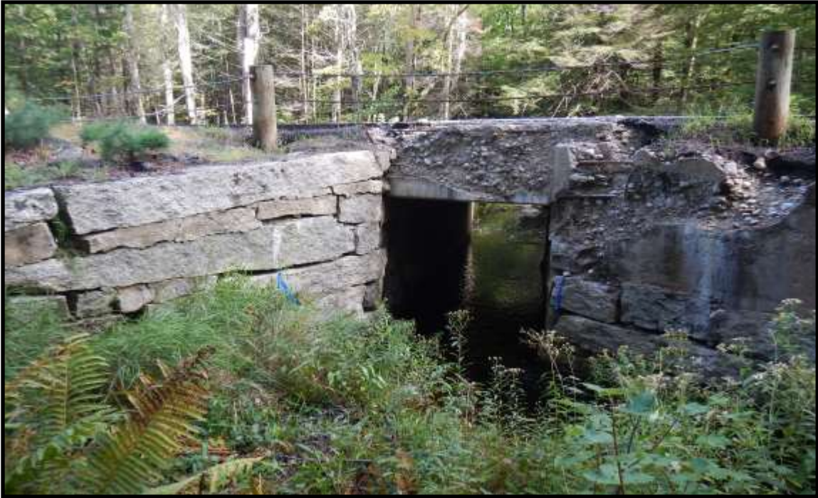
Photo 3: Inlet looking downstream
