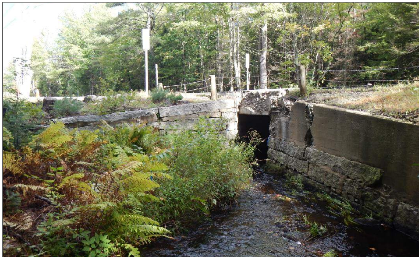
Photo 3: Inlet Looking Downstream (Sept 2021)
