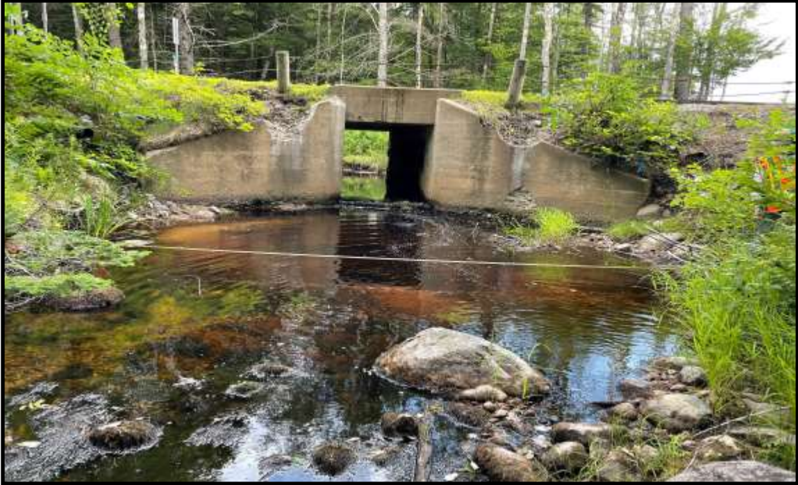
Photo 1: Outlet looking upstream
