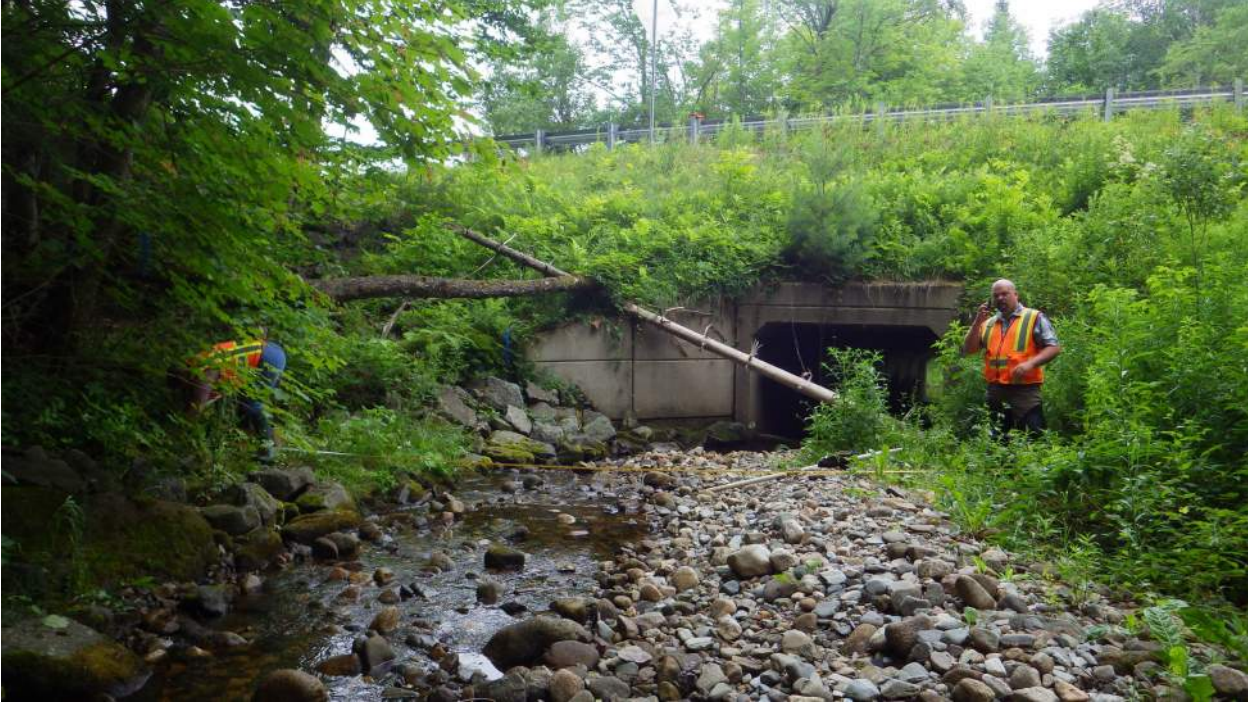
5. Upstream side looking towards the inlet (2021)
