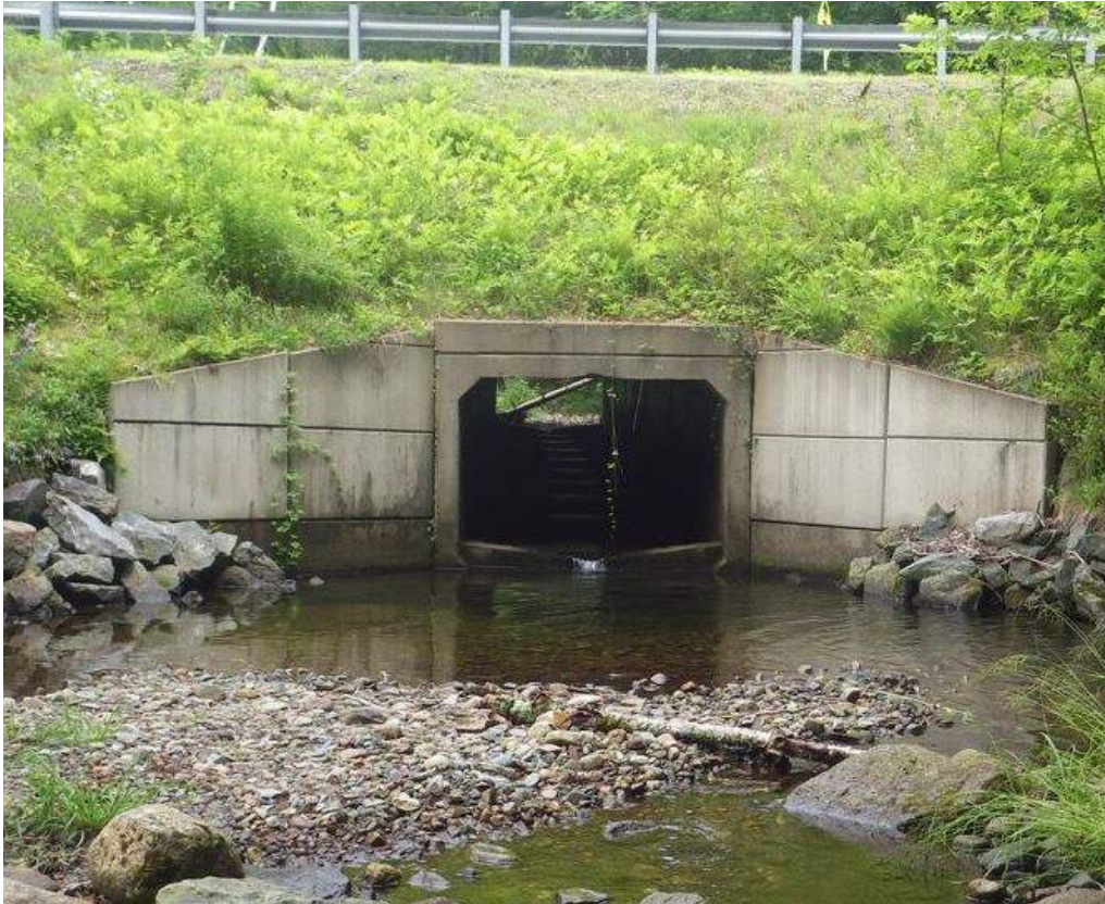
3. Downstream side looking at the outlet (2021)
