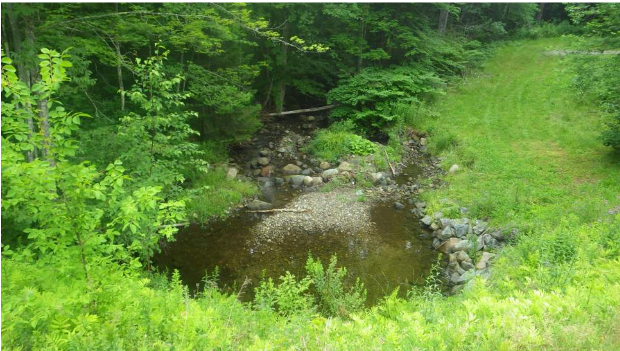
4. Looking downstream from the outlet (2021)
