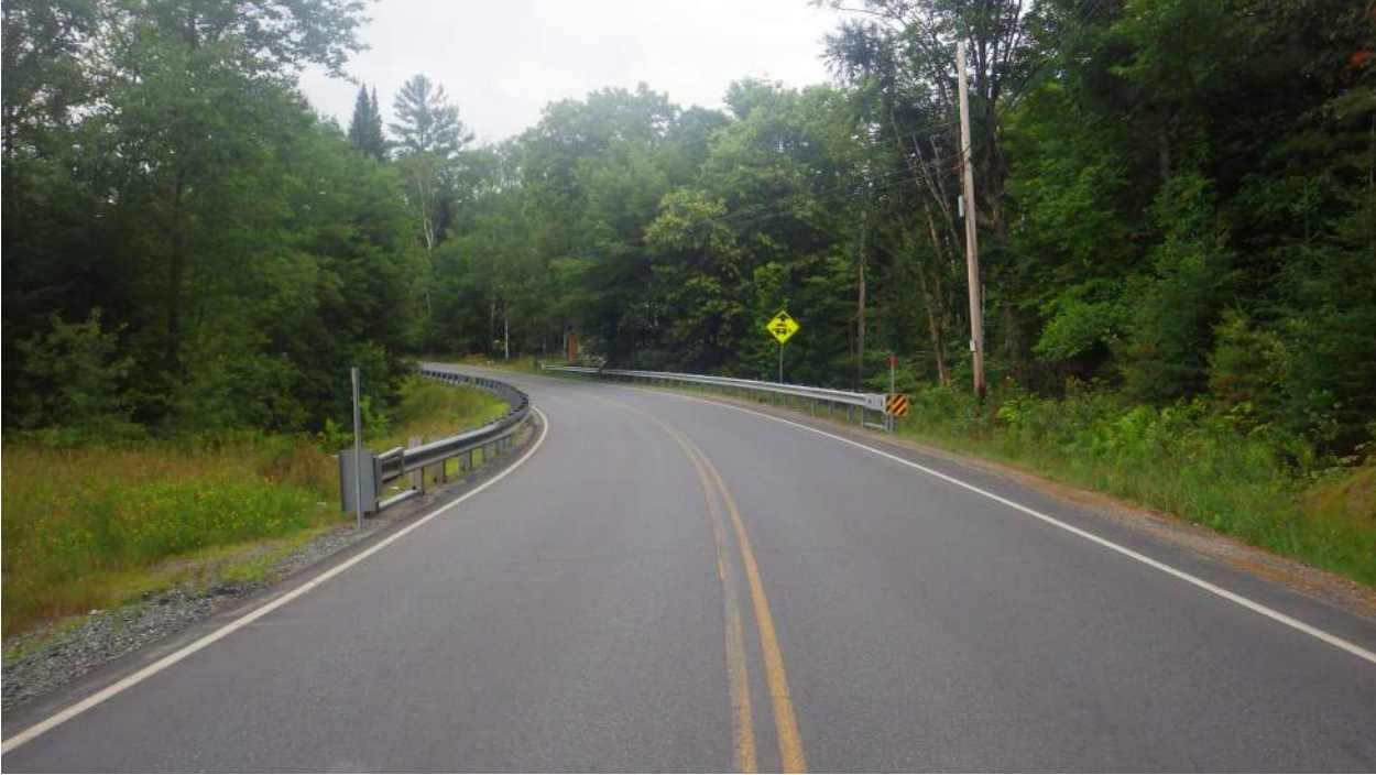
1. NH Route 135 looking easterly
