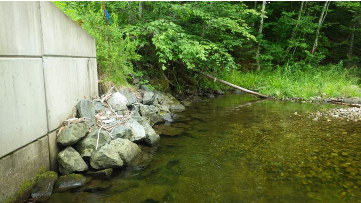
7. Existing rip rap, outlet side bank left (2021)
