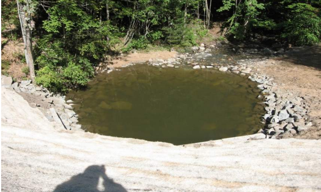
11. 2008-taken during construction at the outlet side looking downstream (for comparison)
