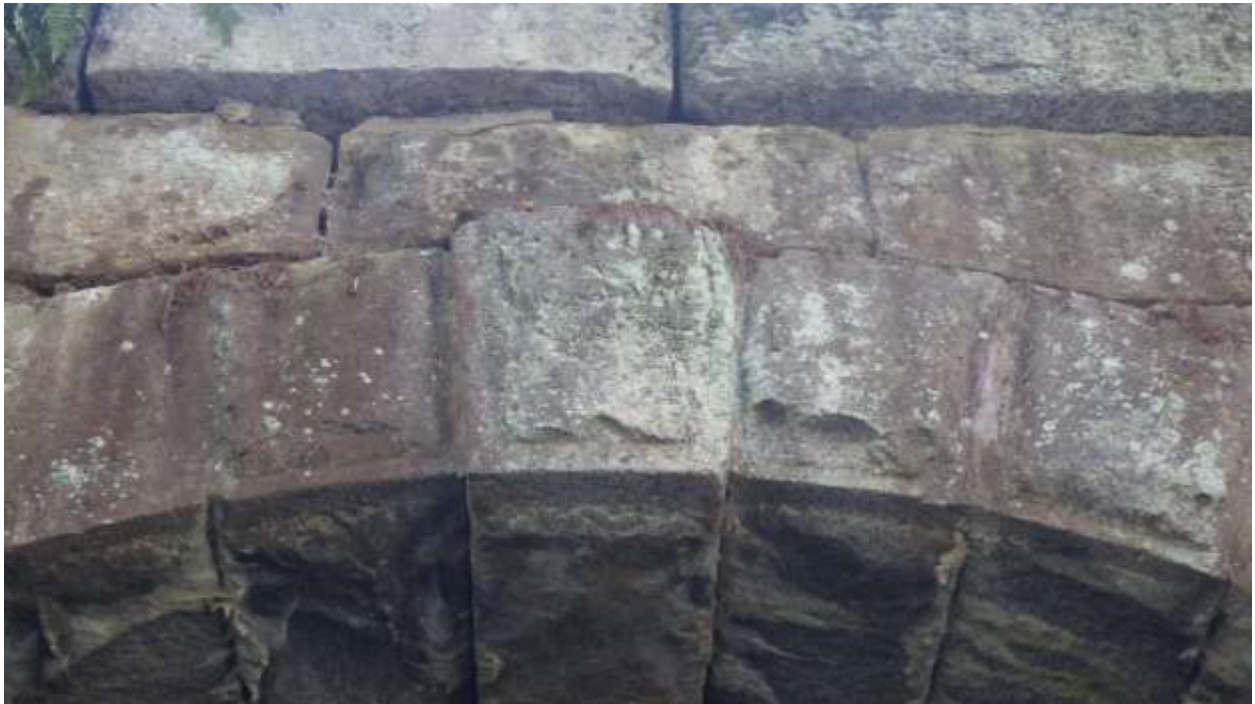
Figure 26. Looking west at northern barrel eastern end (inlet) keystone from upstream
