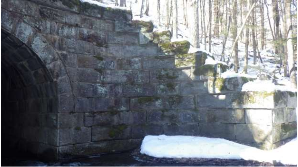
Figure 25. Looking west at northeast wingwall from upstream
