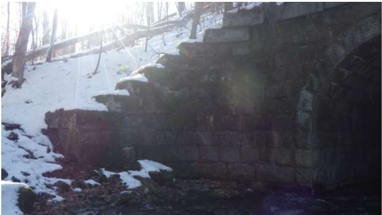
Figure 24. Looking west at southeast wingwall from upstream
