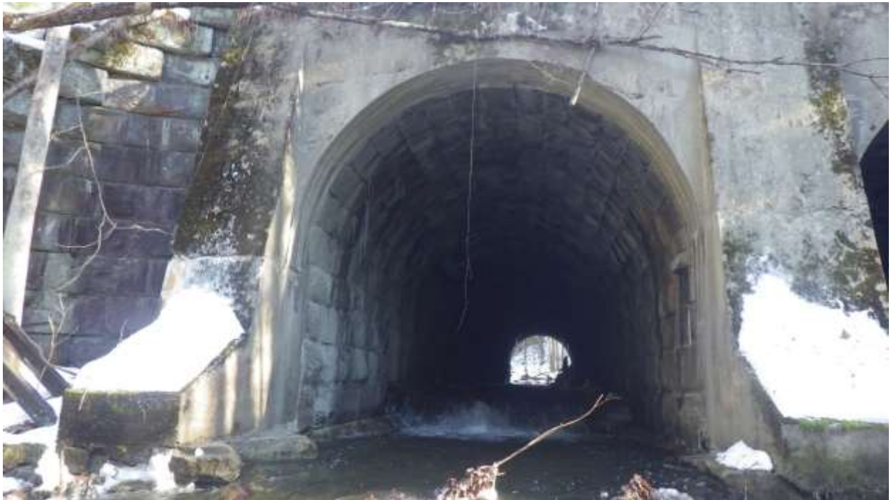
Figure 8. Looking east at north barrel outlet from downstream
