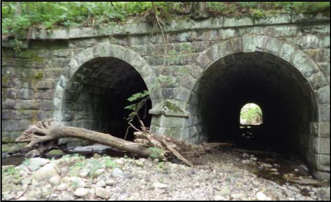
Photo 3: Inlet looking downstream
