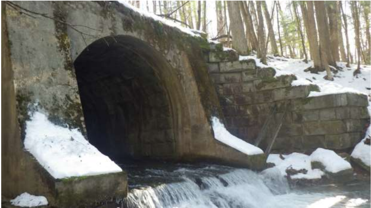
Figure 11. Looking east at south barrel outlet and southwest wingwall from downstream
