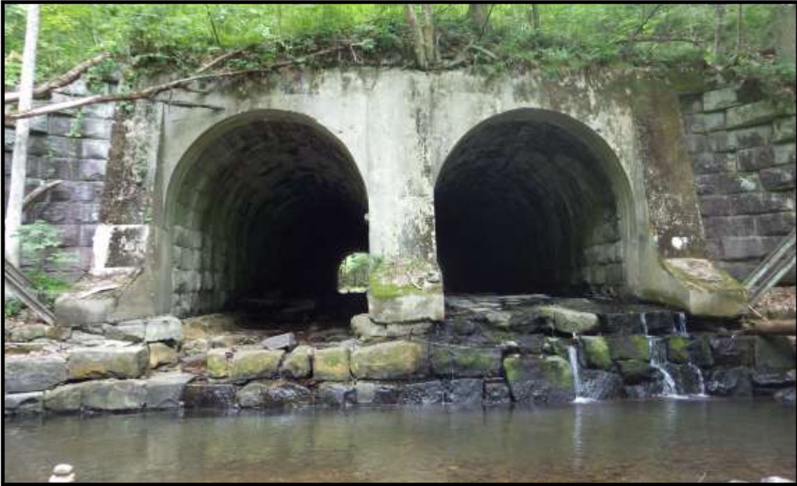
Photo 1: Outlet looking upstream
