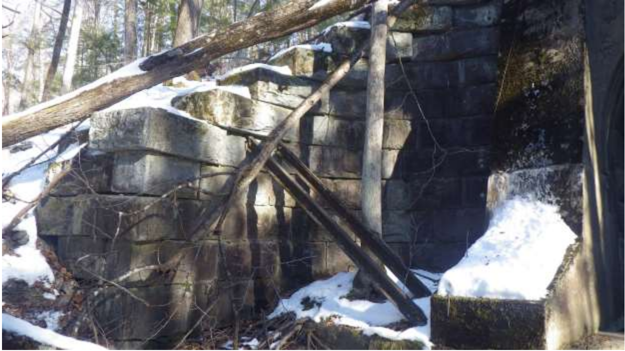
Figure 9. Looking at east at northwest barrel wingwall from downstream
