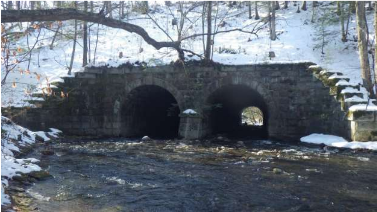
Figure 23. Looking west at inlet from upstream
