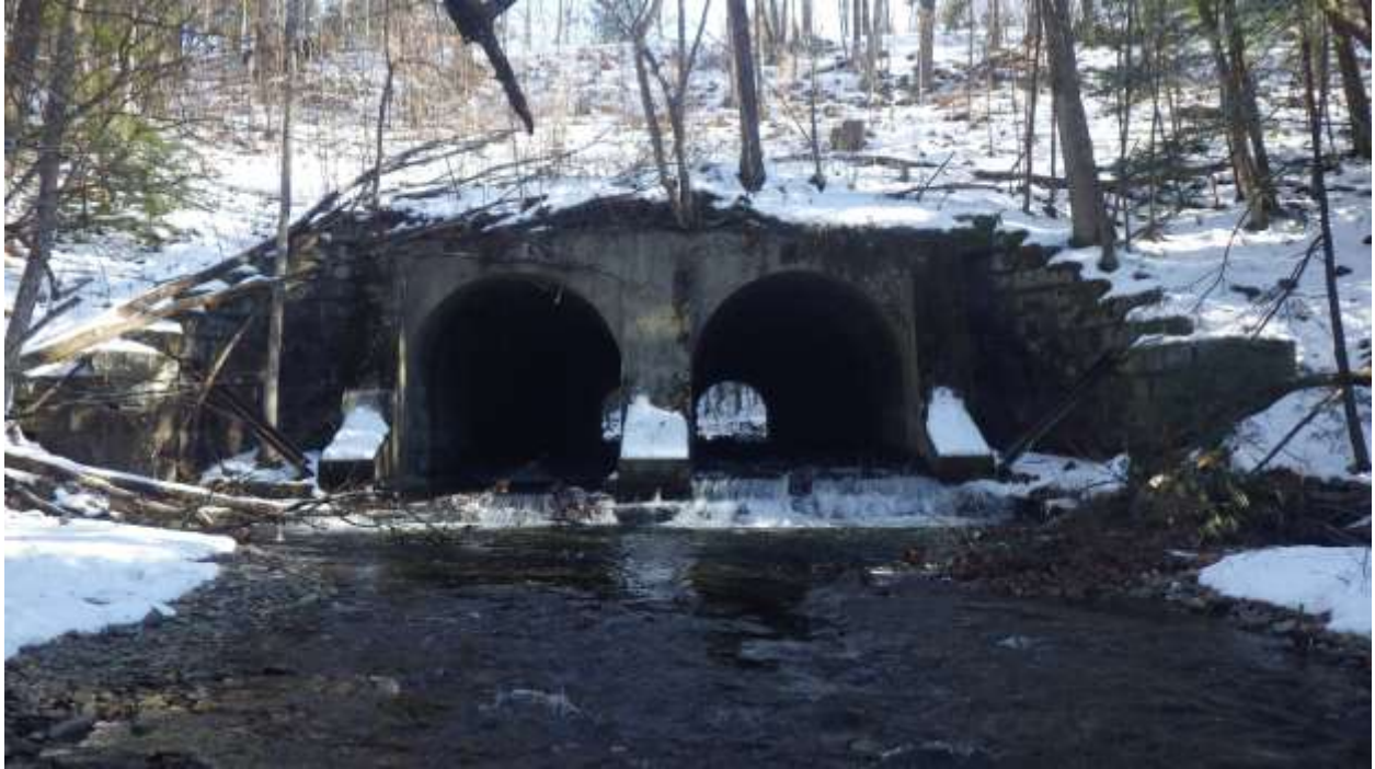
Figure 5. Looking east towards outlet from downstream
