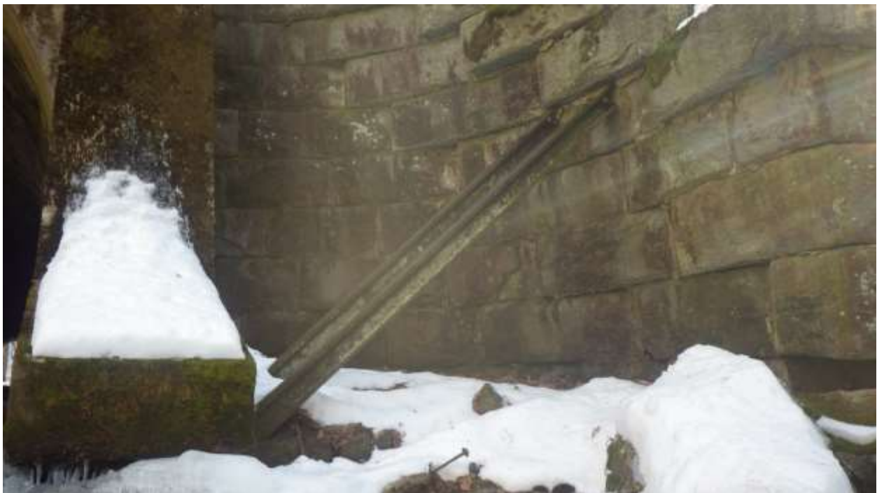
Figure 12. Looking east at southwest wingwall and railroad tie support from downstream
