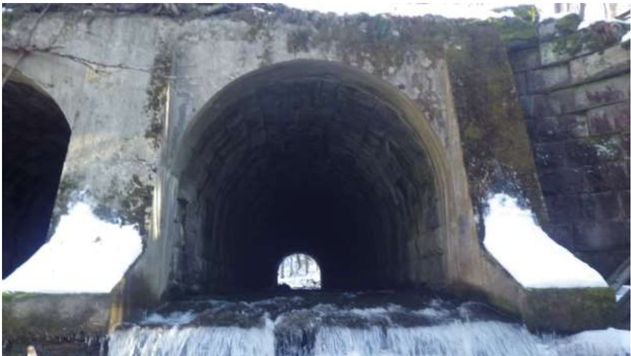
Figure 10. Looking east at south barrel outlet from downstream
