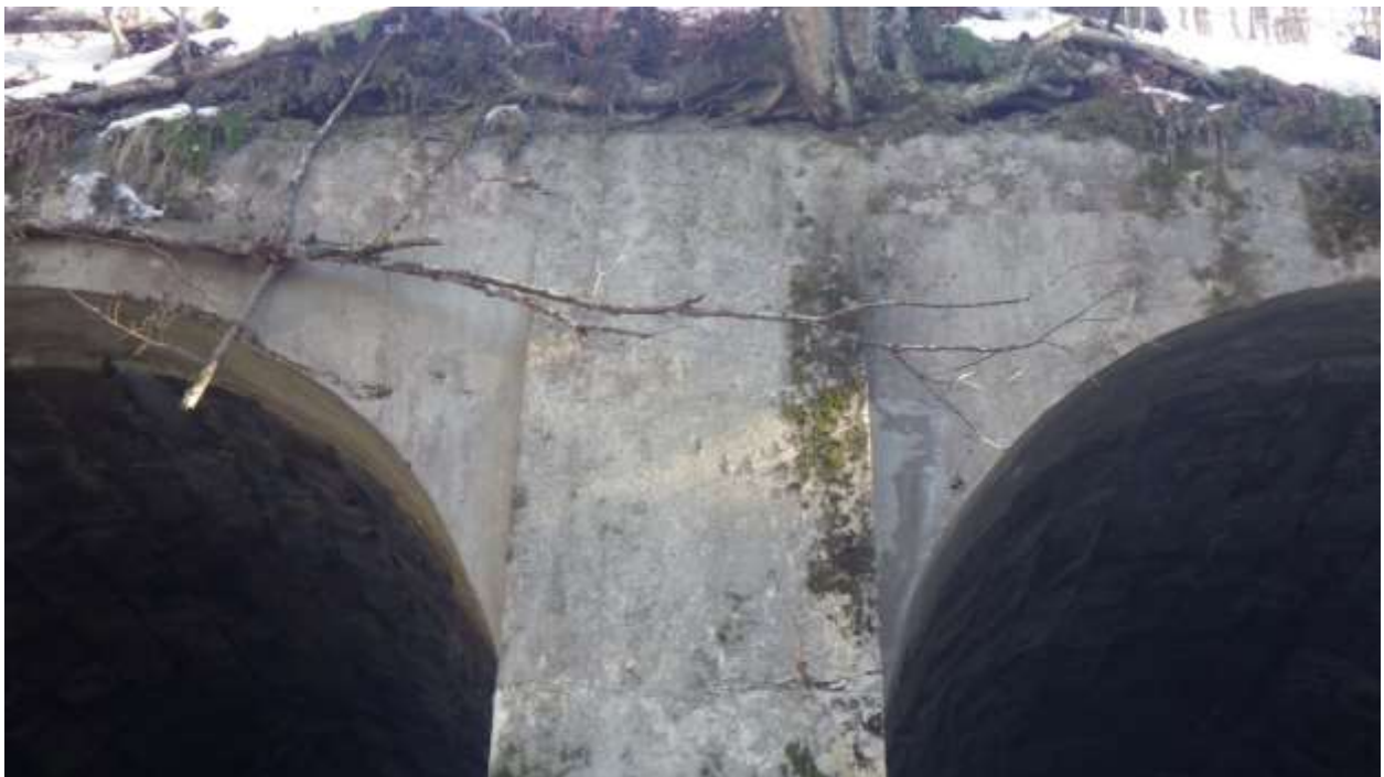
Figure 6. Looking east at top of outlet center buttress support from downstream
