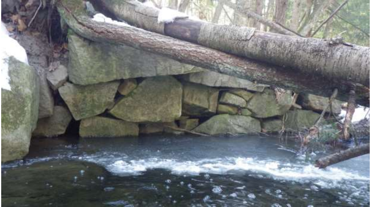
Figure 13. Looking south at the southwest wingwall 15' extension from the outlet
