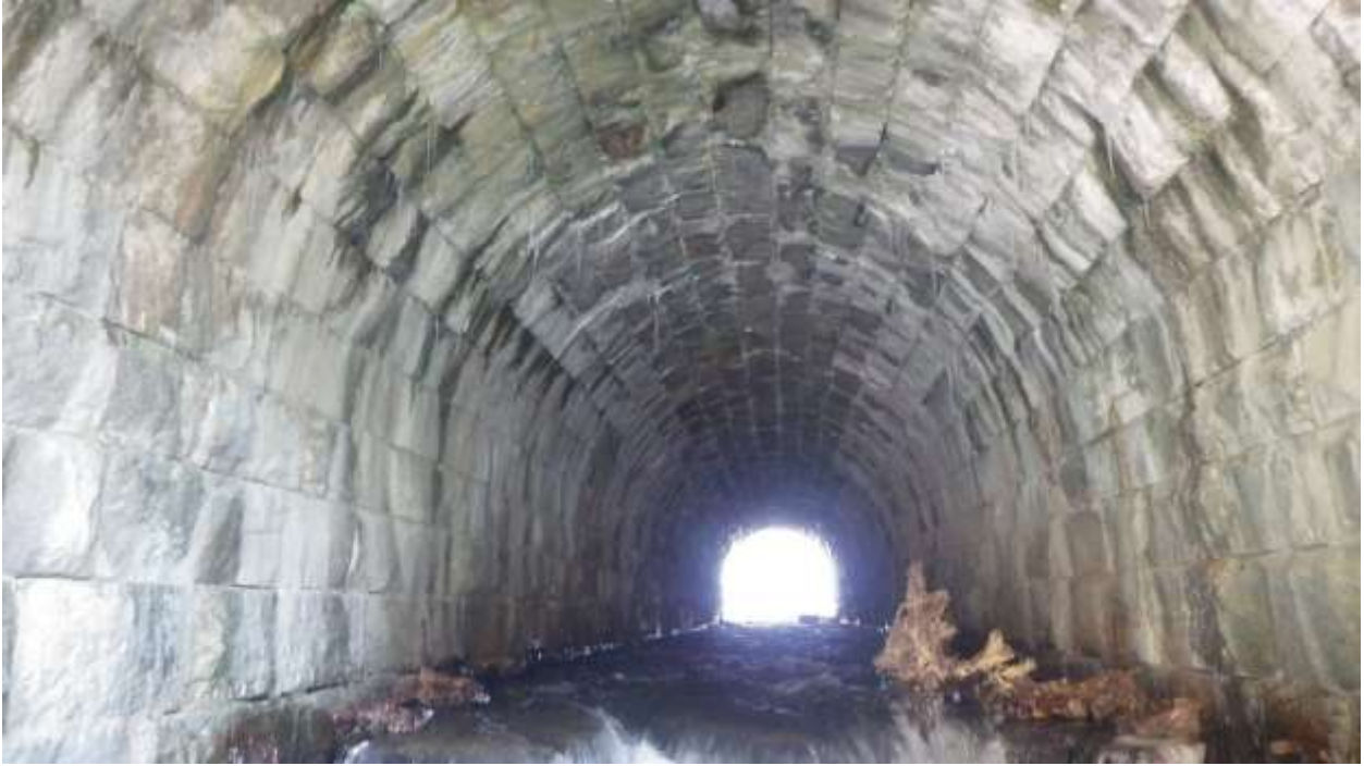
Figure 15. Looking east through the north barrel from the outlet
