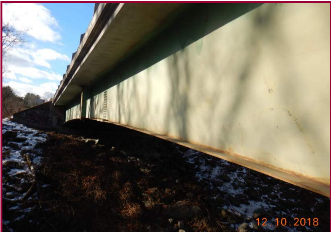
Upstream face of bridge looking west.
