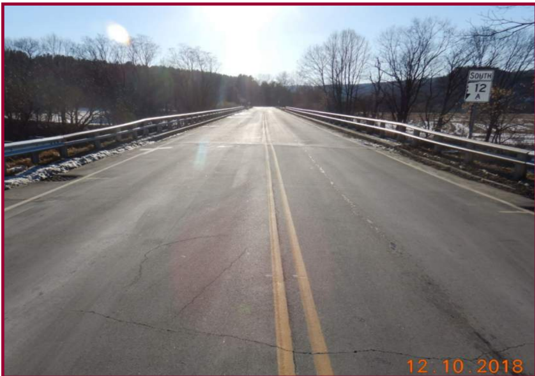
NH Route 12A roadway approach looking west.
