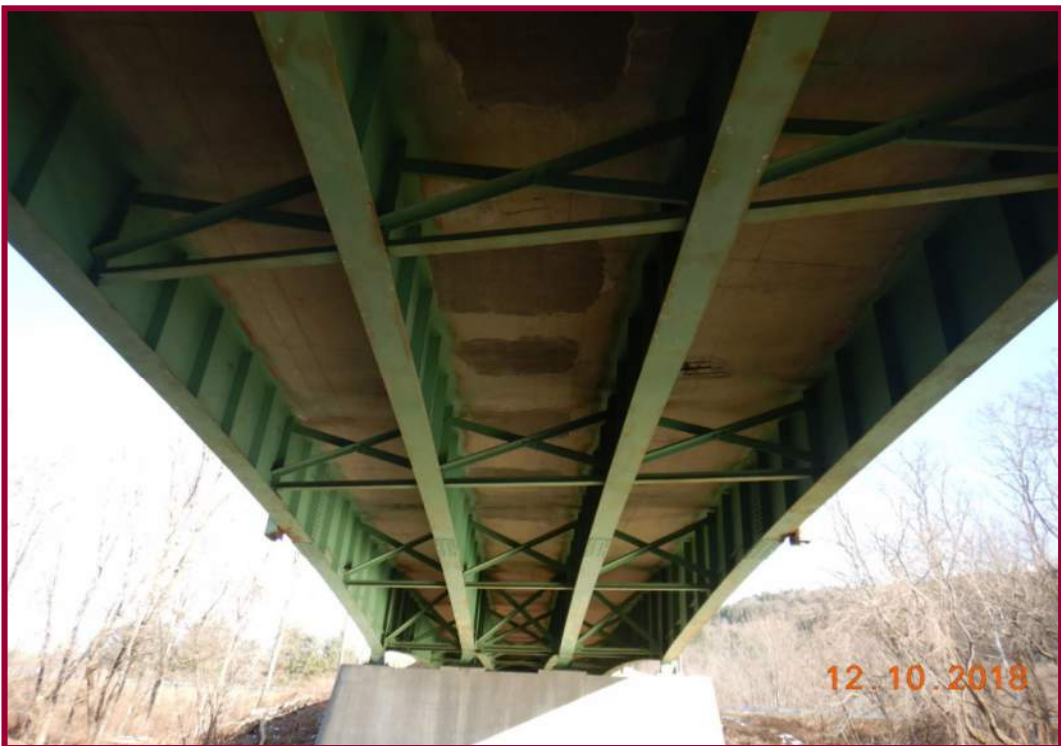
Superstructure conditions, typ.
