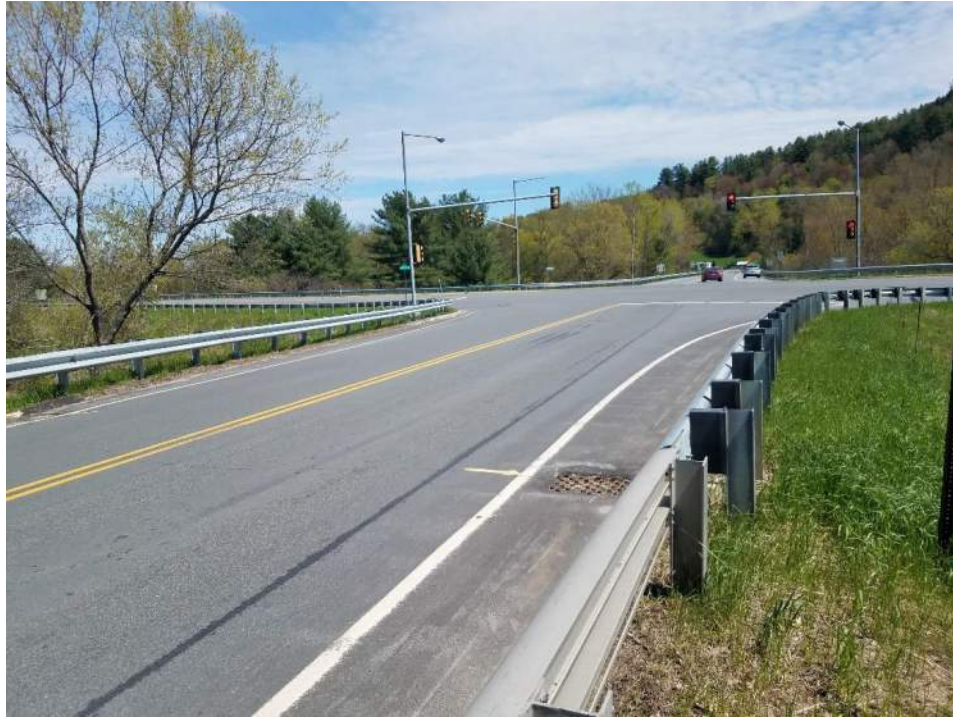
Photo 7: View of the Intersection between NH Route 12A and Route 103 on the eastern bank of the project area
