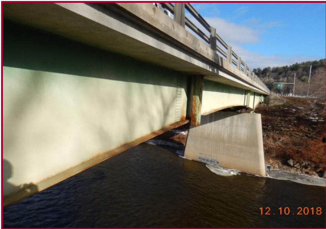
Upstream face of bridge looking east.
