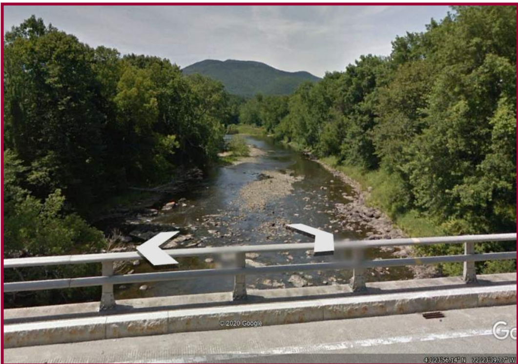
Downstream Channel (Google Earth Imagery 07/2012).
