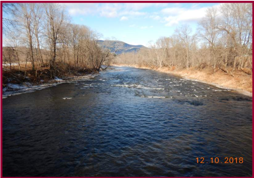
Downstream channel looking northwest.
