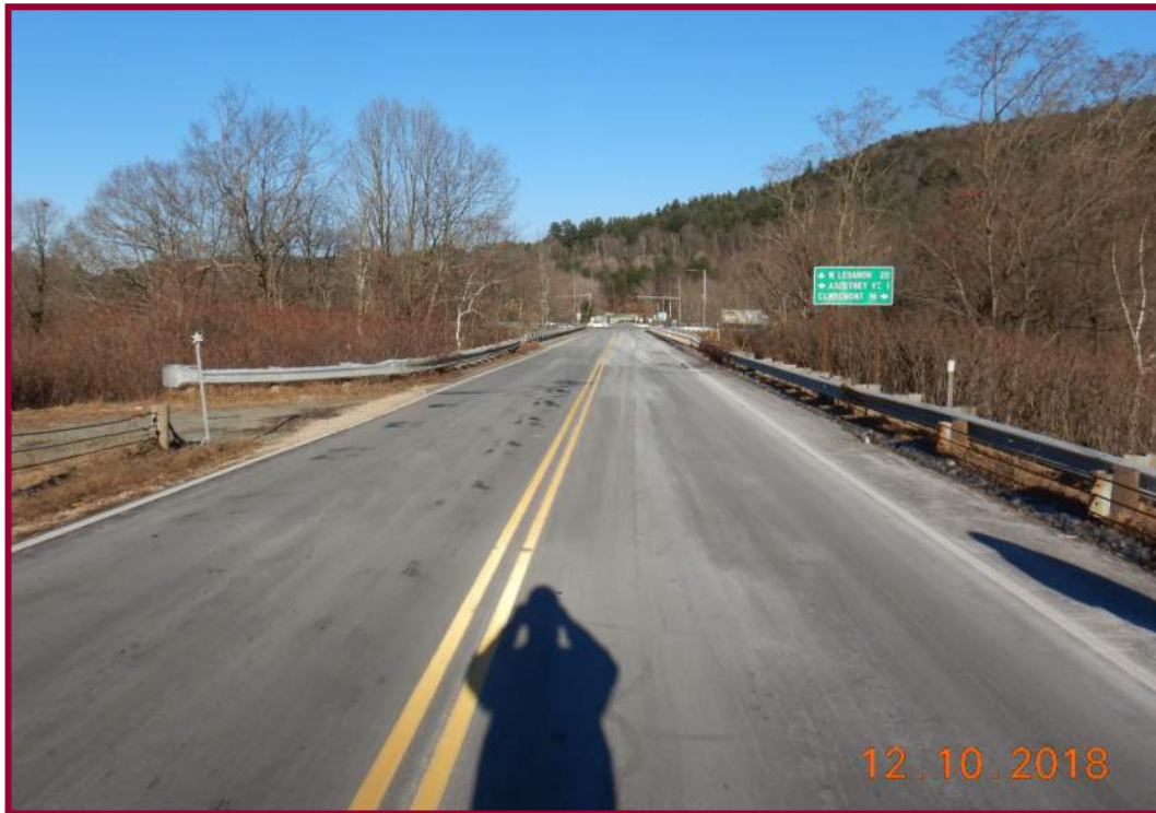
NH Route 12A roadway approach looking east.
