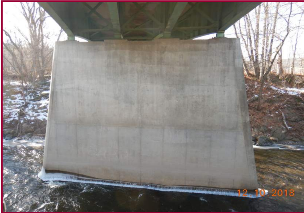
Western pier looking west.
