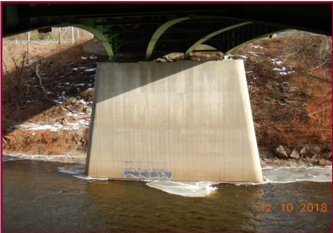
Eastern pier looking east.
