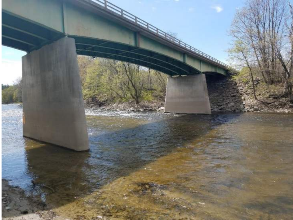
Photo 5: View of the underside of Bridge 072/127 and Sugar River
