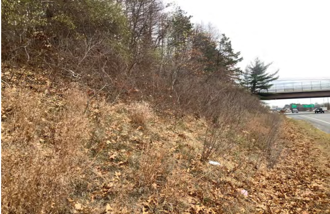
Photo 1: View northeast toward Sherburne Road of the western end of the proposed Pannaway Manor Soundwall Area. Note the Sherburne Road overpass bridge in the background.
