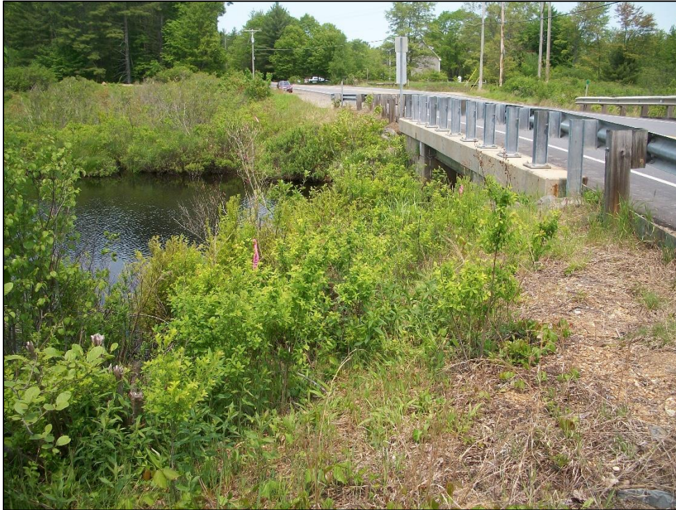
Photo 3. View north of downstream side of Bridge No. 141/127. Photo taken on 5/31/2019.
