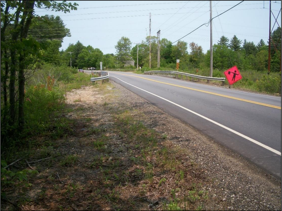
Photo 6. View north along NH Route 152 toward Bridge No. 141/127. Photo taken on 5/31/2019.
