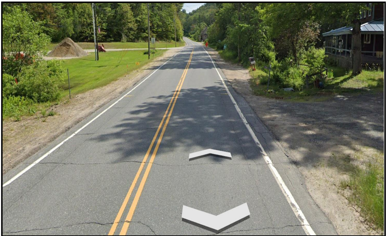
Photo 8: Roadway Looking Southbound Google Streetview
