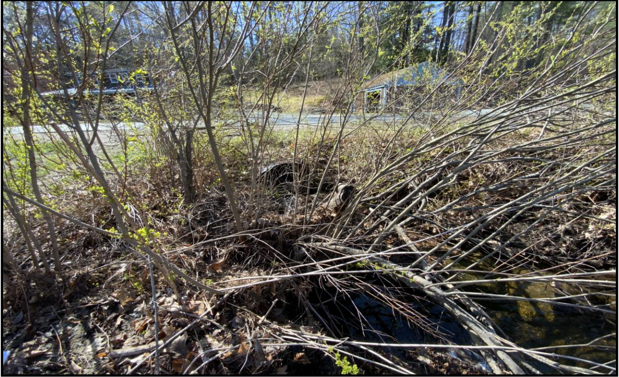
Photo 3: Culvert Outlet (4/28/23) J. Commerford
