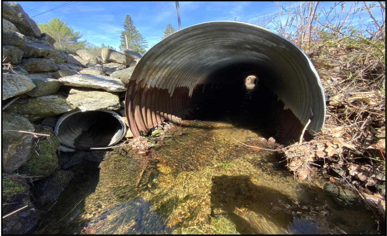
Photo 1: Culvert Inlet with 15" Stormwater Outfall (4/28/23) J. Commerford
