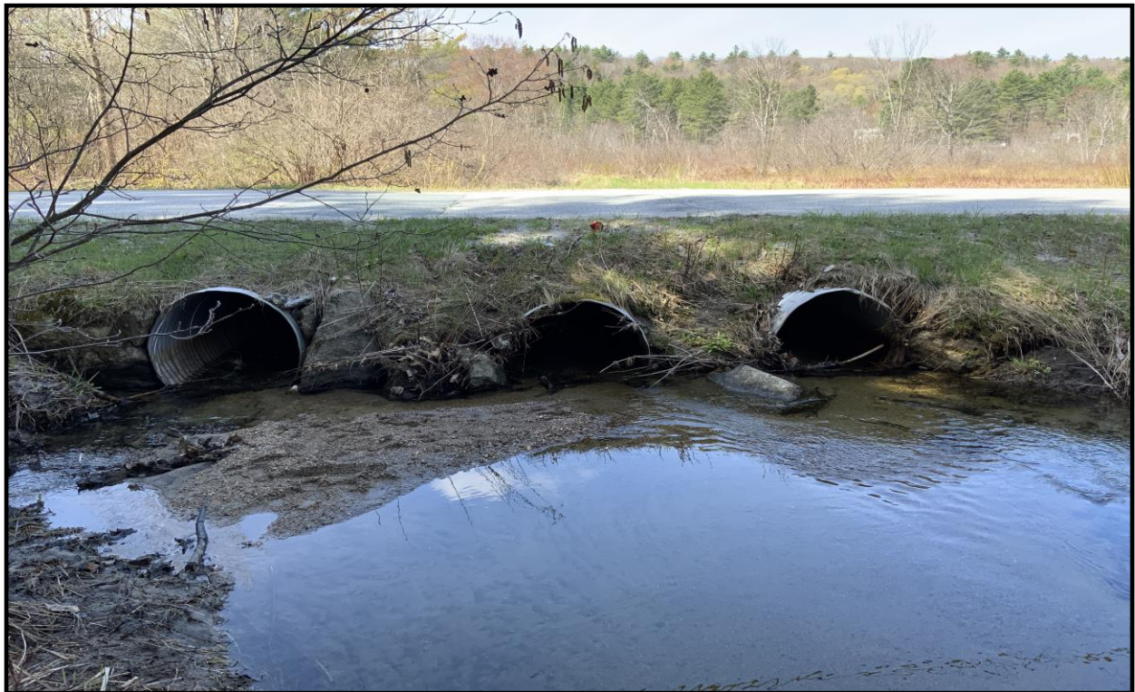
Photo 10: Downstream Main Street Culvert (3) 36" Pipes (Town of Sutton) (4/28/23) J. Commerford
