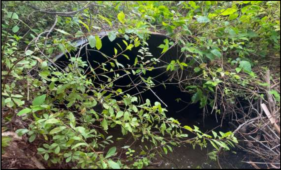
Photo 1: View of Outlet – Looking upstream
