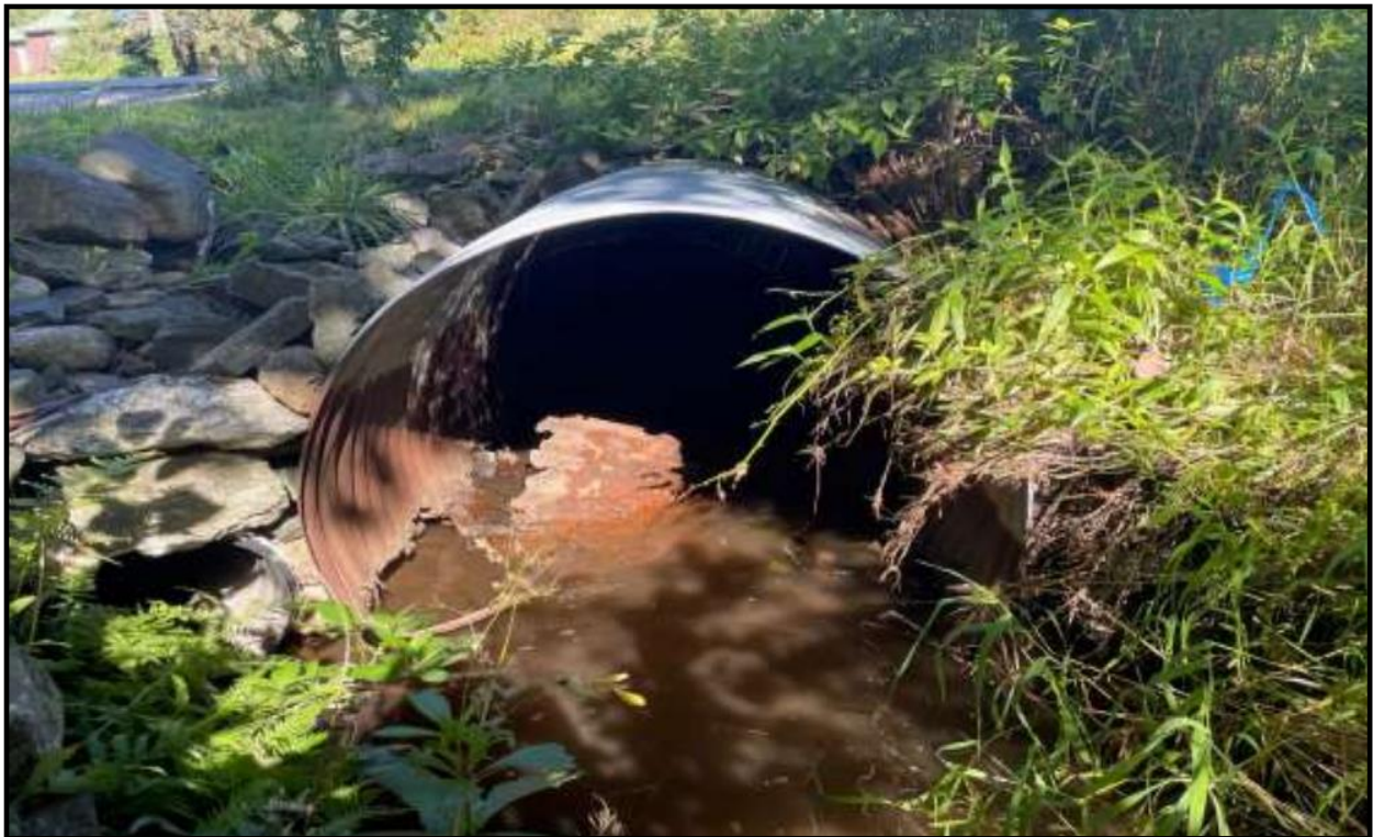
Photo 2: Culvert Inlet (8/14/23) M. Urban
