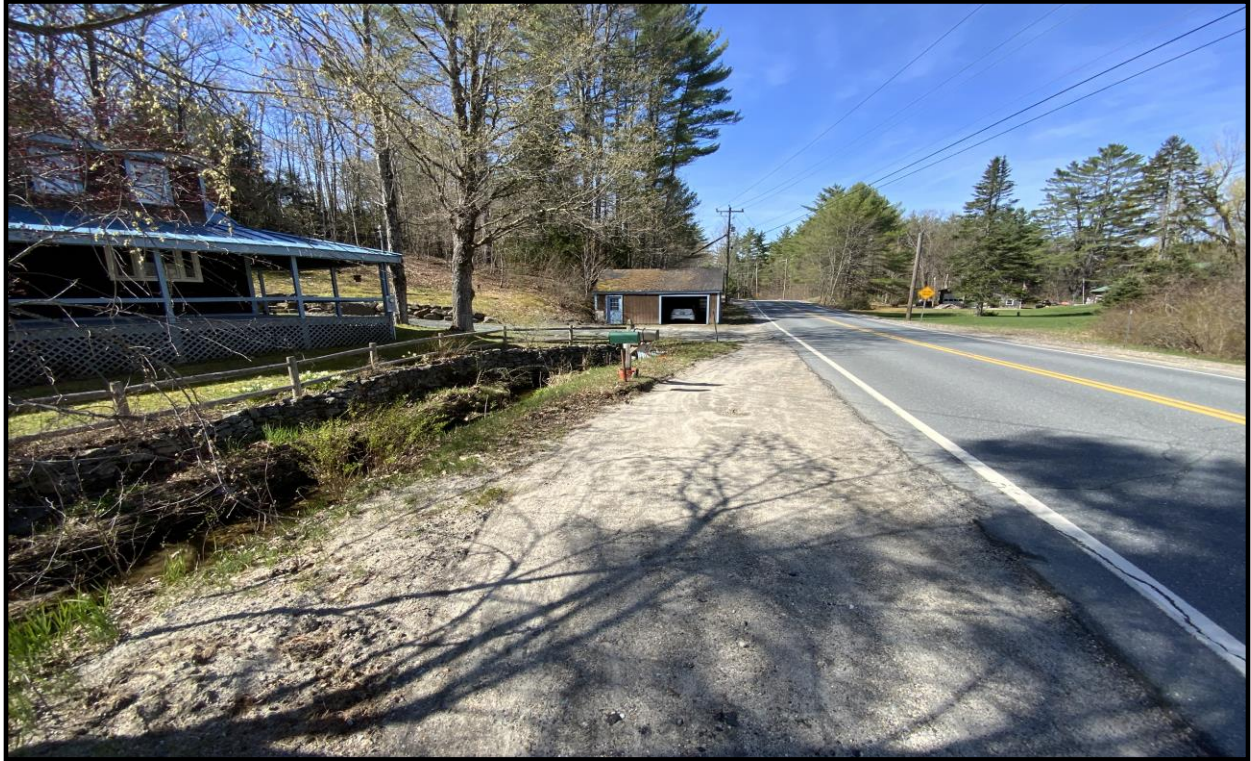
Photo 7: Roadway Shoulder on Inlet Side (4/28/23) J. Commerford
