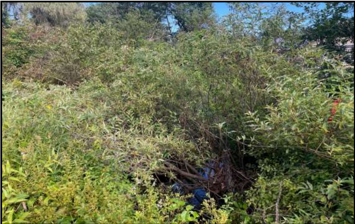
Photo 2: View of Outlet Area – Looking downstream
