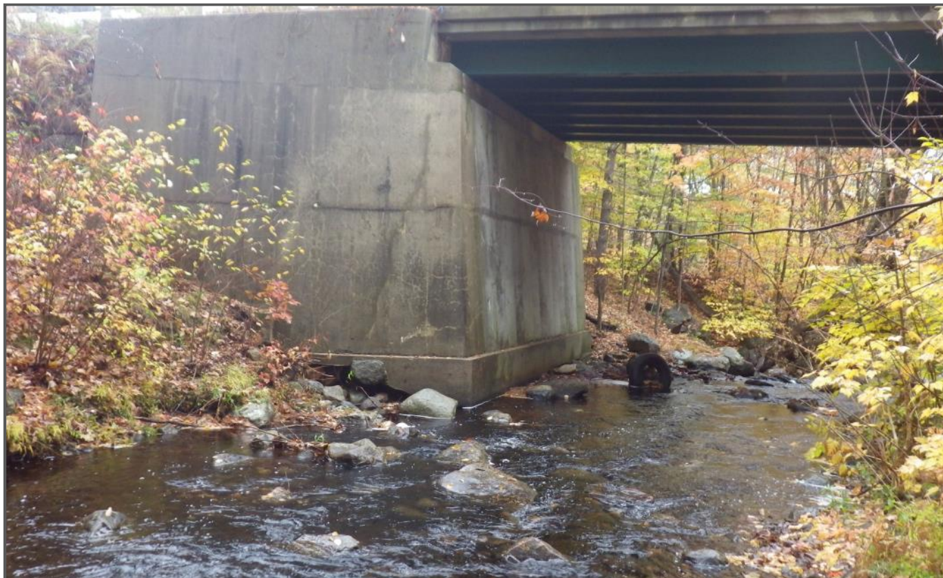
Photo 7: North abutment looking Northeast
