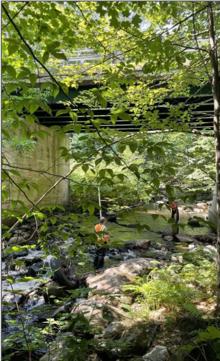
Photo 1: Looking Upstream at Outlet
