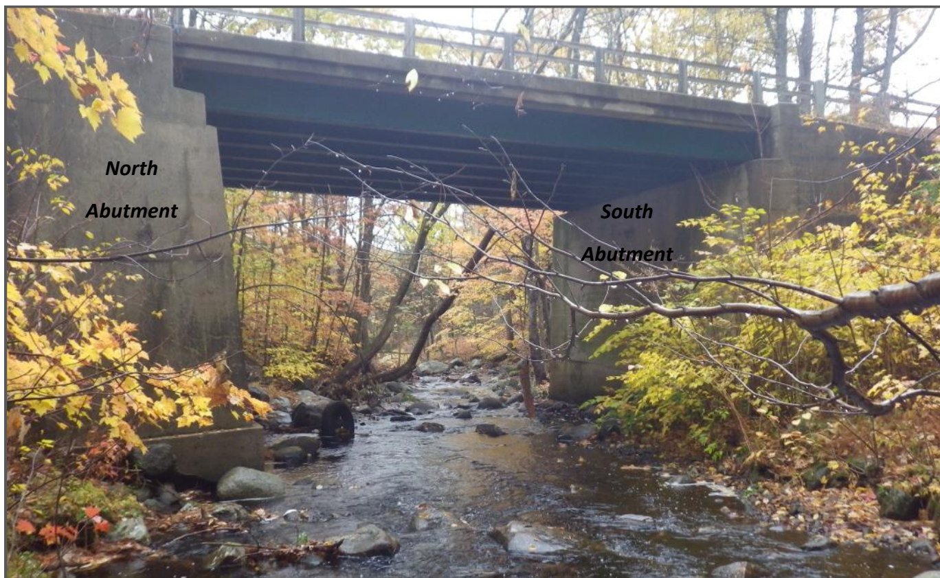
Photo 3: Looking East (downstream) at inlet
