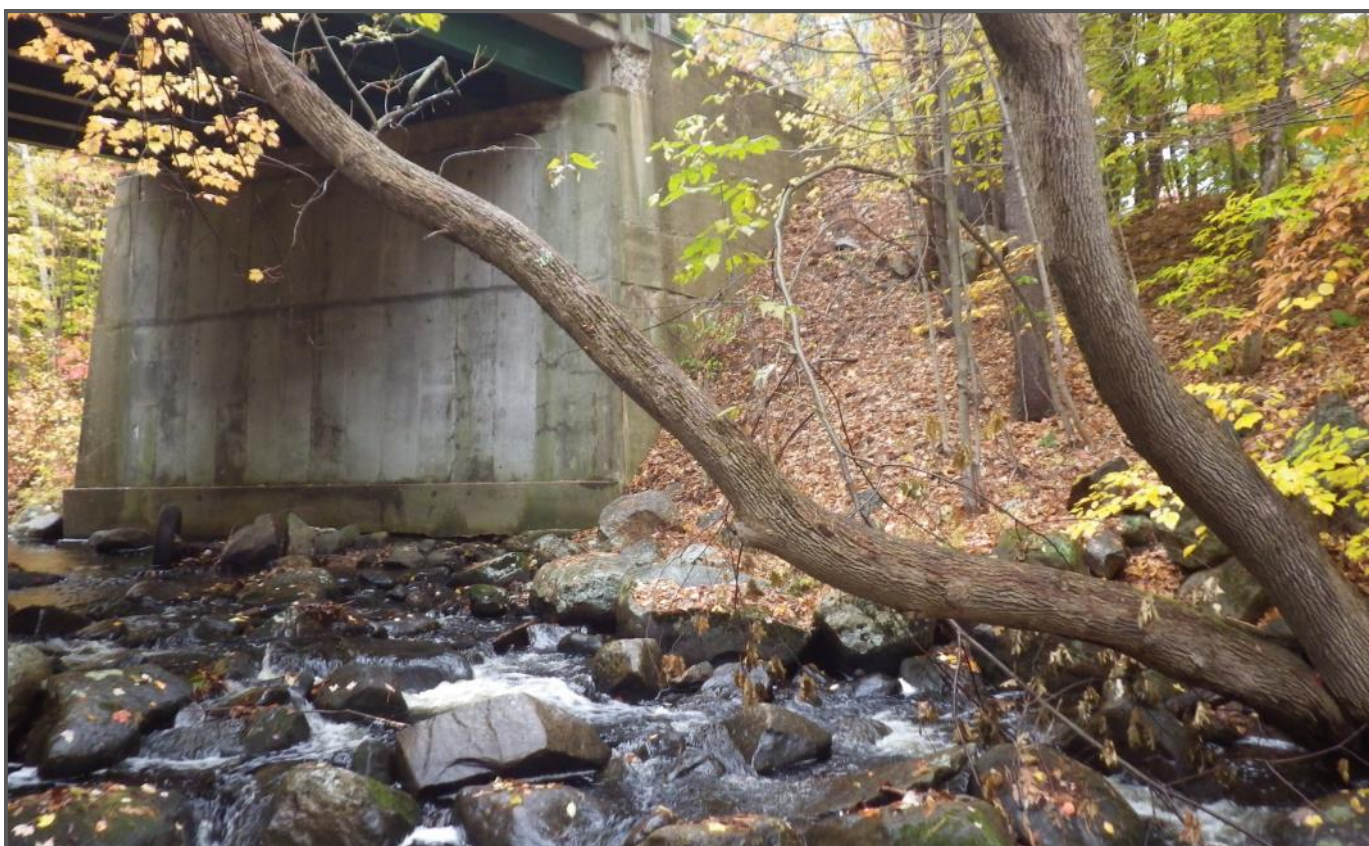
Photo 8: North abutment looking Northwest
