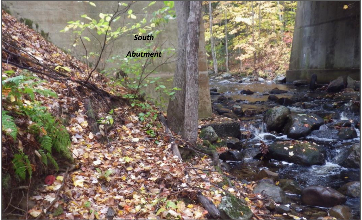
Photo 9: South abutment looking West (upstream)
