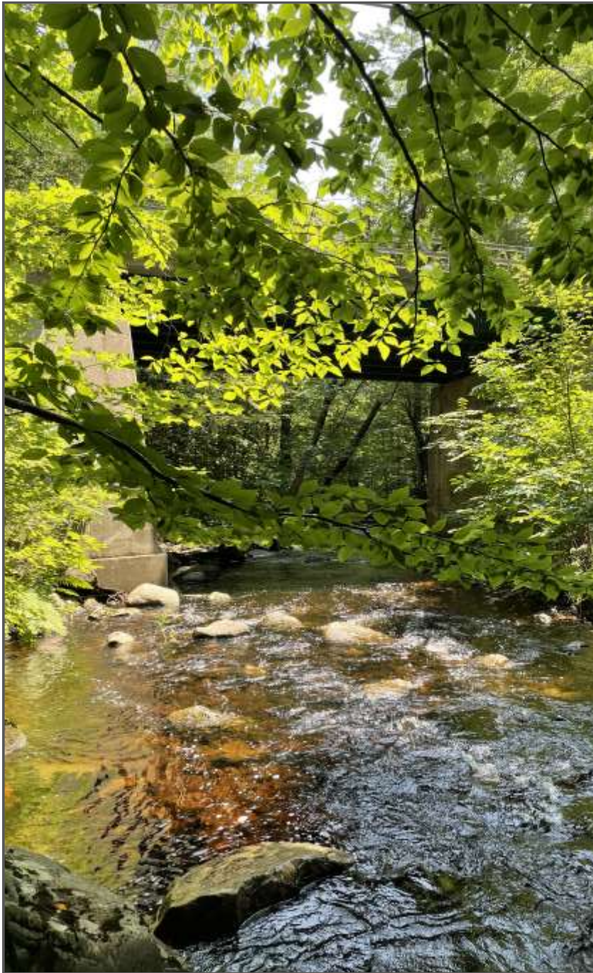
Photo 3: Looking Downstream at Inlet
