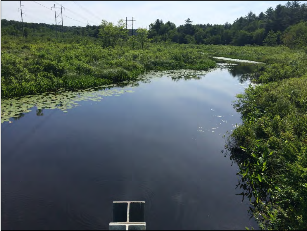
NH Route 152: On Bridge Looking Upstream
