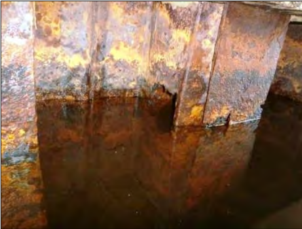
Bridge: Z-pile and H-pile holes at NE corner
