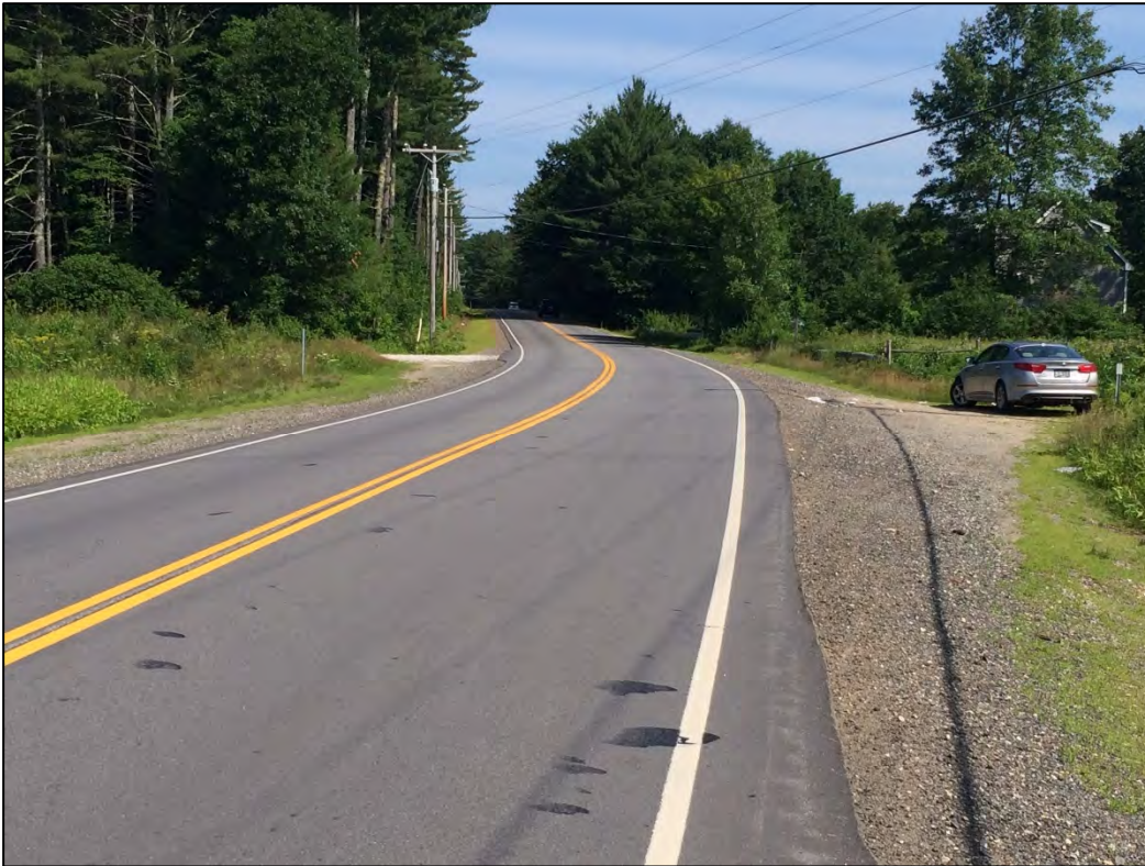
NH Route 152: North Approach Looking North
