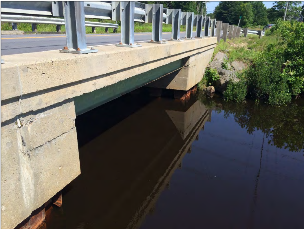
Bridge: East Fascia
