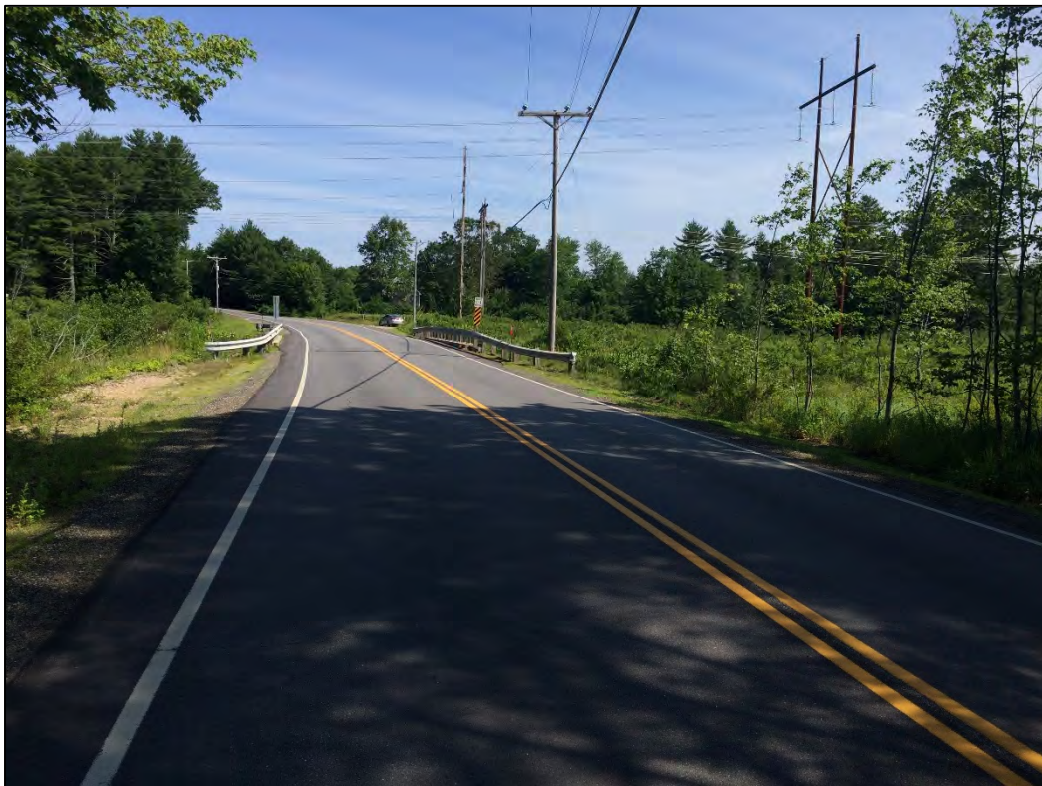
NH Route 152: On South Approach Looking North
