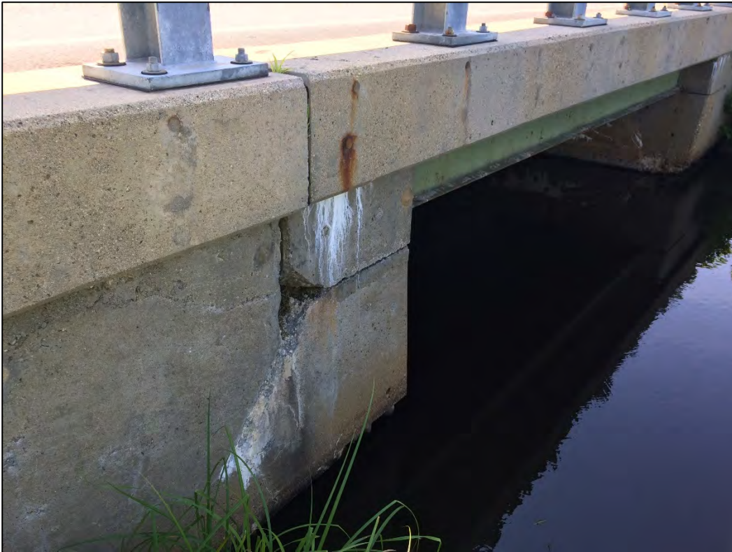
Bridge: West Fascia
