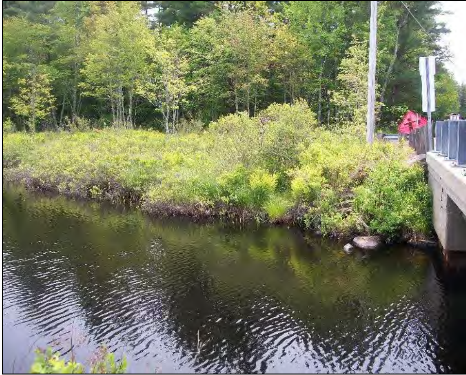
Wetland 6 (Flag Series C) southeast of bridge and south of the North River with forested portion further south View southeast Photo taken 5/31/19
