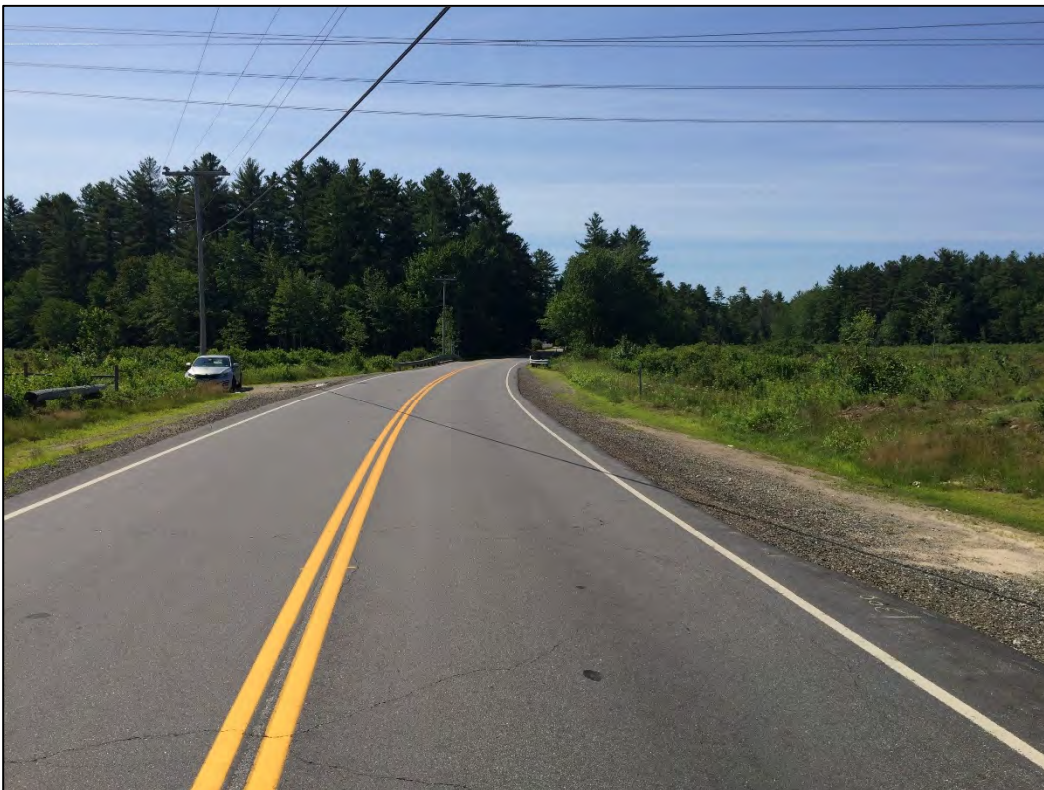
NH Route 152: North Approach Looking South
