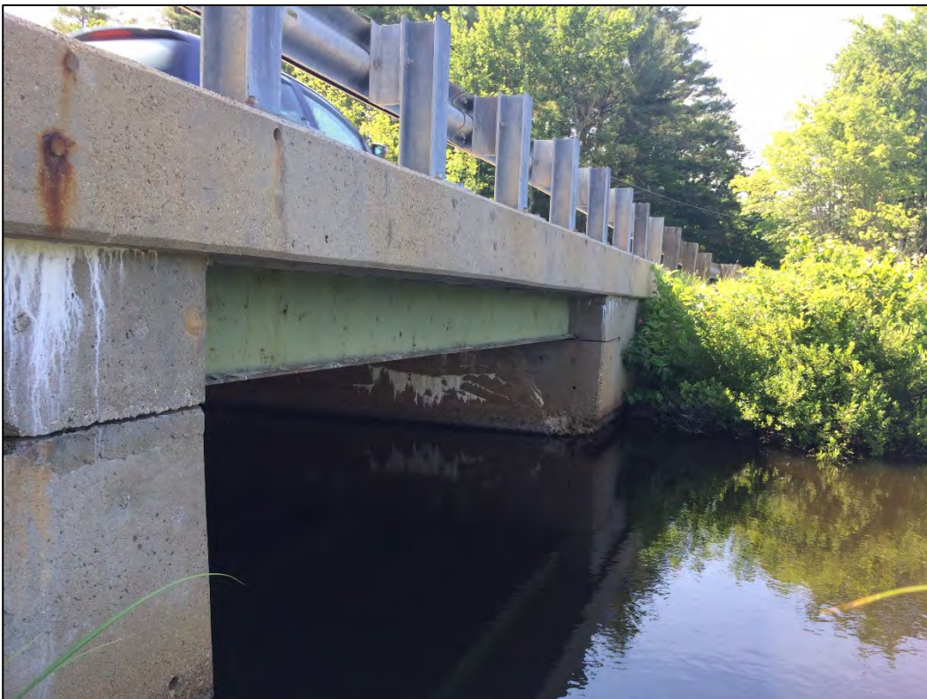
Bridge: West Fascia and South Abutment
