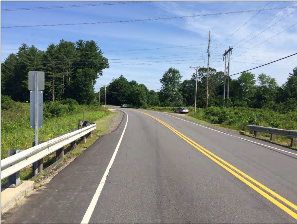
NH Route 152: On Bridge Looking North
