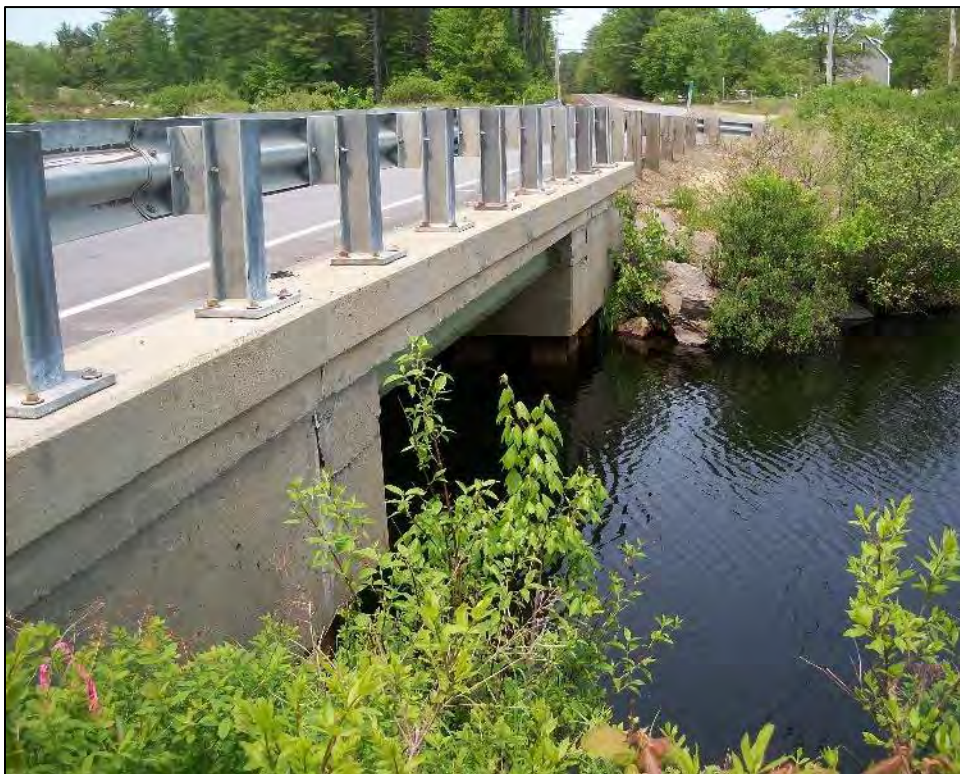
North River (upstream) at bridge View northwest Photo taken 5/31/19
