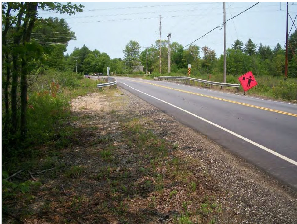
Photo 8. View north along NH Route 152 toward Bridge No. 141/127. Photo taken on 5/31/2019.
