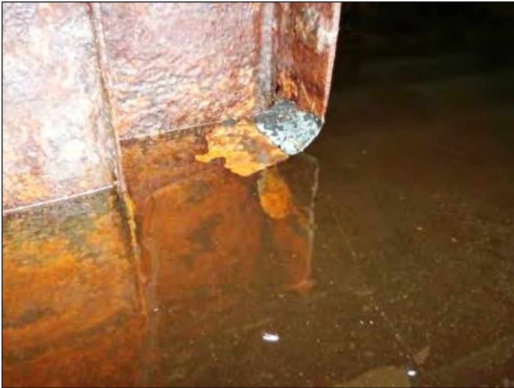
Bridge: H-pile hole at SE corner
