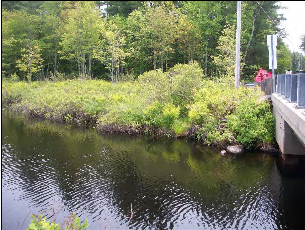
Photo 1. View south toward the North River and Wetland 6 (Impact Areas A, B, C, and D) in the southeast quadrant. Photo taken on 5/31/2019.
