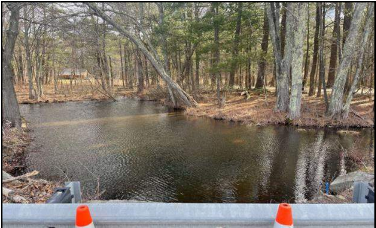
Photo 8: Upstream channel from Culvert (4/7/23) R. Thomson
