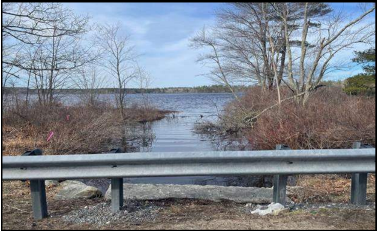
Photo 9: Looking Downstream towards the Culvert (4/7/23) R. Thomson
