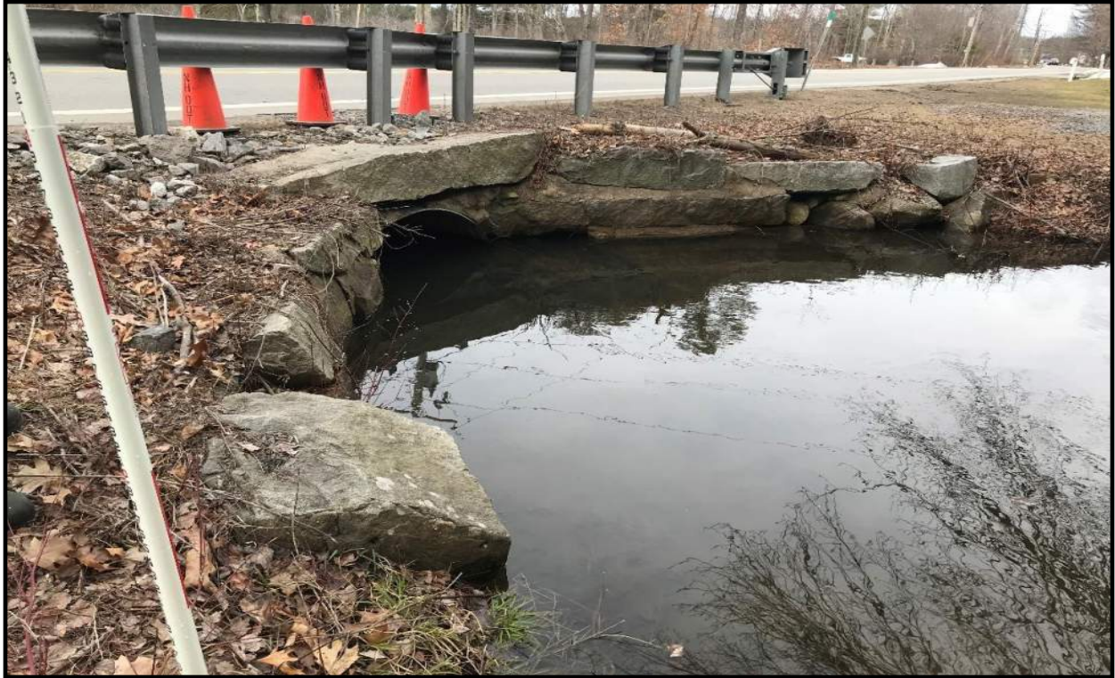
Photo 5: Culvert Inlet (3/24/23) J. Commerford
