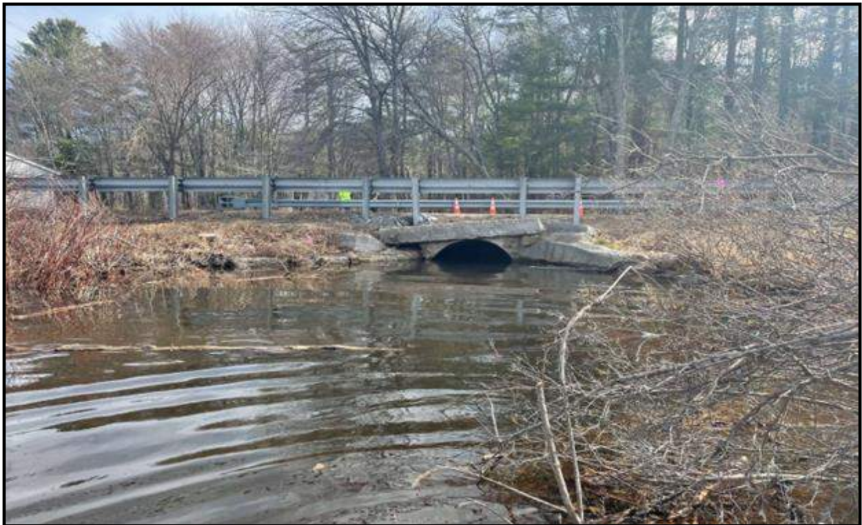
Photo 2: Culvert Outlet from Massabesic Lake (4/7/23) R. Thomson
