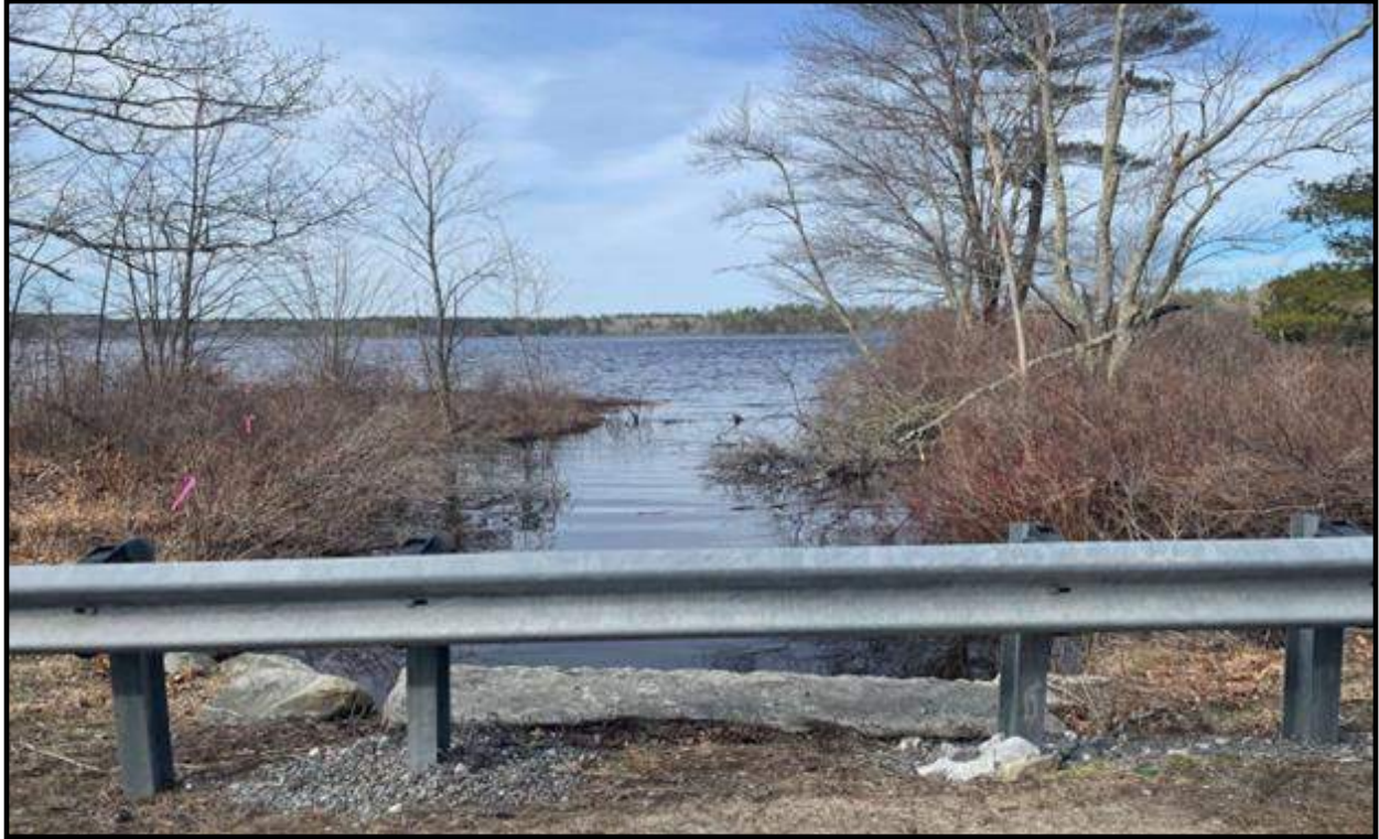
Photo 3: Looking towards Massabesic Lake from Culvert (4/7/23) R. Thomson
