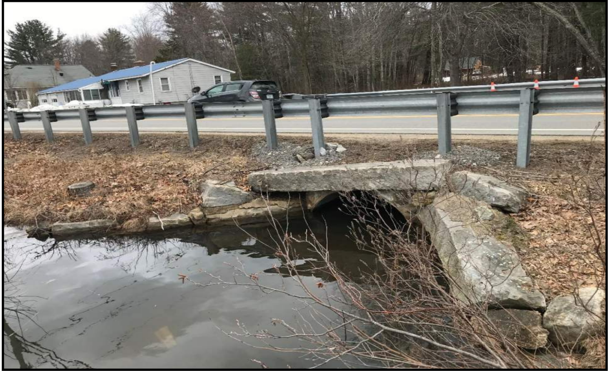
Photo 1: Culvert Outlet (3/24/23) J. Commerford
