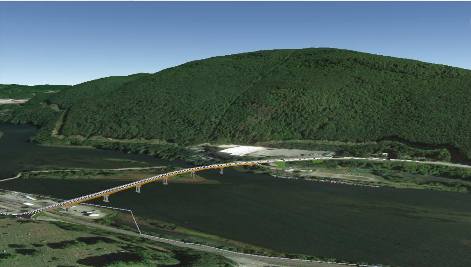
View From Southwest
