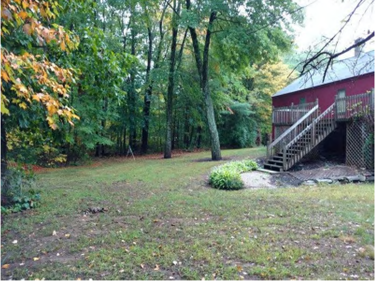
Location B: 52 Trolley Car Lane, Looking Southeast
