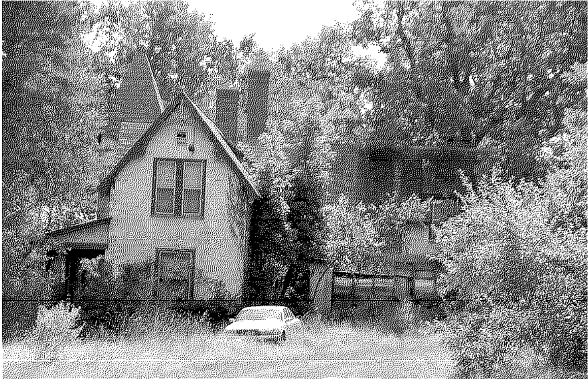
Photo 01: Rosencrans Pillsbury House, 22 Pillsbury Rd., abandoned and overgrown ( LON-WO , Woodmont Orchard Historic District)
