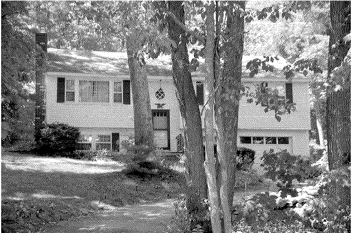
Photo D17: 64 Tsienneto Road, façade File Name: Derry2016_D17
