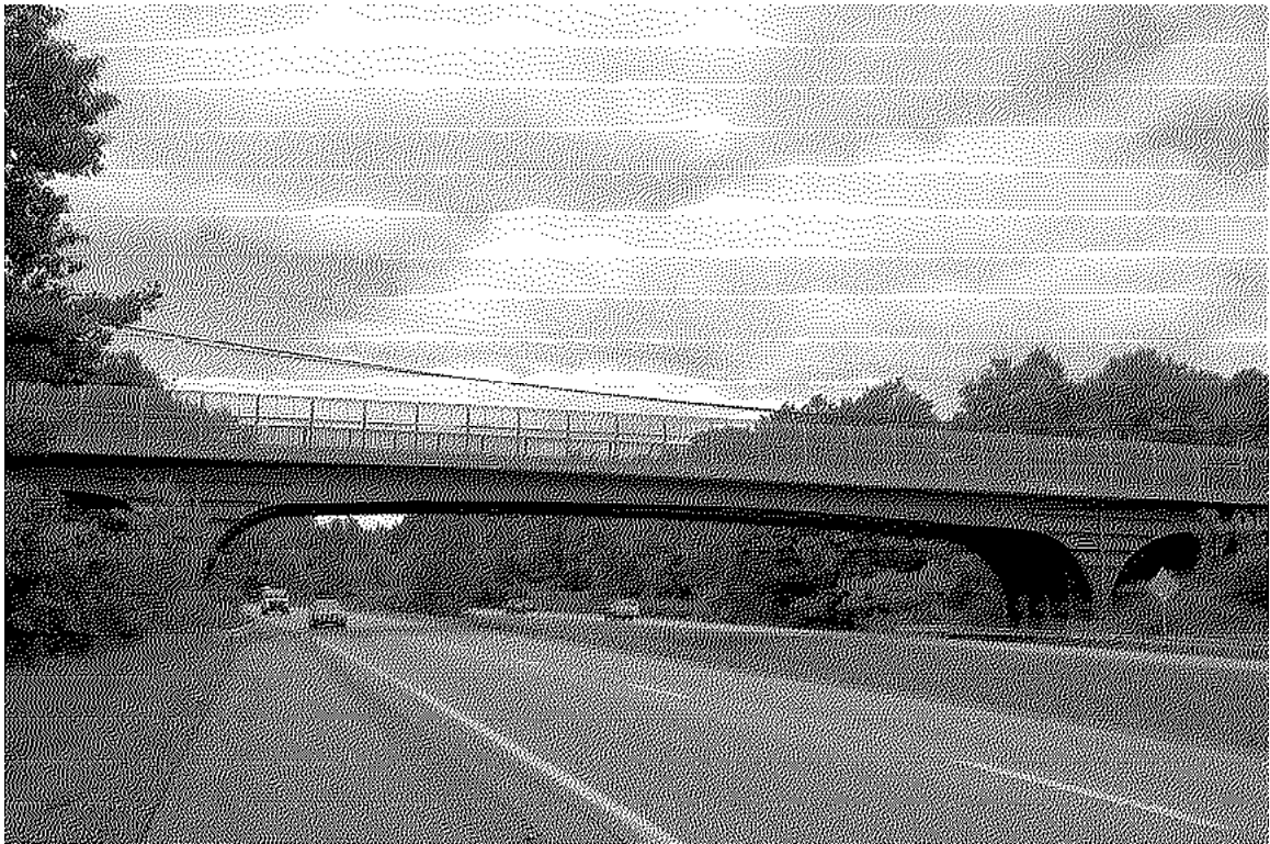
Photo 14: Ash Street Bridge (Robert J. Prowse Memorial Bridge) over Interstate 93 (LON0116)
