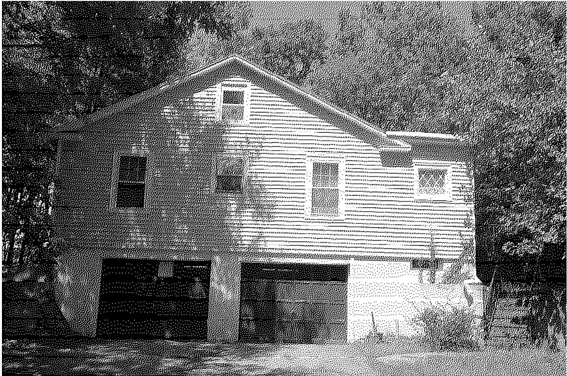
Photo D19: 83 Tsienneto Road, southwest elevation (façade not accessible)
