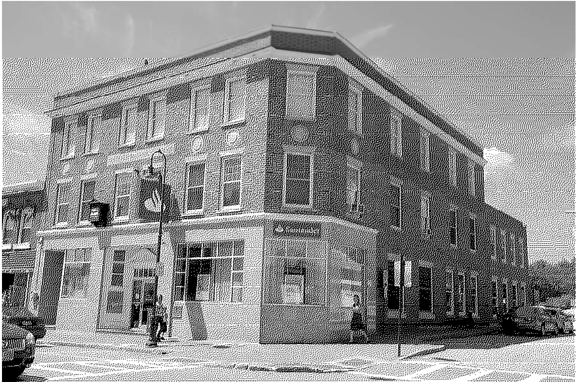
Photo U09: 20 East Broadway ( DER0062 ). Façade and east elevation of the First National Bank. No changes noted.
