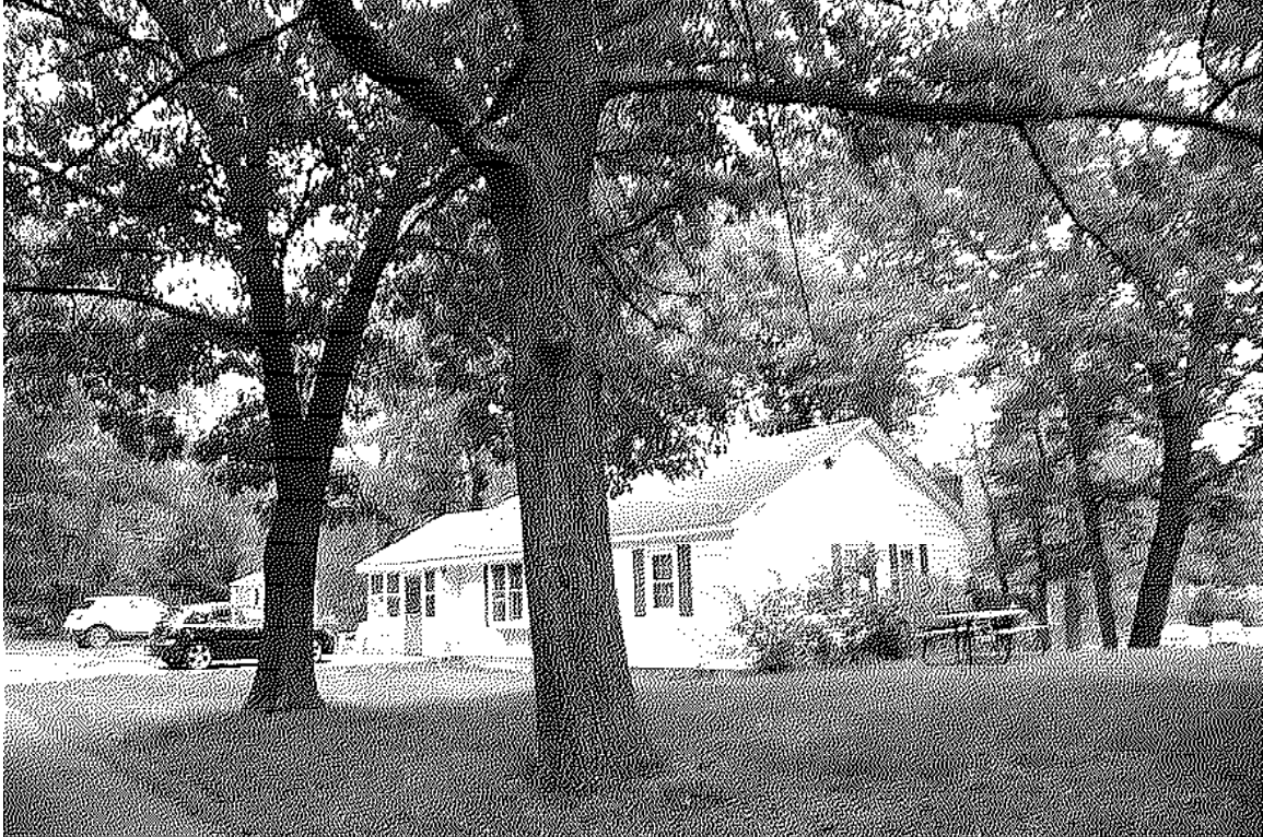
Photo 2) Façade and south elevation with street frontage; shed in background Reference (file name): Photo_June2018_176
