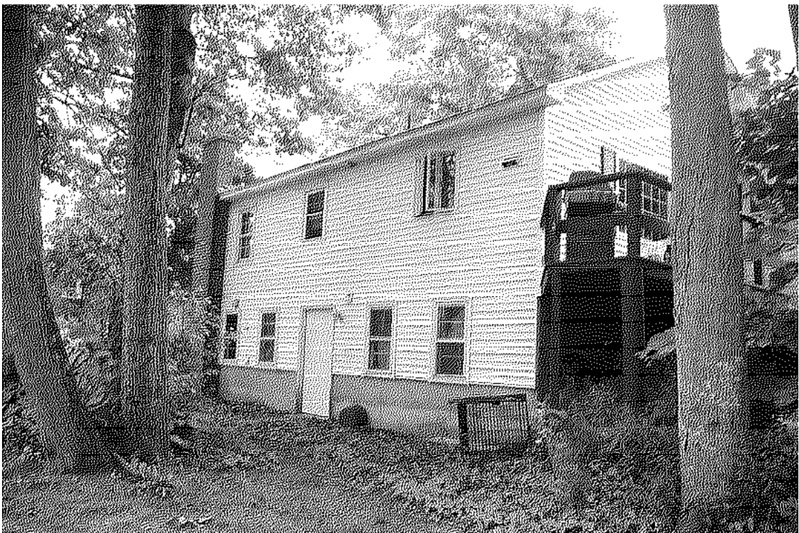
Photo 5) West (rear) elevation
