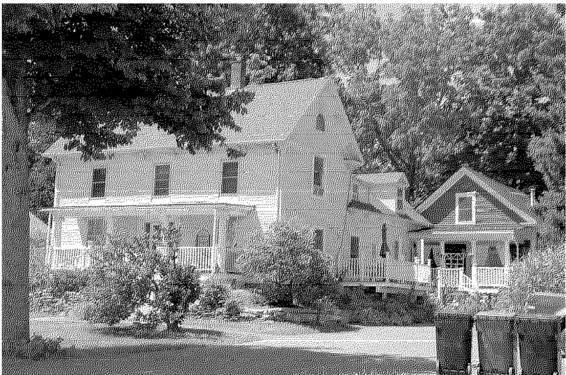
Photo U26: 126 East Broadway ( Area DV ). Façade and northeast elevation of the Wilson House. Vinyl siding and gutters added, vinyl replacement windows on upper floor. No other changes noted.
