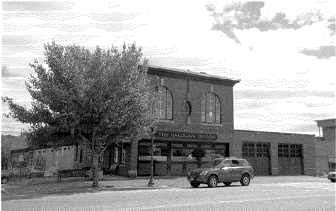
Photo U04: 32 West Broadway ( DER0047 ). Façade of the Central Fire Station. Building use changed to a restaurant, windows and garage doors have been replaced and/or infilled.
