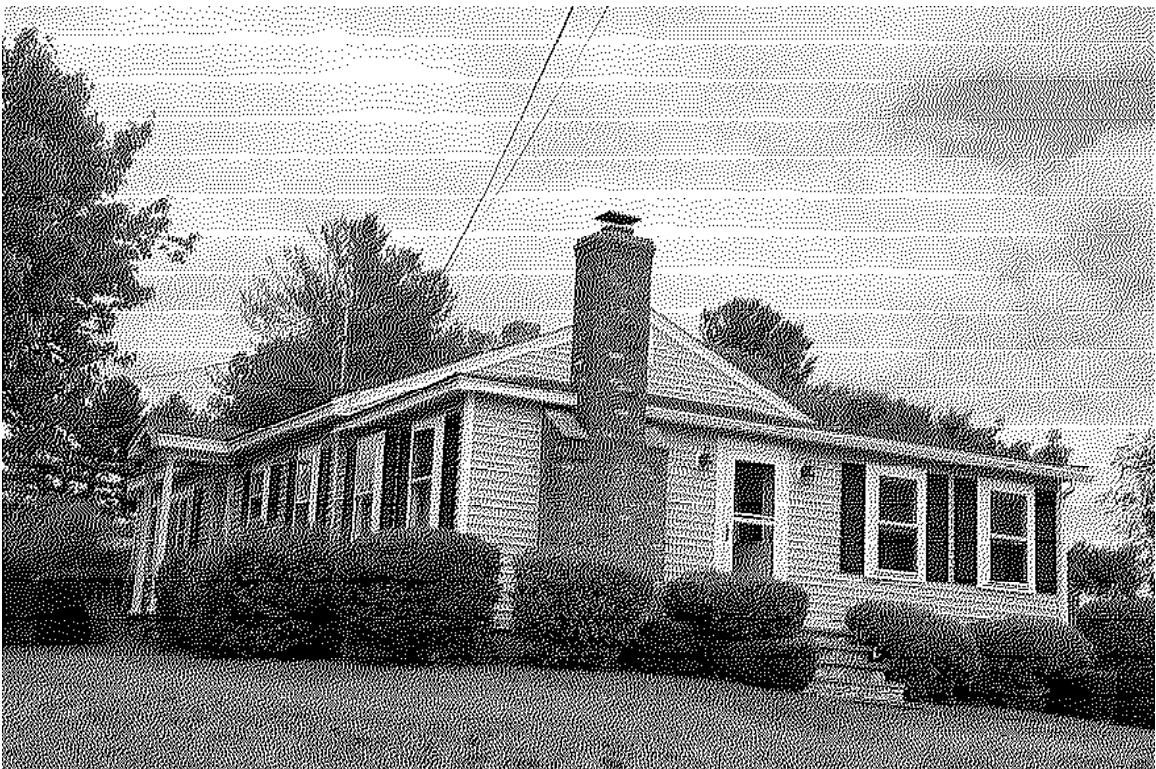
Photo D04: 9 Folsom Road, façade and southwest elevation.
