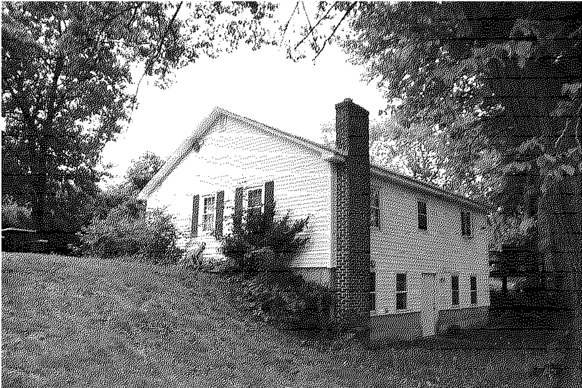
Photo 6) North and west elevation Reference (file name): Photo_June2018_181
