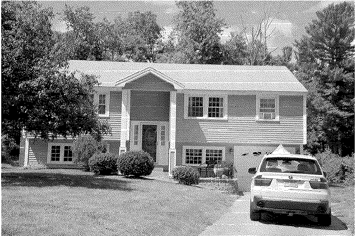
Photo D15: 1 Horseshoe Drive, façade File Name: Derry2016_D15
