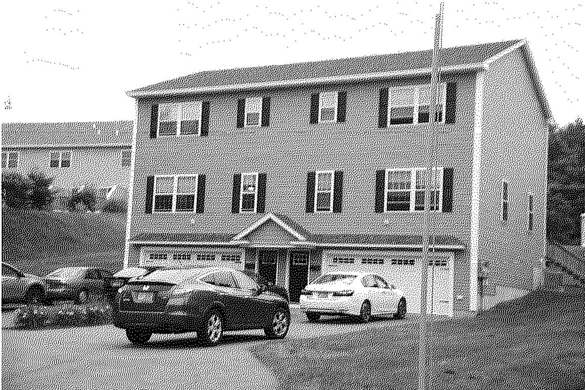
Photo 12) 5 Ferland Drive, façade Reference (file name): Photo_June2018_391
