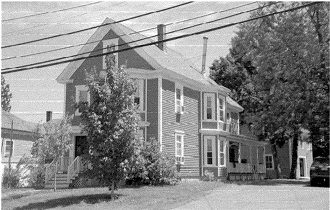
Photo U14: 69 East Broadway ( DER0083 ). Façade and west elevation the Wheeler House. Vinyl siding and replacement windows have been added, wood trim details and brackets have been removed, new front porch constructed.
