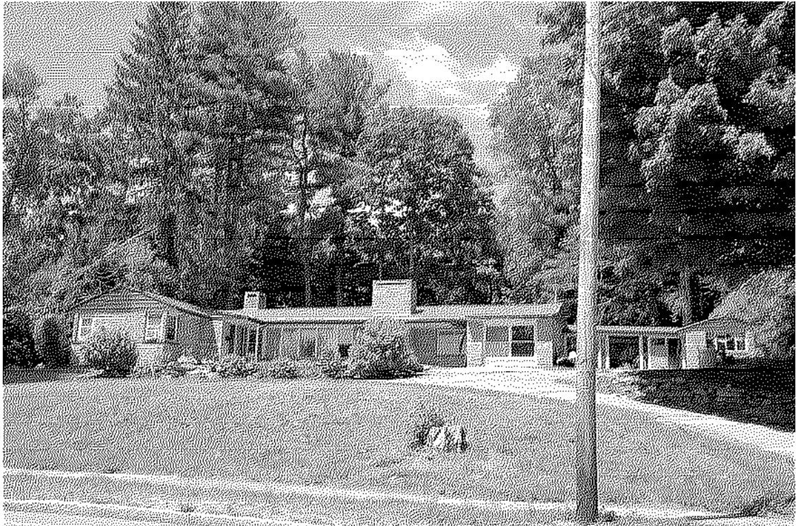
Photo U25: 104 East Broadway ( DER0141 ). Façade of the Amadee Cote House. Bay window has been replaced, no other changes noted.
