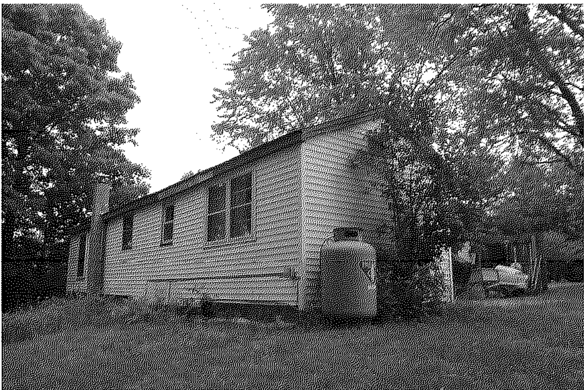
Photo 5) North (rear) and west elevations Reference (file name): Photo_June2018_169
