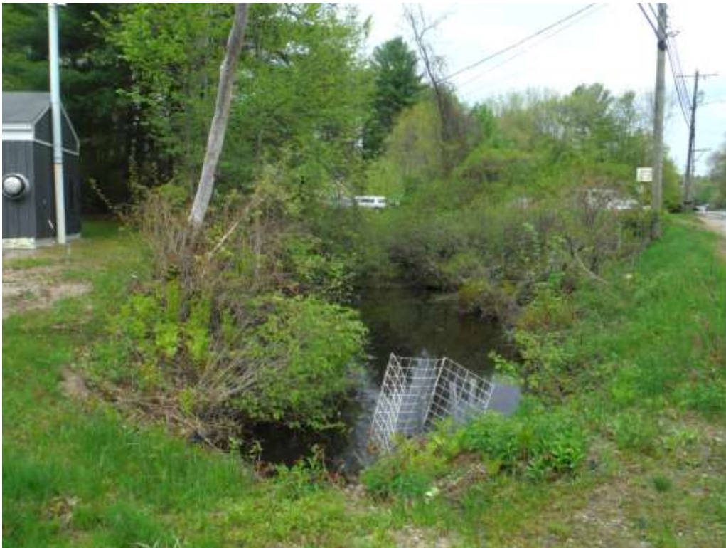
Photo 37. Facing northwest from Chester Road (NH Route 102) towards Stream Crossing 6 (5/15/2018)
