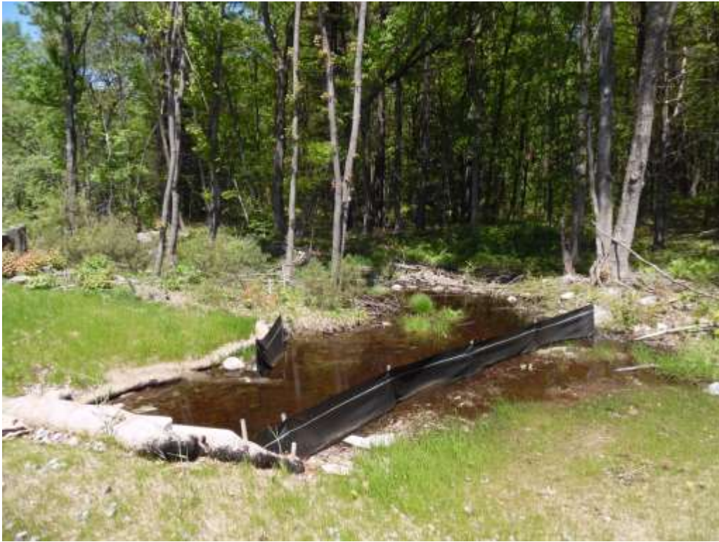
Photo 5. Facing north near southern end of Wetland 15 towards Vernal Pool 2 (5/21/2018). Erosion controls from recent construction for I-93.
