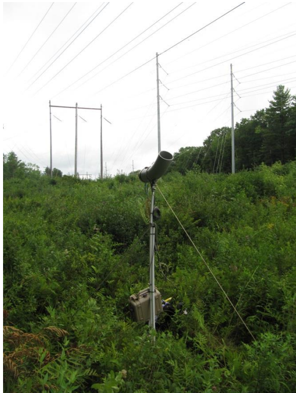
Figure C-24. Segment 4 – facing west.
