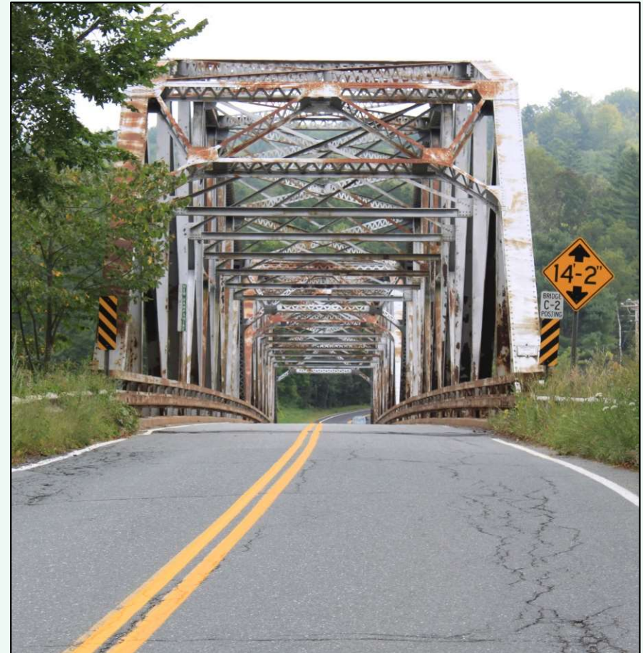
Vermont roadway approach
