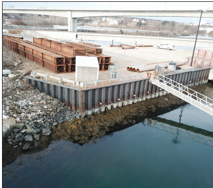
BARGE WHARF BULKHEAD LOOKING WEST (A1)
