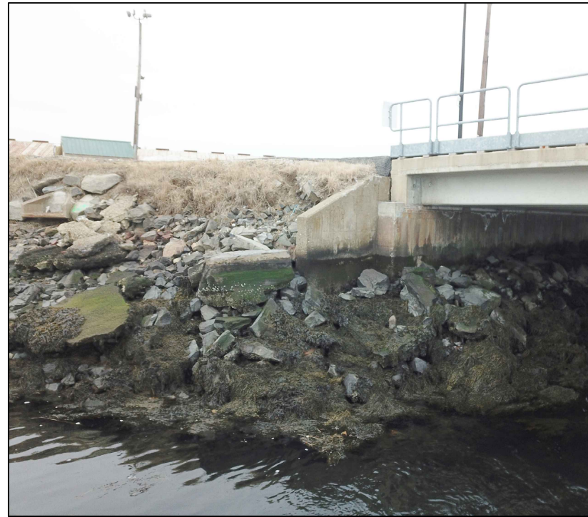
MAIN WHARF - BRIDGE ABUTMENT LOOKING WEST
