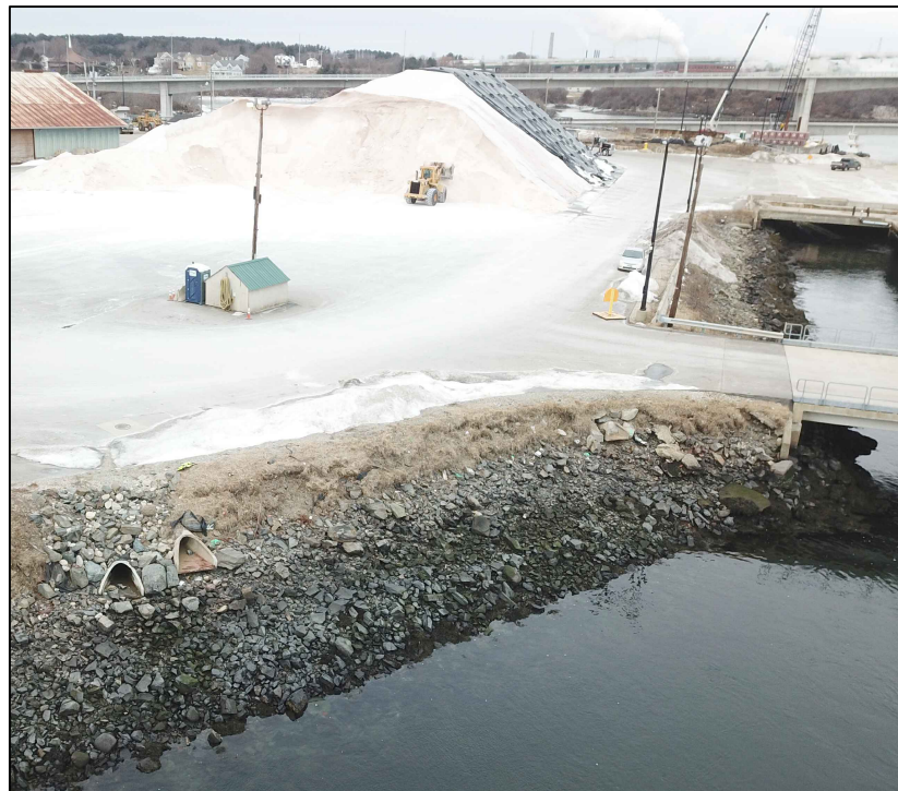
SOUTH WHARF EXTENSION REVETMENT LOOKING WEST
