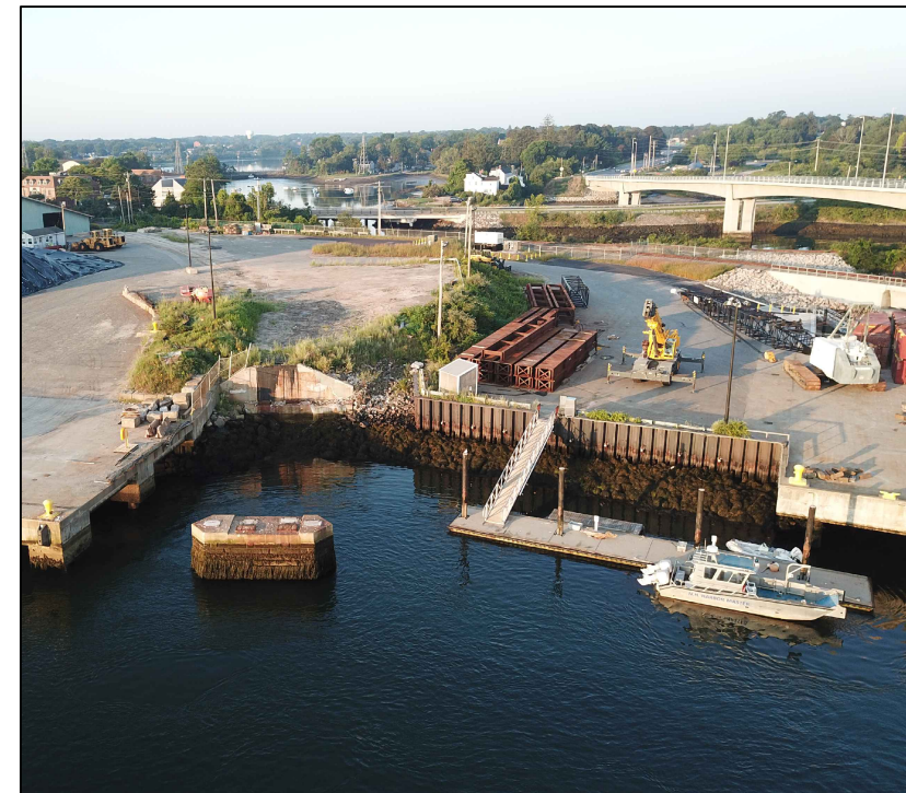
NORTH WHARF EXTENSION LOCATION LOOKING SOUTH
