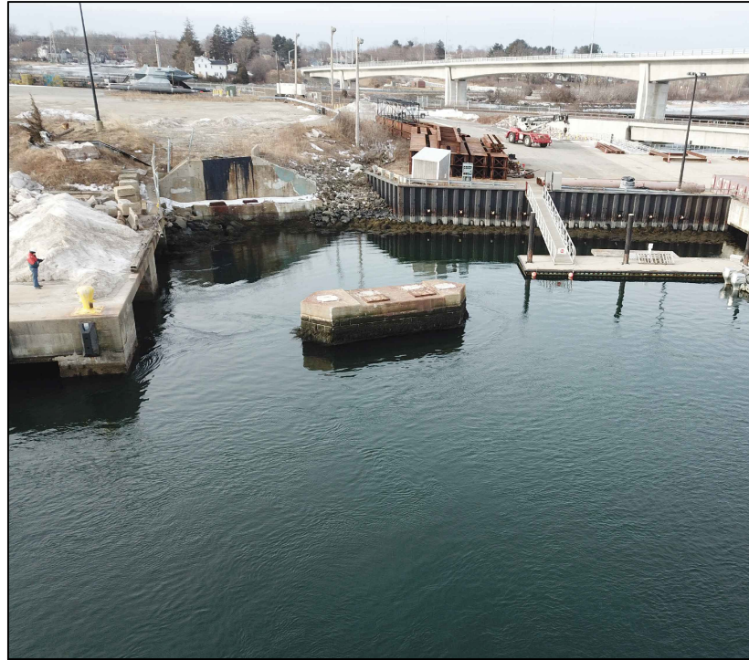
NORTH WHARF EXTENSION LOCATION LOOKING SOUTHWEST (C1)
