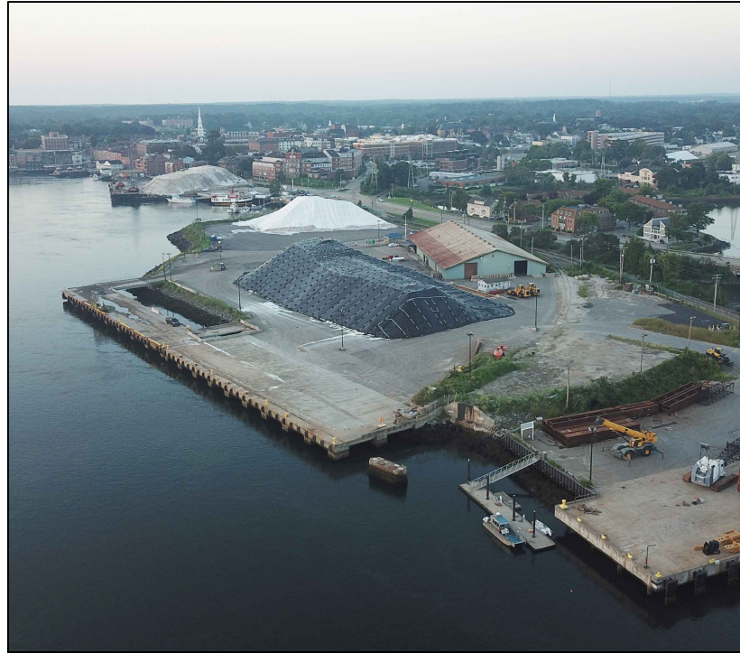
OVERALL SITE LOOKING SOUTH
