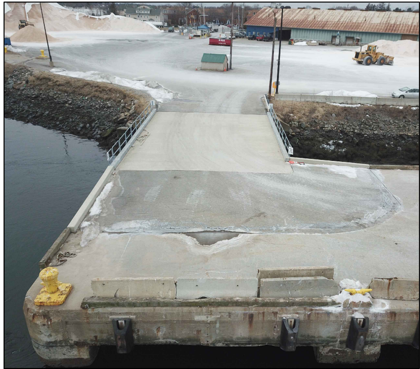
MAIN WHARF - SOUTH ACCESS BRIDGE LOOKING SOUTHWEST
