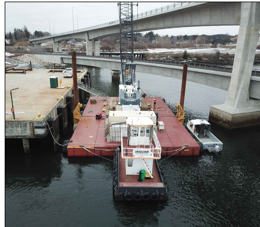
FLOATING DOCK - NEW LOCATION LOOKING SOUTHWEST (A4)
