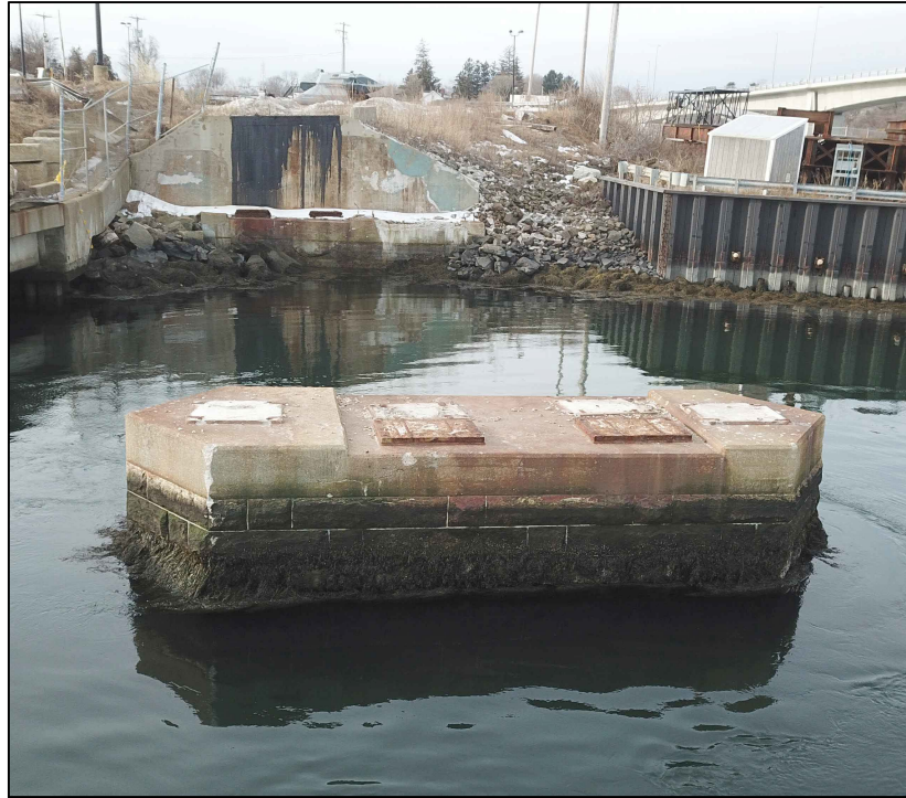
BRIDGE PIER 14 LOOKING SOUTHWEST (C3)
