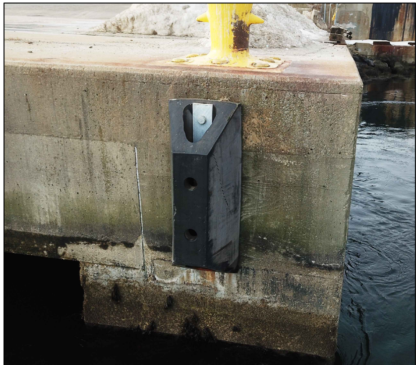
MAIN WHARF - FENDER SYSTEM LOOKING SOUTHWEST
