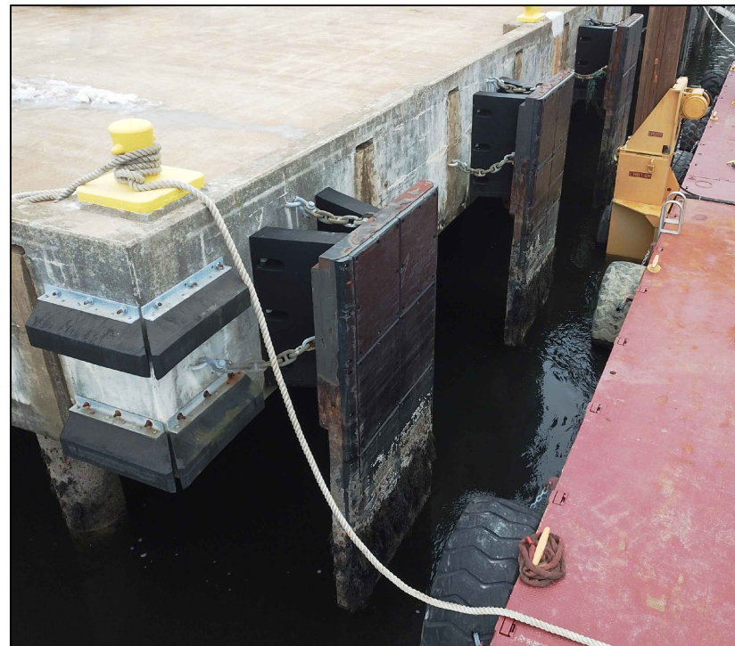
BARGE WHARF - FENDER SYSTEM LOOKING SOUTH
