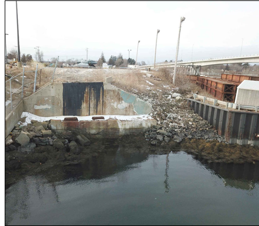
BRIDGE ABUTMENT 13 LOOKING SOUTHWEST (C4)
