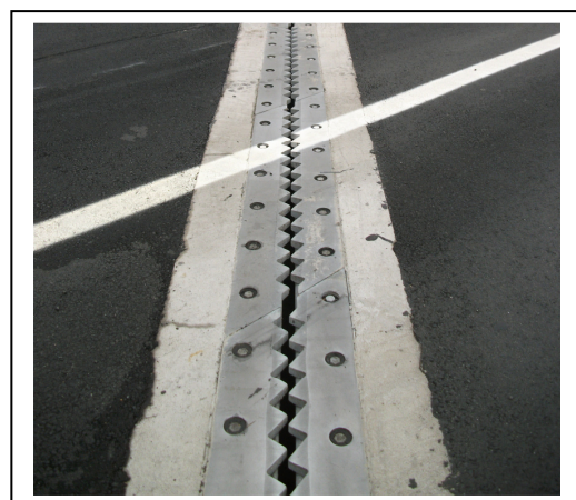
Strip Seal Expansion Joint with Plow Plate
