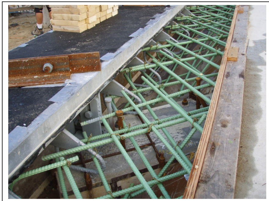
Finger Expansion Joint Reinforcing
