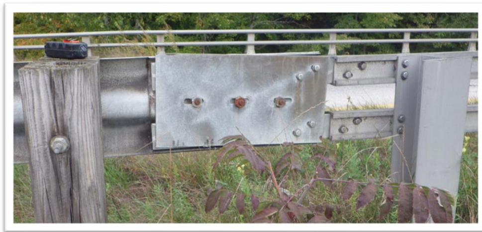
Aluminum Bridge Back-up Plate
