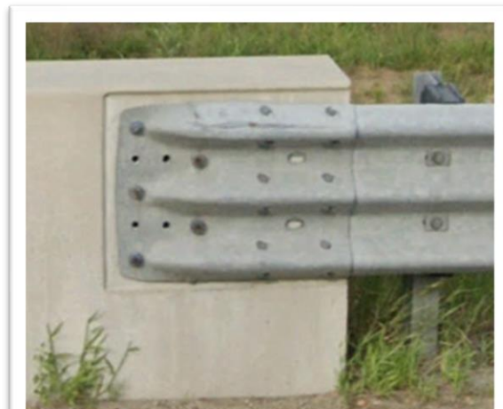
Connection Plate and Thrie-Beam Terminal Connector
