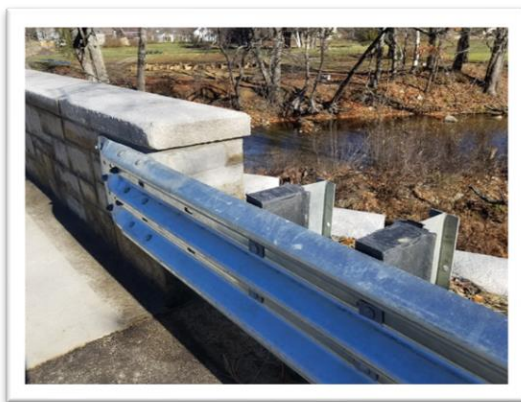
Connection Plate and Thrie-Beam Terminal Connector
