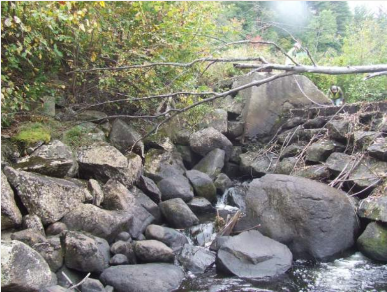
Southern Bridge Abutment
