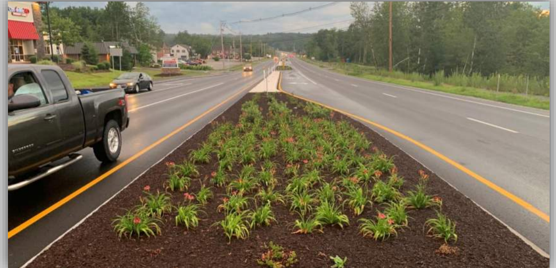
Landscaped Median NH Route 101 - Bedford
