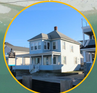
PROPERTIES ON HAVERHILL, BRADFORD, AND ATLANTIC AVENUES
