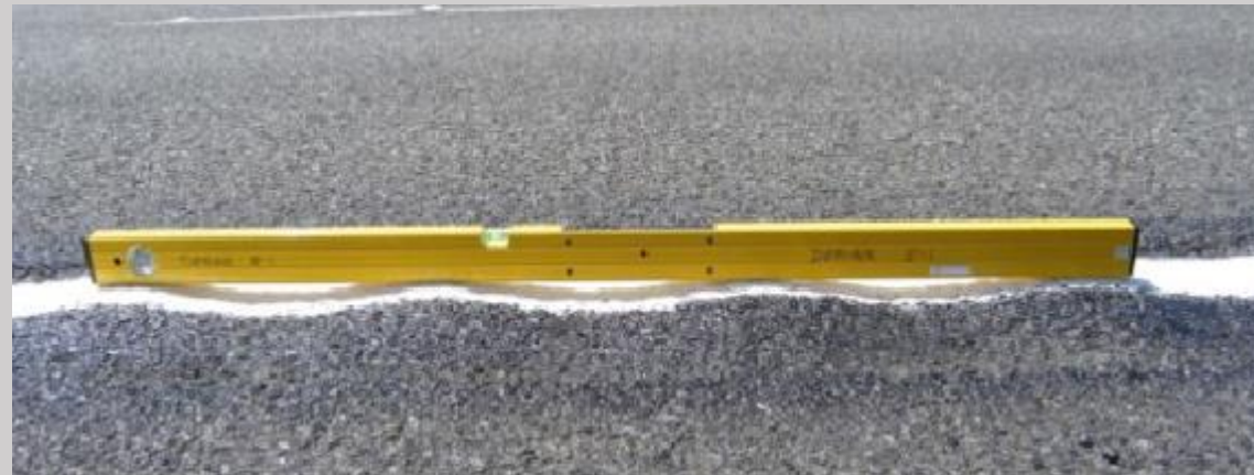
Figure 2. Sinusoidal Rumble Strip - Longitudinal Section
