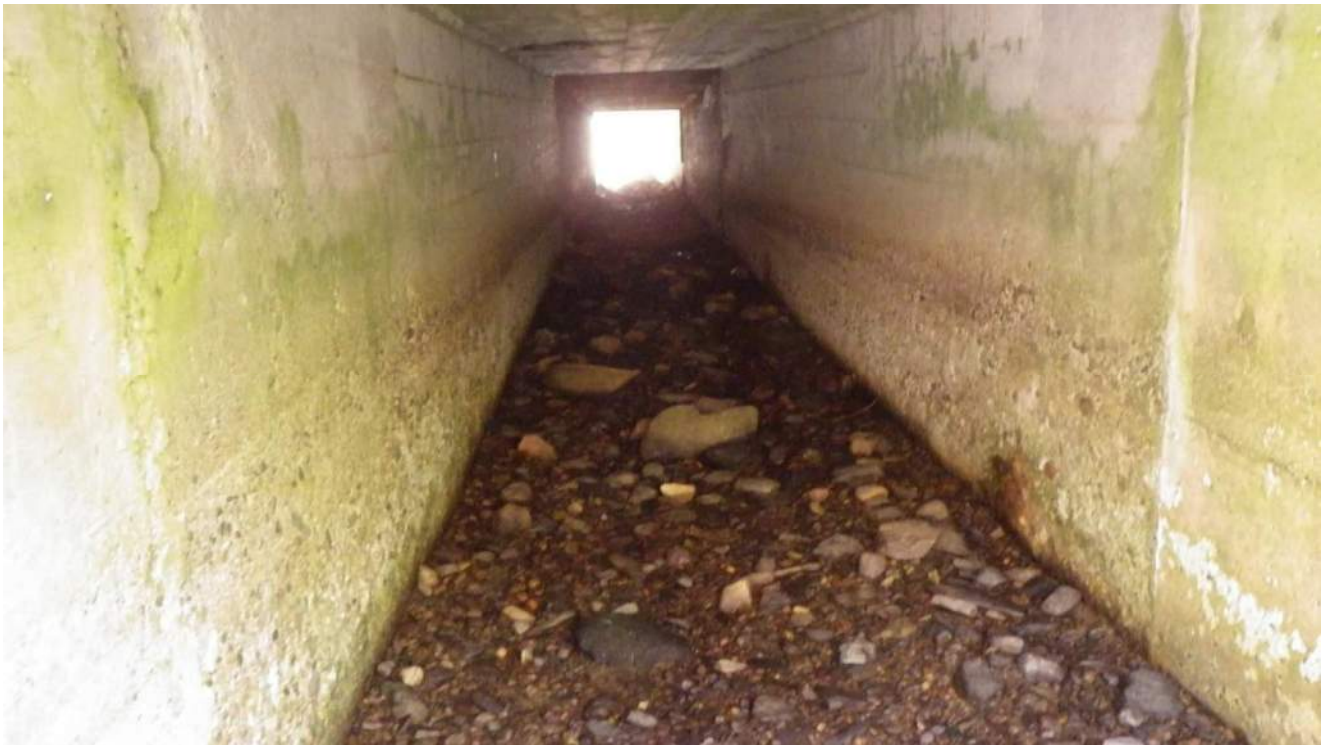
Outlet side (newer construction) Proposed simulated bed material is similar to existing bed material inside culvert
