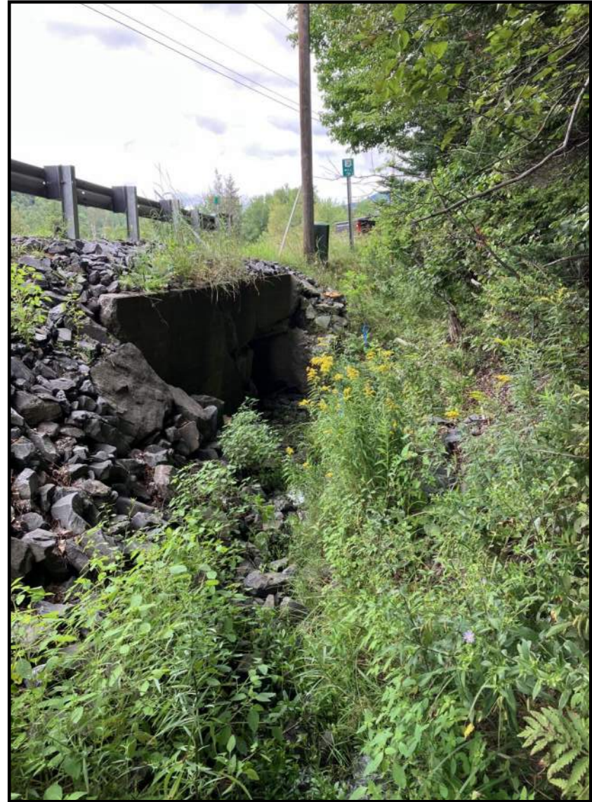
Photo 2: Looking downstream at inlet at hard armoring on banks.
