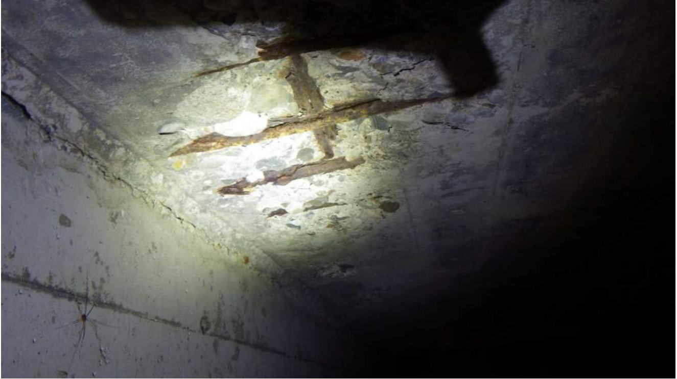
Severe spall in culvert roof, rebar exposed
