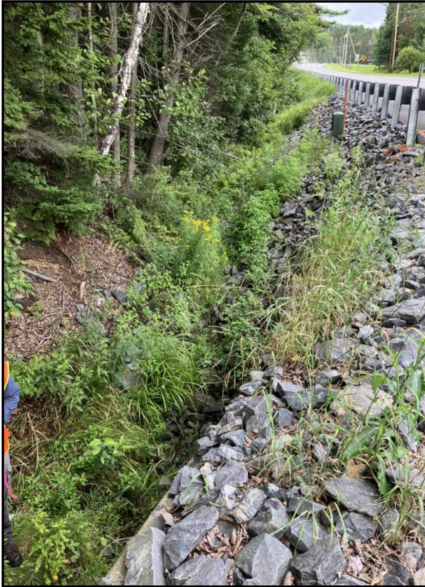
Photo 1: Looking upstream from Inlet at hard armoring on banks.
