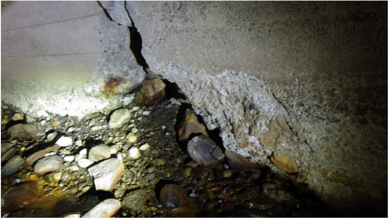
Wall joint between older and newer construction Cracking / spalling with void behind, backfill material leaking
