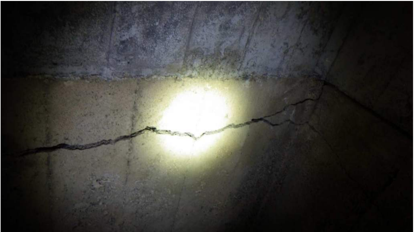
Structural crack in culvert roof
