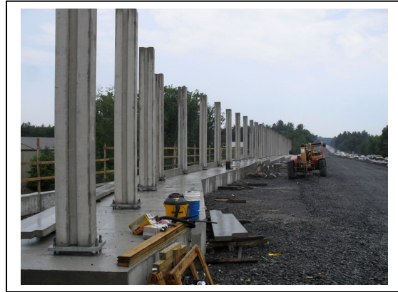
NHDOT Soundwall on a Moment Slab
