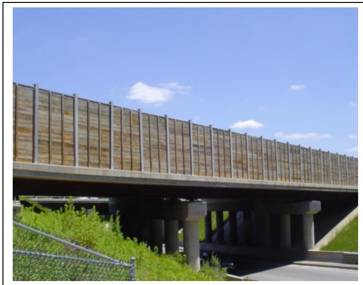
NHDOT Timber Soundwall on a Bridge (No longer used.)
