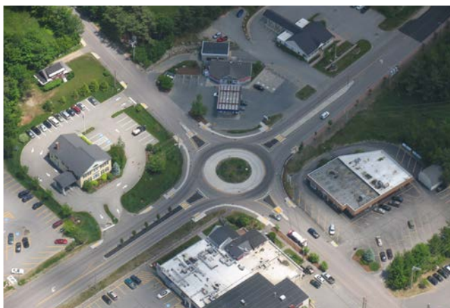
Newport/County Road Intersection Improvements, New London, NH (LPA/CMAQ Funded)
