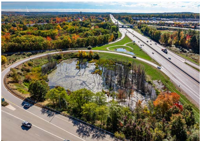
The widening of the F.E. Everett Turnpike Nashua-Merrimack-Bedford 13761/13761D project was successfully completed on time and within budget by the CHA proposed team members: Rob Faulkner, Ellen Moshier, John Parrelli, Charlie Symmes, Rebecca Howe, Matthew Kowalski, and Sam Molner.
