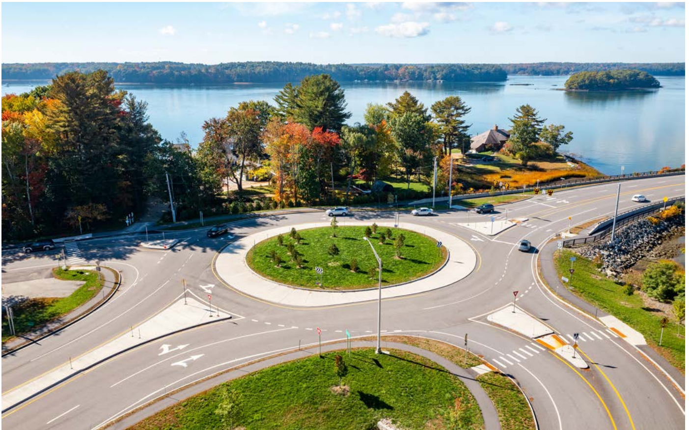
U.S. Route 4/Spur Road/Boston Harbor Road Roundabout (Newington-Dover 11238).
