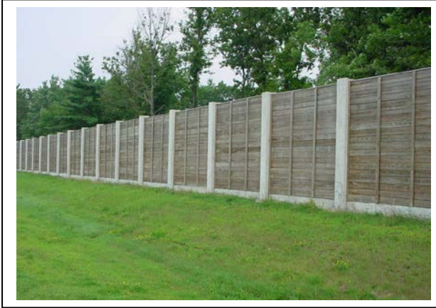
NHDOT Soundwall on a Precast Leveling Panel
