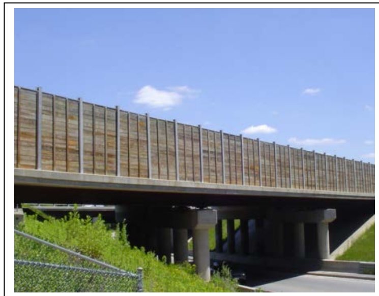
NHDOT Soundwall on a Bridge
