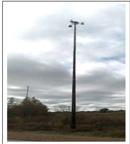
Typical NHDOT High-mast Light Poles
