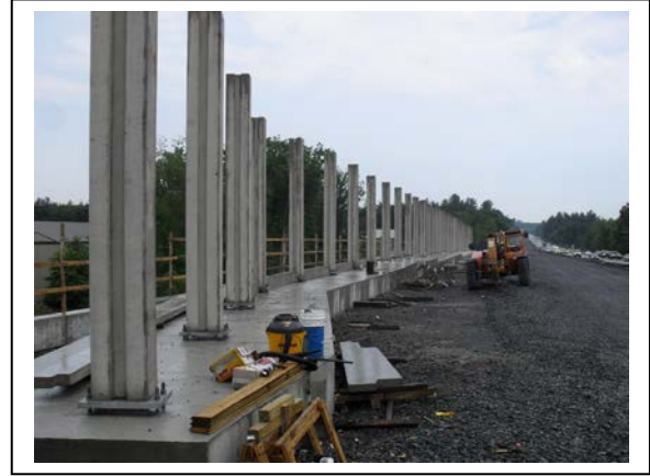
NHDOT Soundwall on a Moment Slab
