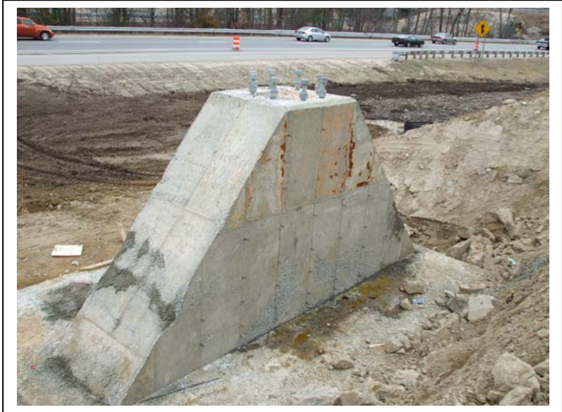
Typical NHDOT Sign Structure Footing
