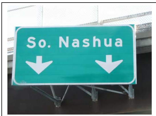
Typical NHDOT Bridge Mounted Sign Supports
