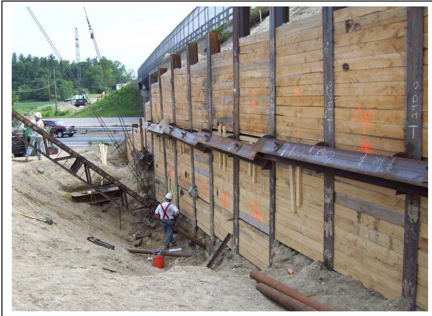
(Soldier Pile with Timber Lagging)
