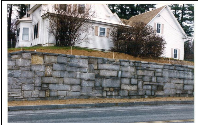
BARTLETT (Sheet Pile Wall with Stone Facing)
