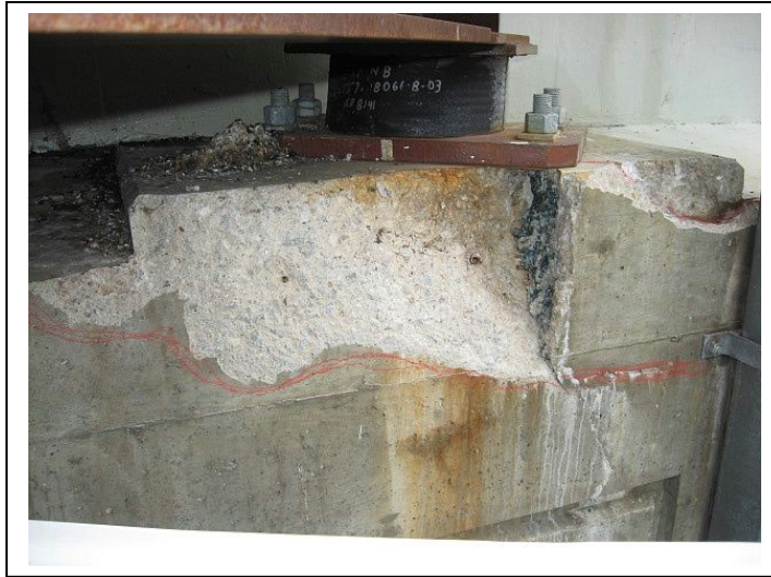
Pedestal Failure
