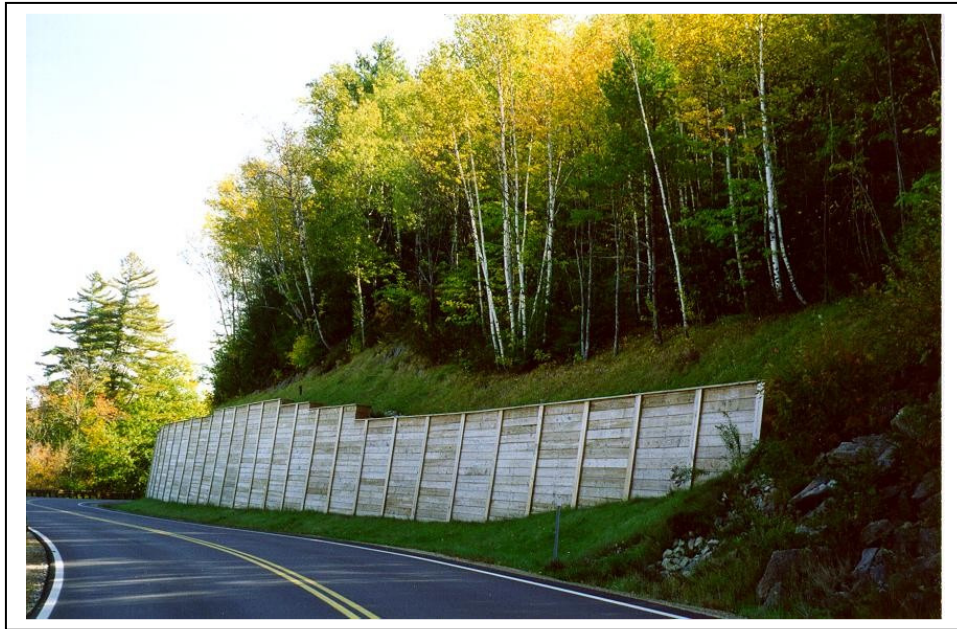
ALBANY (Soil Nail Wall with Timber Facing)
