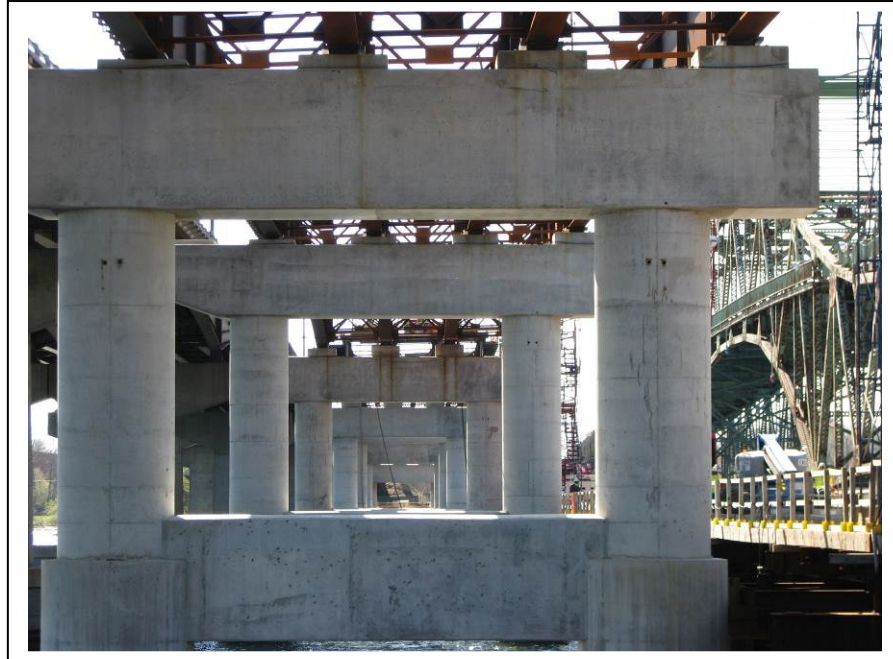
(Phase 1 construction, three-column pier when completed)
