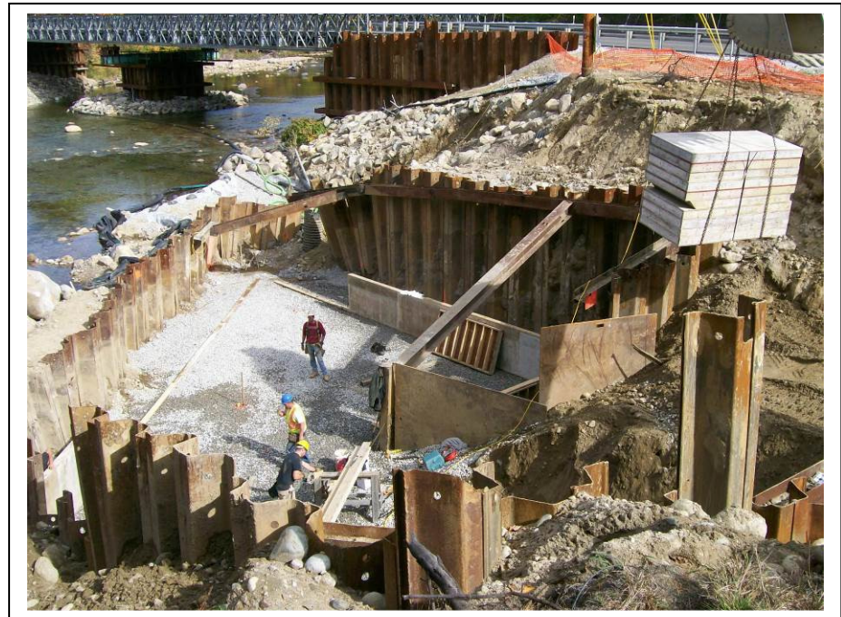
(Steel Sheetting - Cofferdams)
