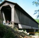
Covered Bridge, constructed in 1906, is a 124-ft-long, single-span truss. Principles of the Secretary of the Interior's Standards for Rehabilitation and the Burlington Charter were applied to all phases of the work. This project included a Section 106 historical clearance.
