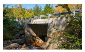
the deteriorated concrete deck span with a new precast concrete voided slab deck, new bridge and approach rails, and minor repairs to the concrete abutments.
