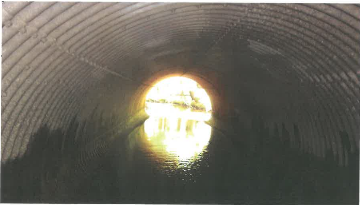
Looking Downstream through Structure
