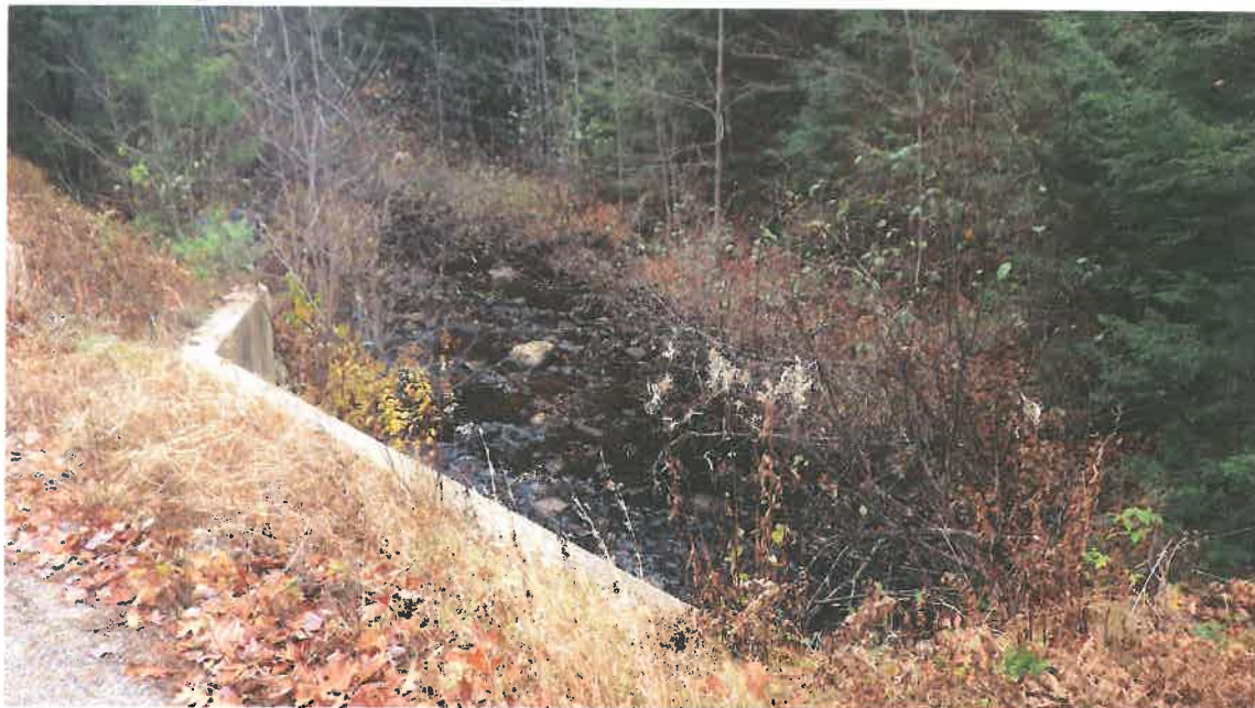
Upstream Channel – Facing Upstream from Above the Inlet
