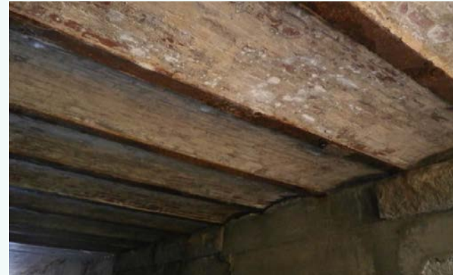
Underside of 1898 jack arch bridge (NHDOT)
