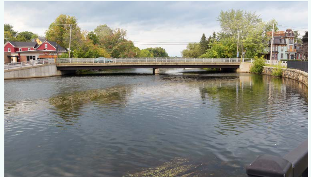
The modern Church Street Bridge built in 1981 is an I-beam bridge with a concrete deck (Preservation Company)
