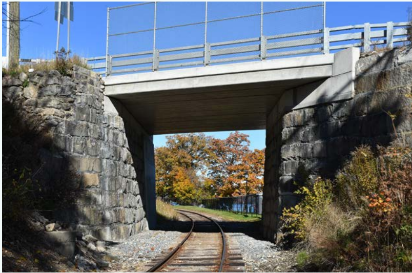
2021 view facing northwest, with original stone abutments still visible (Preservation Company)
