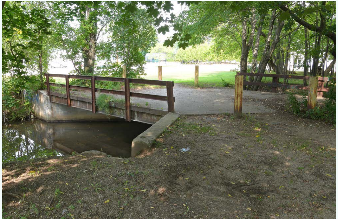
I-beam stringer bridge, 2021 (Preservation Company)
