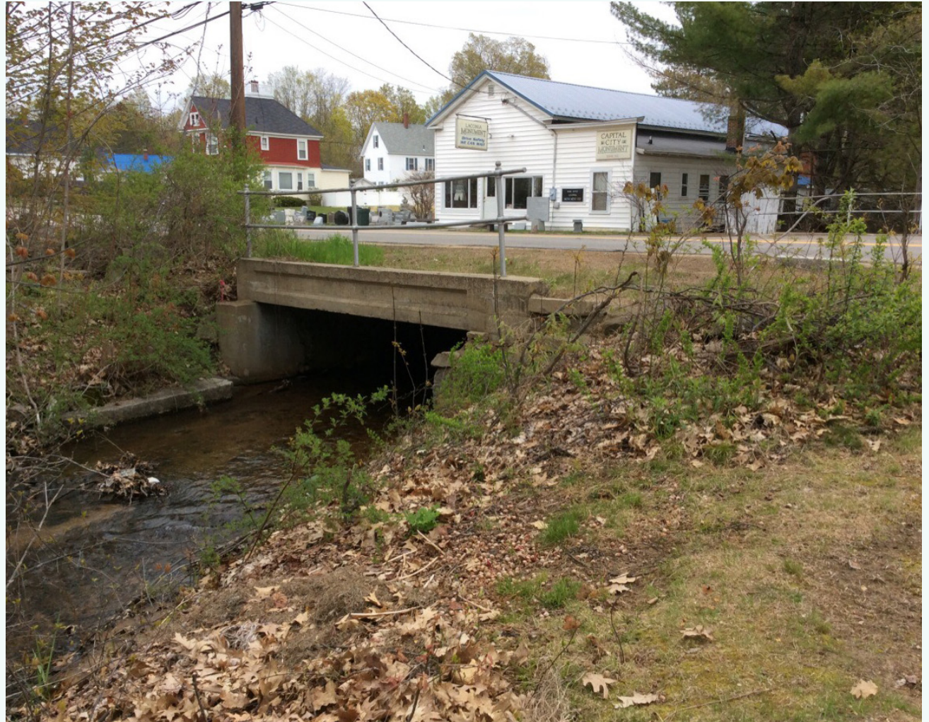
Academy Street Bridge, 2019 (NHDOT)
