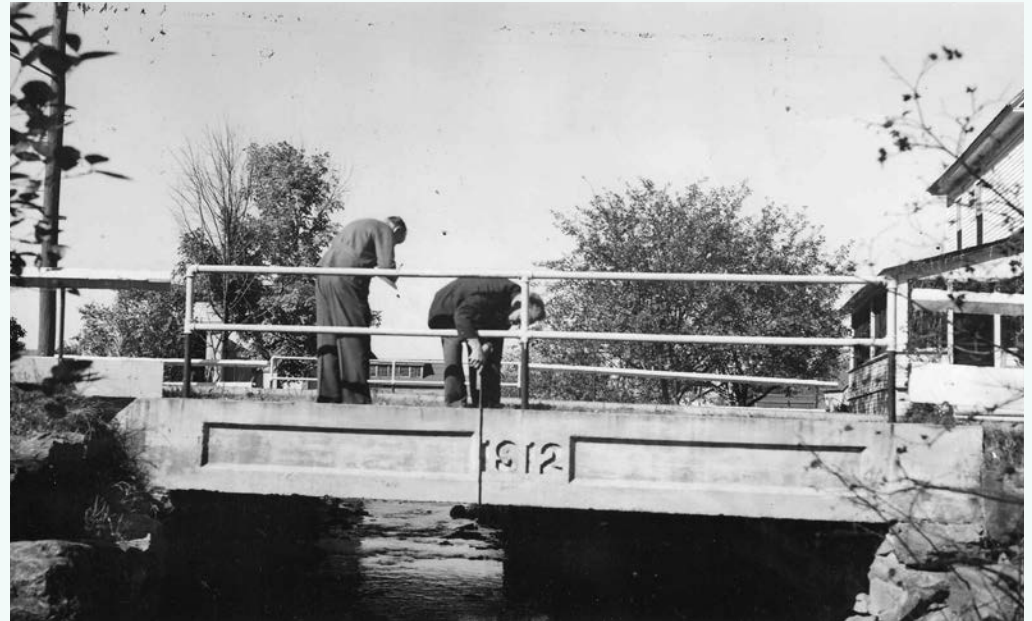
Court Street Bridge in 1940 (NHDOT)
