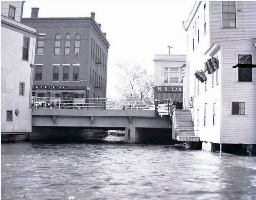
Old Main Street Bridge in Downtown Laconia in the 1930s or 1940s, showing buildings later demolished for Urban Renewal (Huse 2017, courtesy of Dean Dexter)
