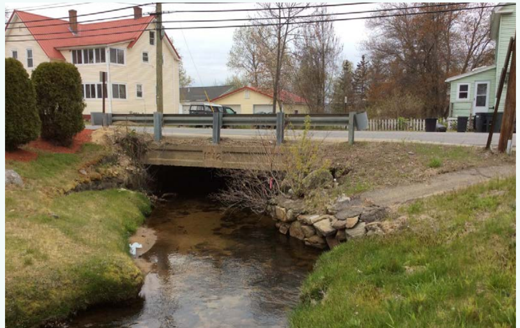
Court Street Bridge in 2019 (NHDOT)
