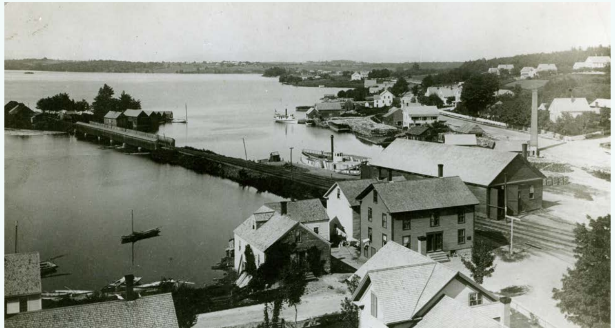
1880s view facing northeast, showing the earlier Lakeport railroad bridge with a wooden boxed pony truss bridge over the water (Laconia Public Library)
