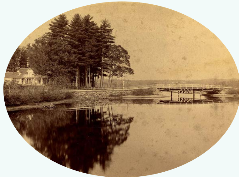
The Messer Street Bridge built ca. 1880 was an open deck type of suspension bridge supported by truss rods below the deck (Laconia Historical and Museum Society)
