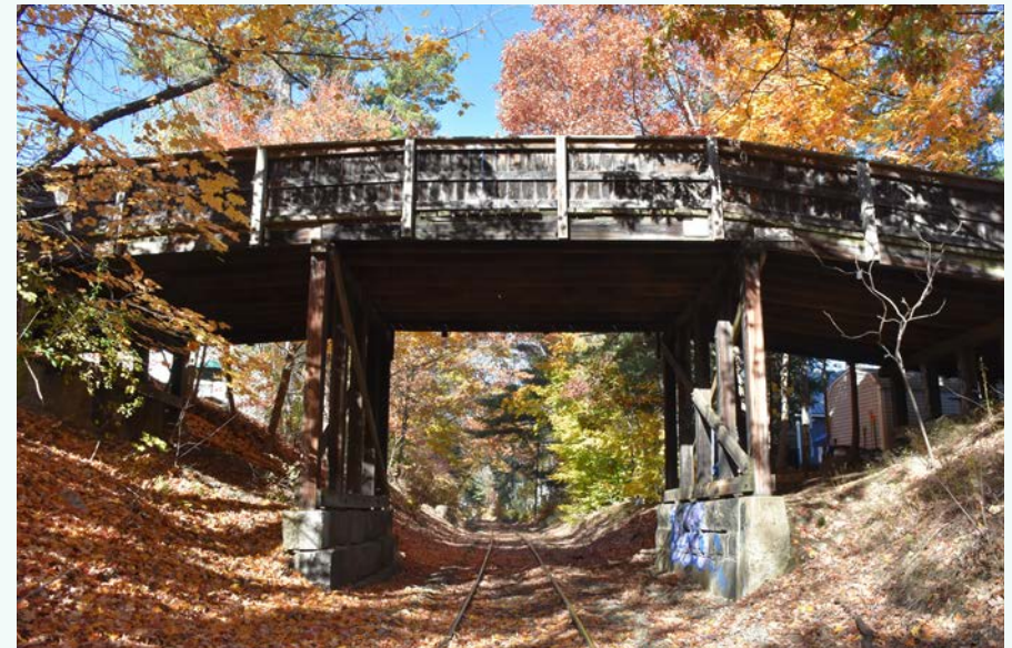
Centenary Avenue Bridge, facing north, 2021 (Preservation Company)
