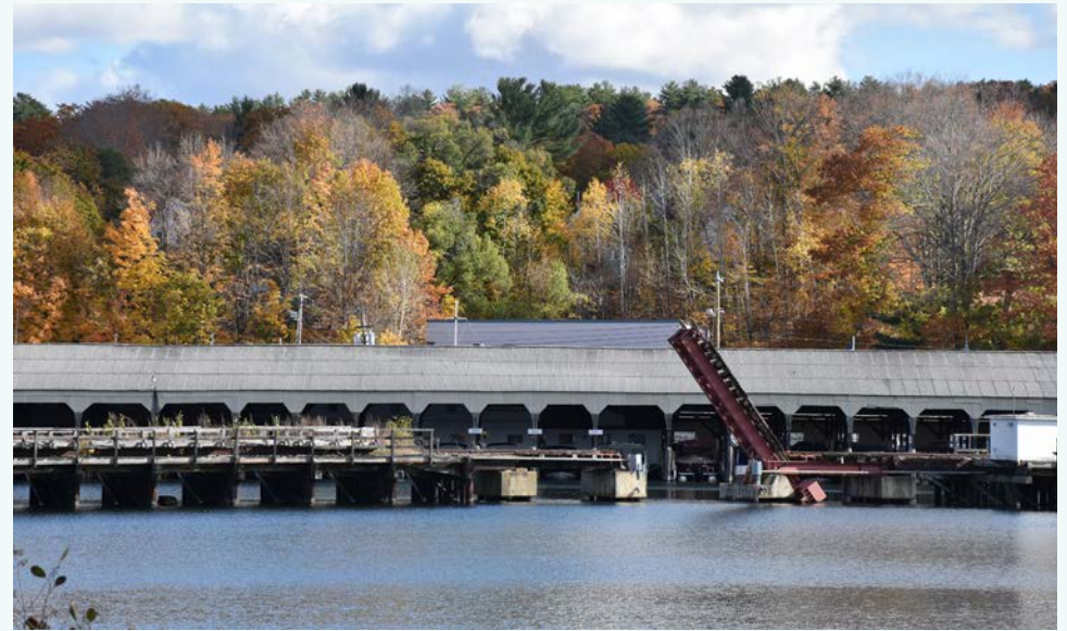
Lakeport Drawbridge, facing southeast, 2021 (Preservation Company)
