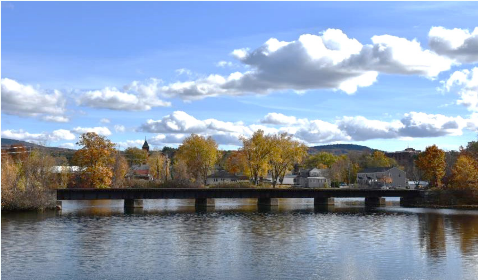
View of railroad bridge from Messer Street Bridge, 2021 (Preservation Company)
