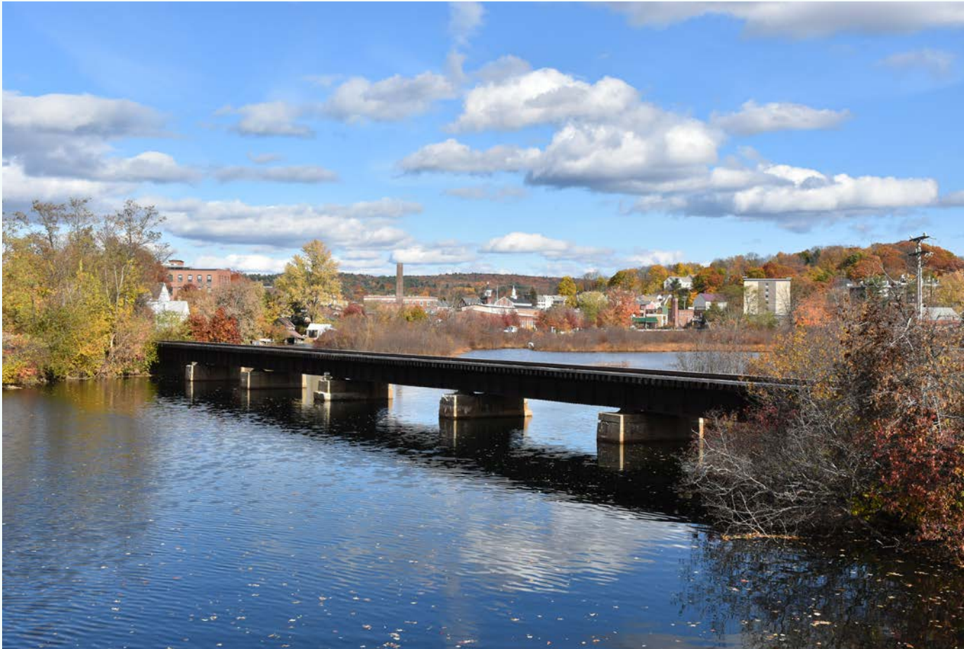
View of railroad bridge from Fair Street Bridge, 2021 (Preservation Company)
