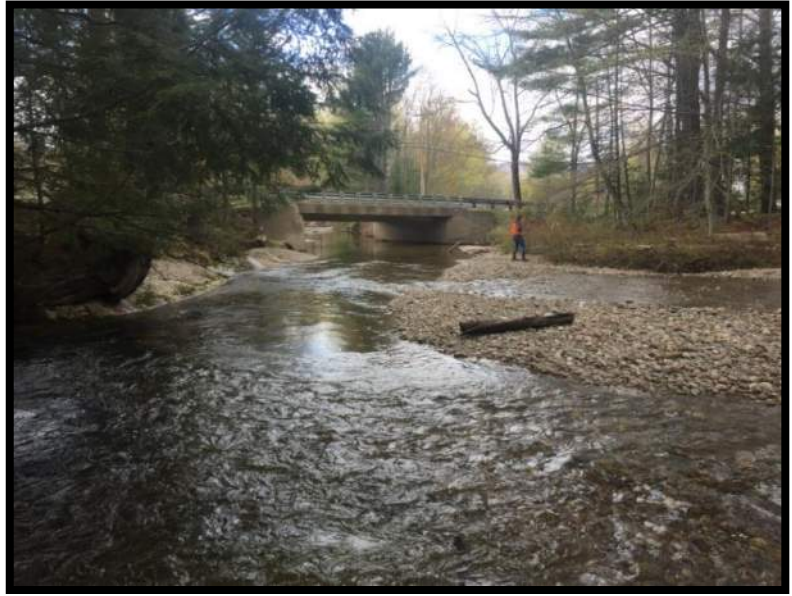
This is a view looking downstream towards the crossing structure.
