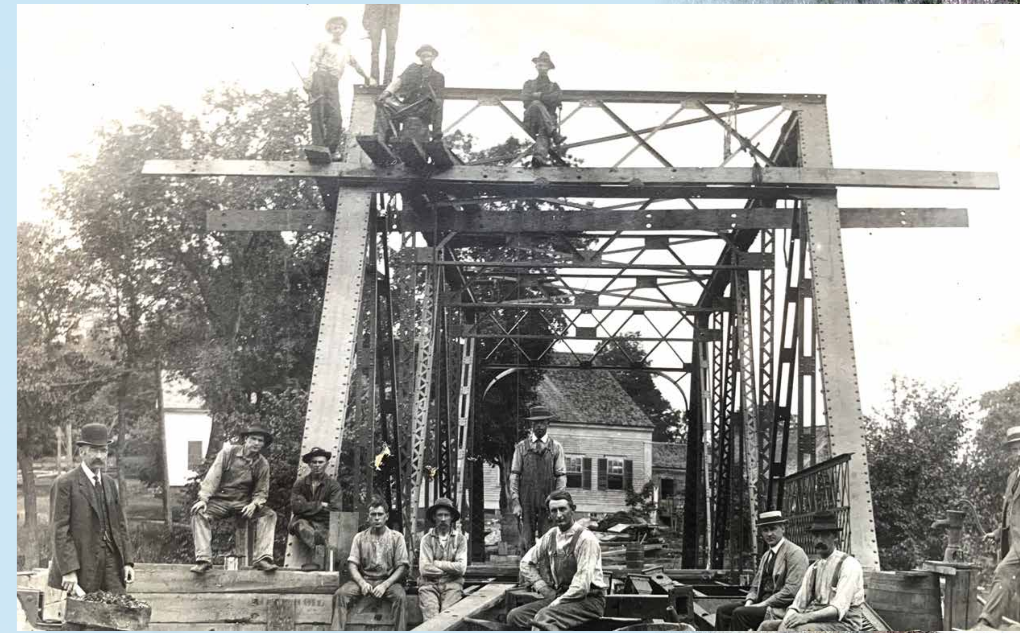
The men constructing the new steel bridge taking a moment to pose for this photo. Courtesy of Wentworth Historical Society
