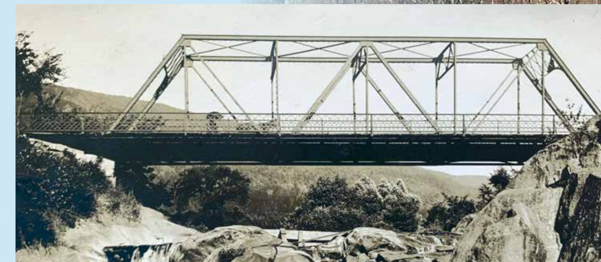
Look closely and you will see that there's a horse and buggy crossing the steel bridge, a Warren thru-truss built in 1909. Courtesy of Wentworth Historical Society
